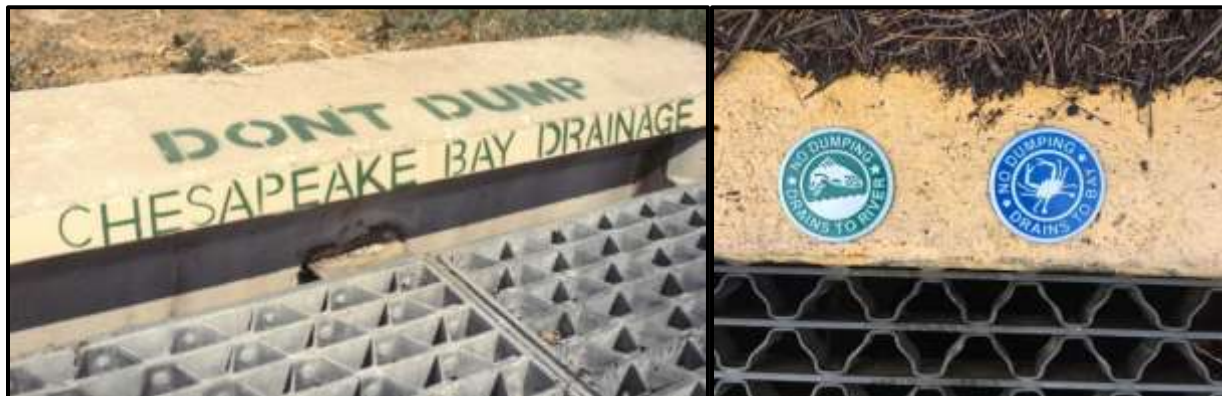
Figure 7. Storm drain stencil (left) and medallion (right) used by Anne Arundel County.
