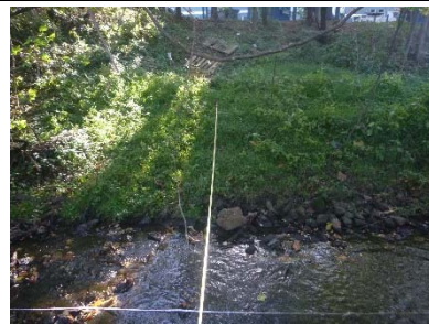
Right Bank View
