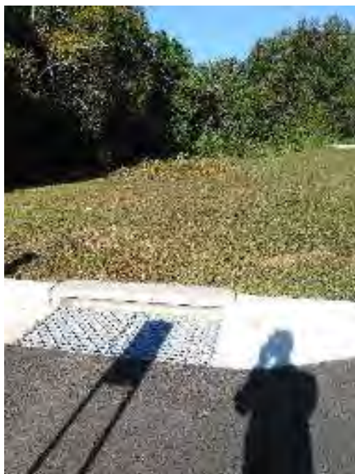
Figure 5: Unidentified stormwater structure and storm drain inlet.
