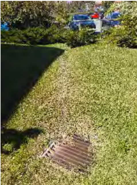
Figure 3: Stormdrain in grass area north of building.
