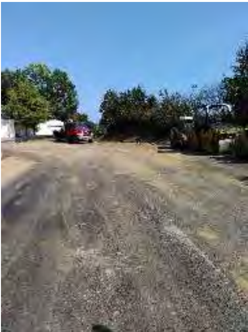
Figure 5: fresh pavement in rear of property.
