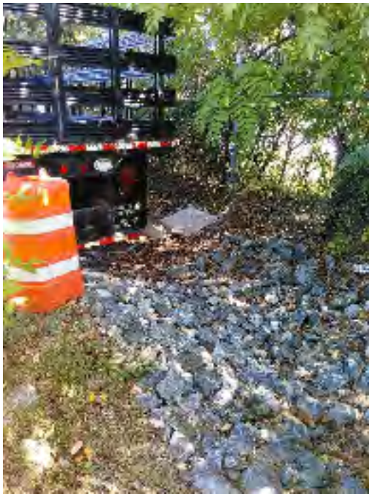
Figure 2: Rip rap lined drainage channel draining east parking lot along I-97.
