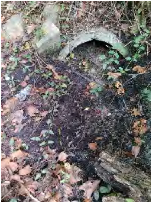
Figure 3: Blocked Outfall
