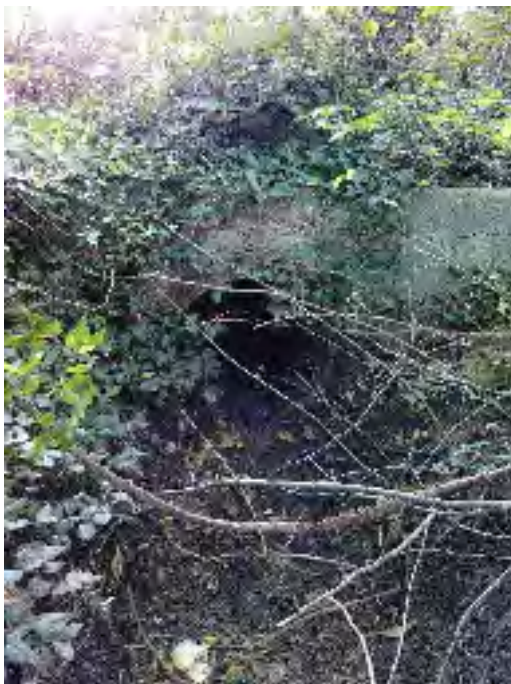
Figure 5: Stormwater outfall at the Northern District Police Station (Brooklyn, MD)
