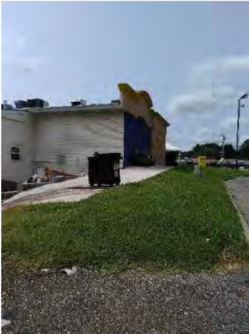
Figure 2: La Trampita Restaurant's grease storage container with visual evidence of leaking grease on the ground to the left of the container.
