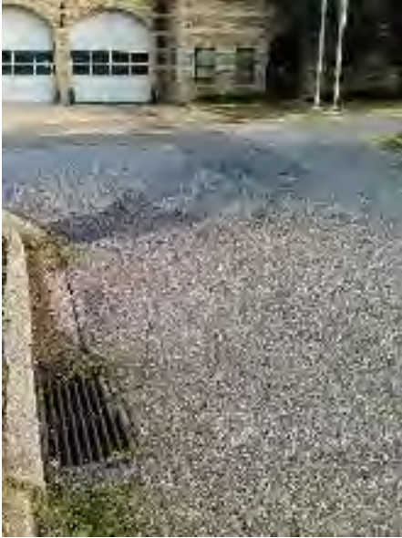
Figure 2: Possible wash water drainage into the stormdrain inlet.
