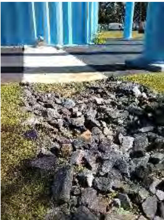
Figure 4: Water tower spillway.
