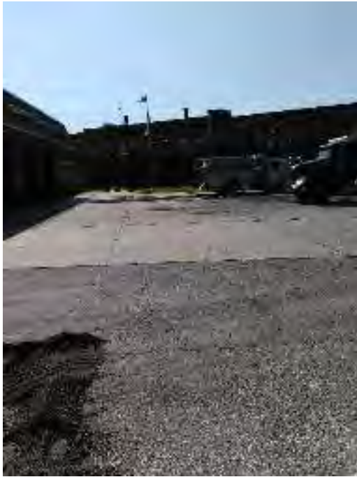
Figure 2: Front driveway pad undergoing construction.
