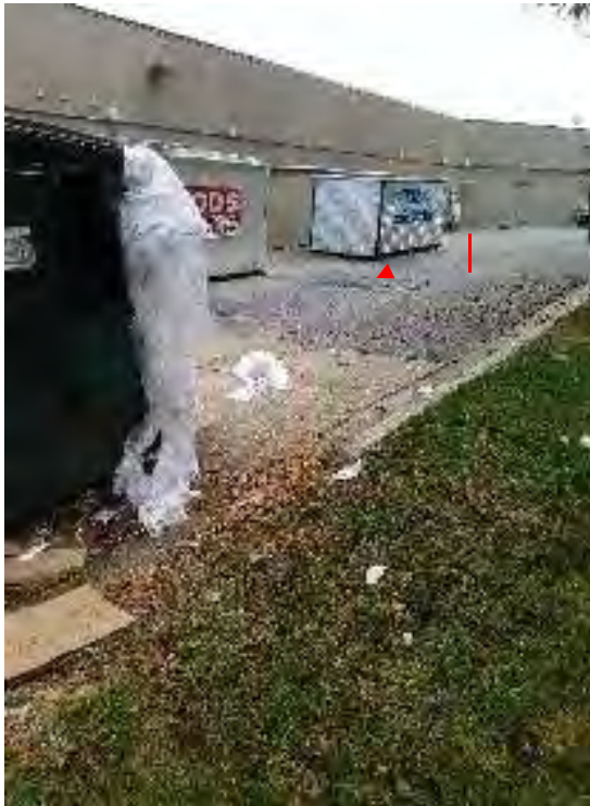
Figure 3: Dumpster location relative to inlet indicated by red arrow.
