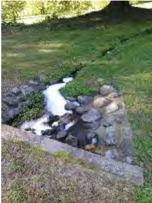
Figure 6: Outfall discharge area during first test and washing activity.
