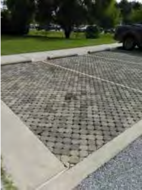
Figure 2: Permeable pavement
