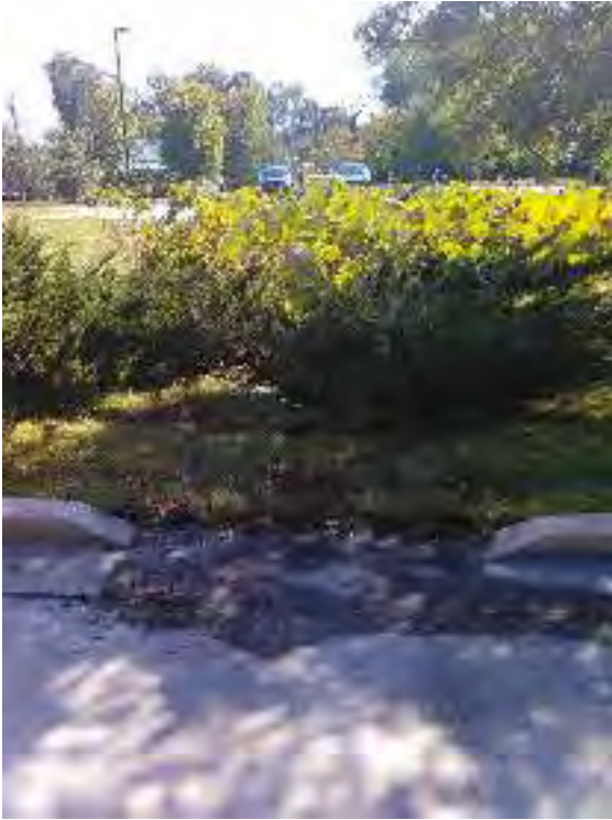
Figure 2: curb cut draining rear driveway pad. Drains to western pond.
