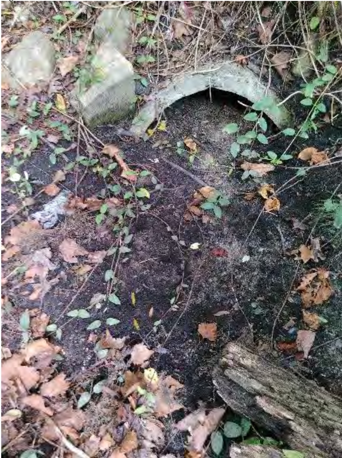
Figure 2: Sedimentation of Outfall Q050007
