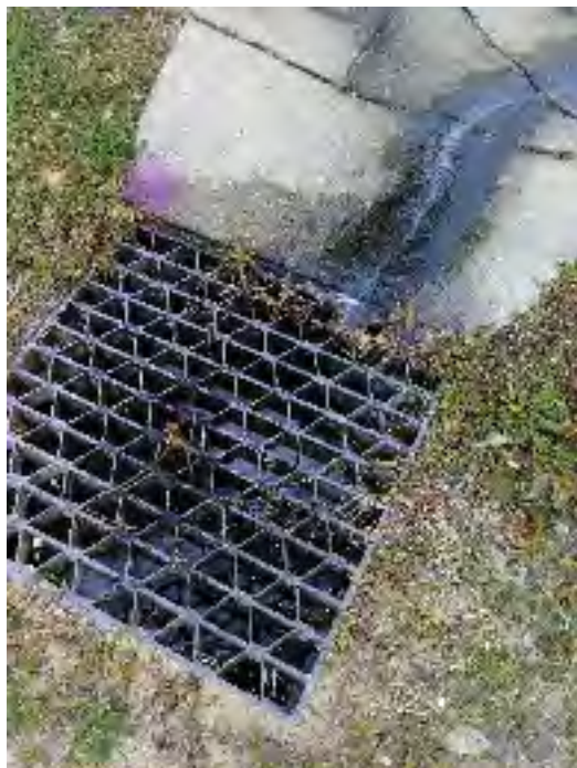
Figure 3: Stormdrain inlet accepting wash water runoff during first test.
