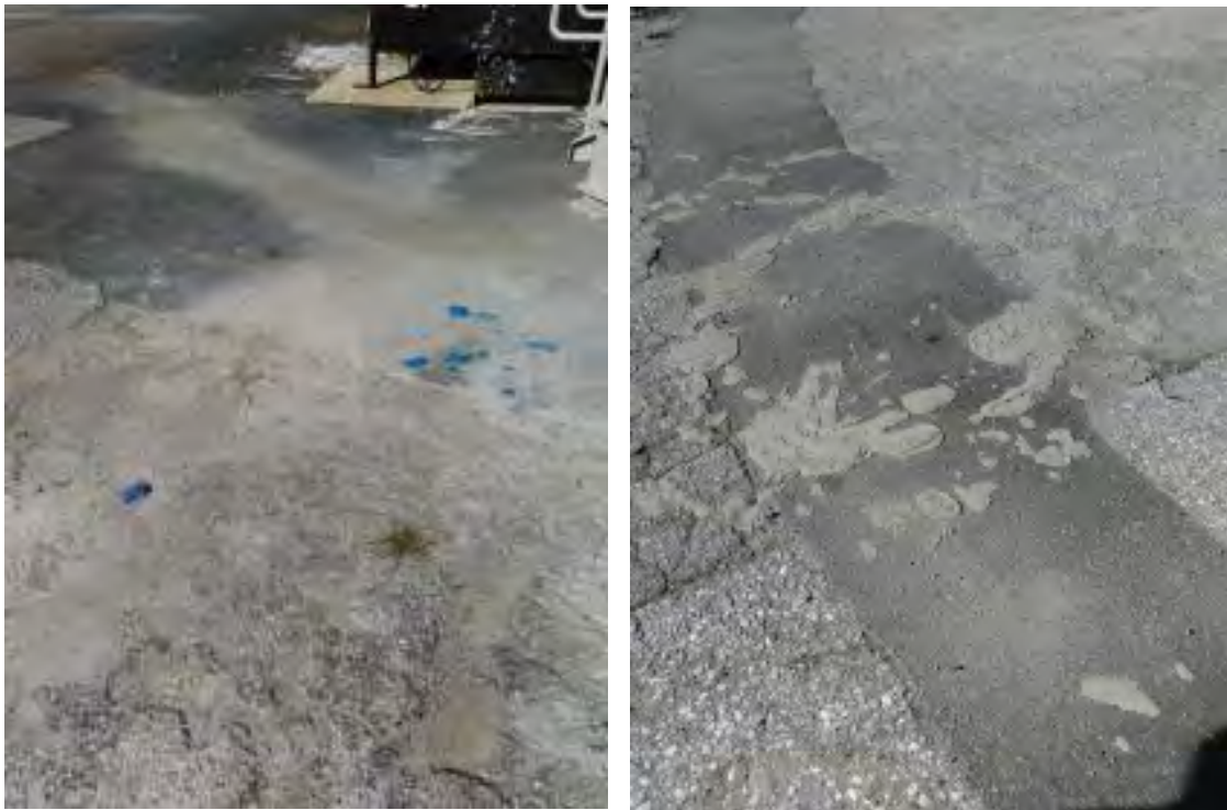
Figure 5: Smaller patches of blue (left) and gray (right) hardened Dryvit product scattered on pavement within approximately 30 ft of rear retail space door.
