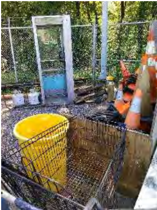
Figure 9: Gas can storage, other materials storage requiring secondary containment
