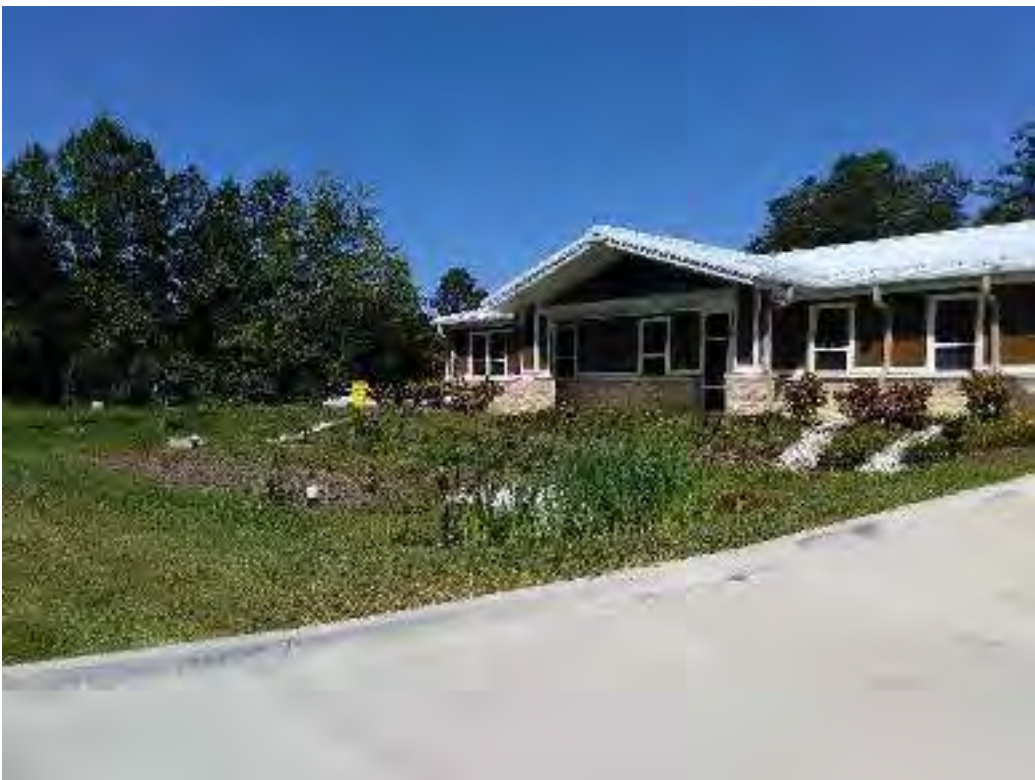
Figure 5: Stormwater pond receiving rooftop runoff
