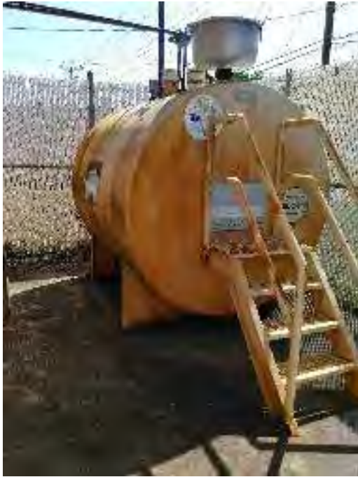
Figure 10: Fuel tank in front of old Lake Shore Fire Co 20 facility
