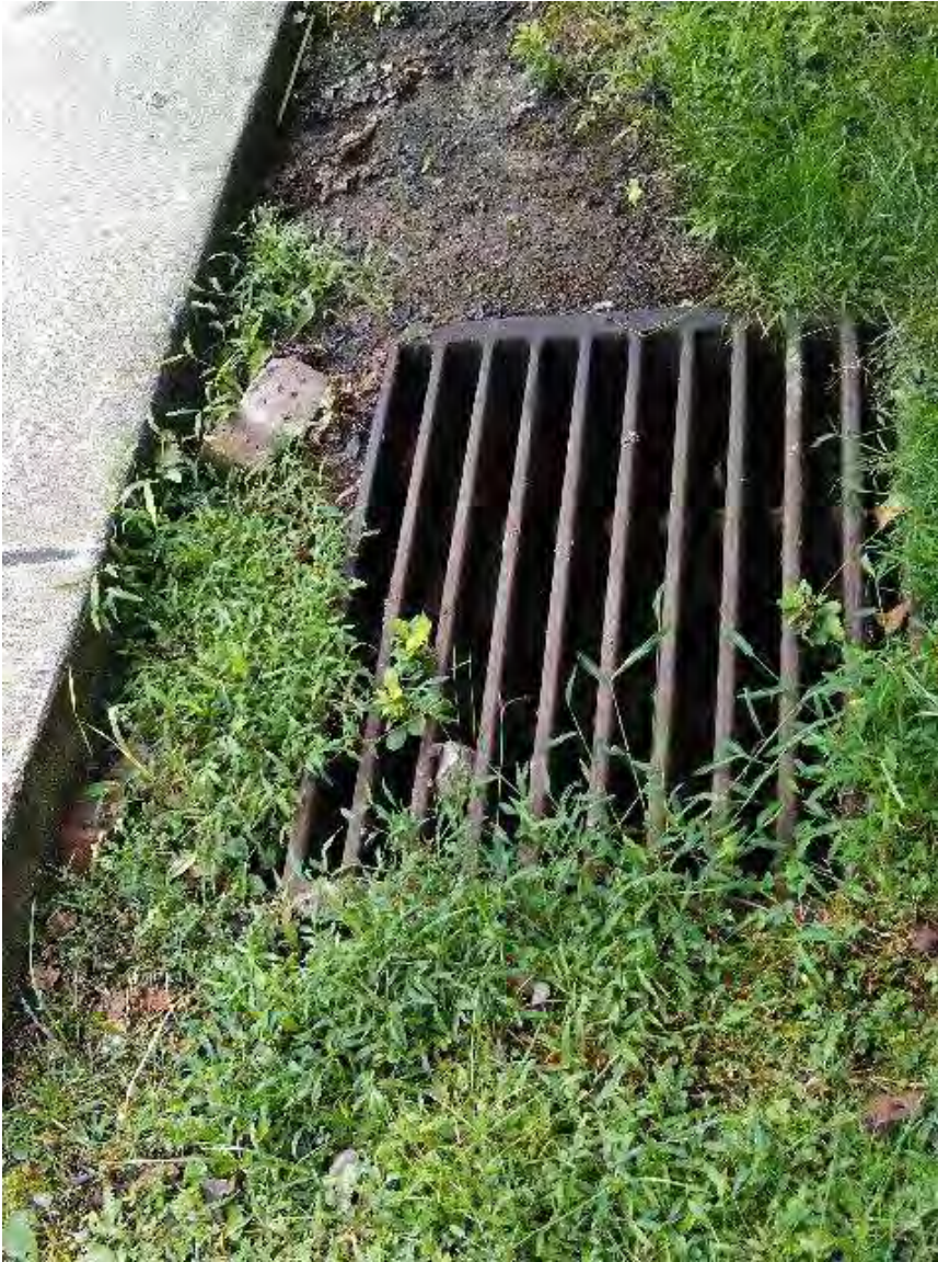
Figure 2: Stormdrain inlet near rear of parking lot.
