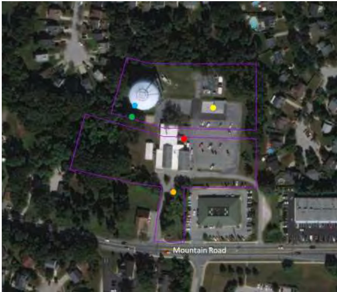
Figure 1: Aerial map of Jacobsville Fire Station Blue Circle = water tower spillway Red Circle = uncover soil, behind silt fence Orange Circle = front inlet Yellow Circle = fueling station Green Circle = outfalls
