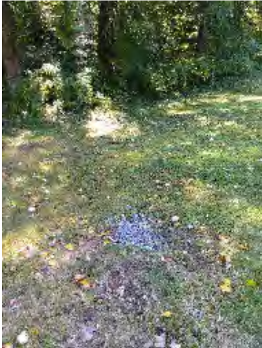
Figure 8: Outfall discharge area.
