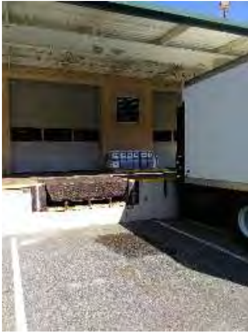
Figure 8: Proper liquid storage in loading dock.
