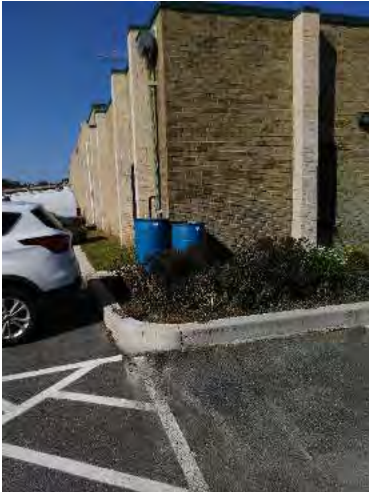
Figure 12: Rain barrels on downspout located on southeast corner of warehouse building.
