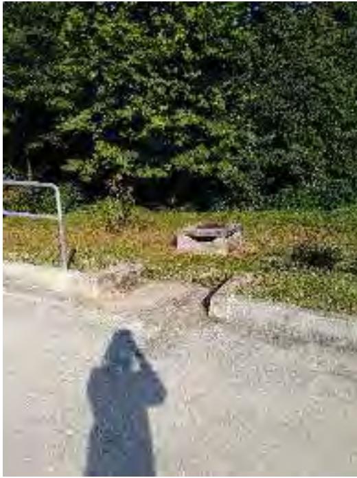
Figure 3: Curb cut inlet from front drive way into dry pond.
