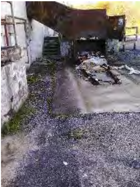
Figure 3: Trash compactor chute without dumpster; view 2
