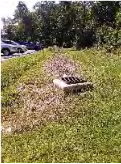
Figure 3: Western stormwater pond adjacent parking area
