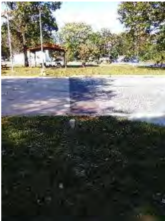
Figure 9: Pavement cut under which a pervious pipe is draining the groundwater.
