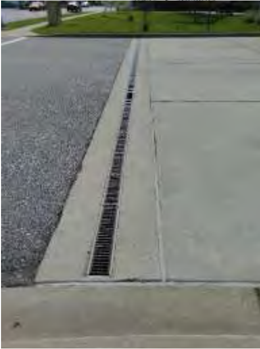
Figure 5: Trench drain
