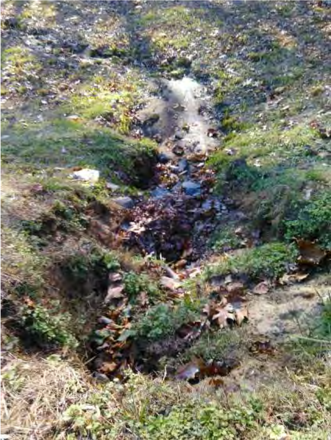
Figure 3: Erosion downstream of Outfall T150001
