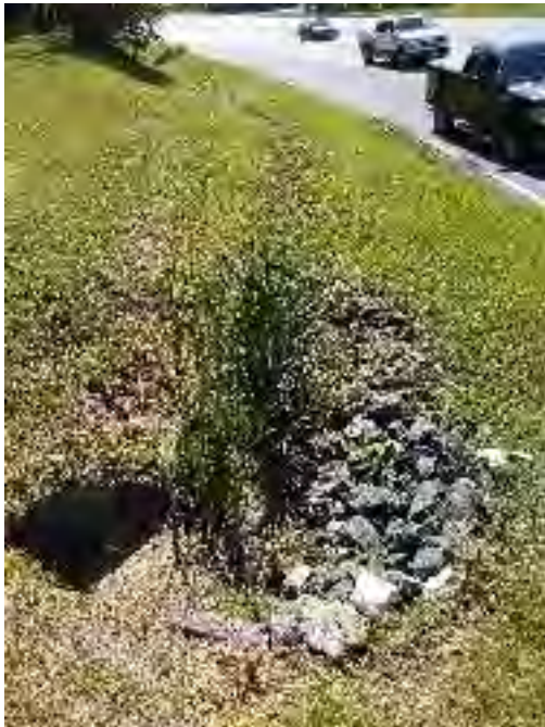
Figure 5: Outfall M110006 riprap and grass channel.
