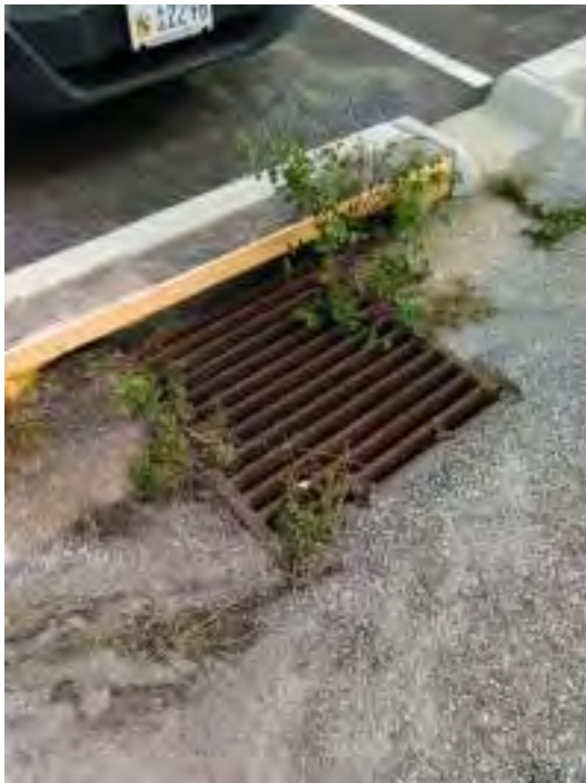
Figure 3: Partially vegetated inlet
