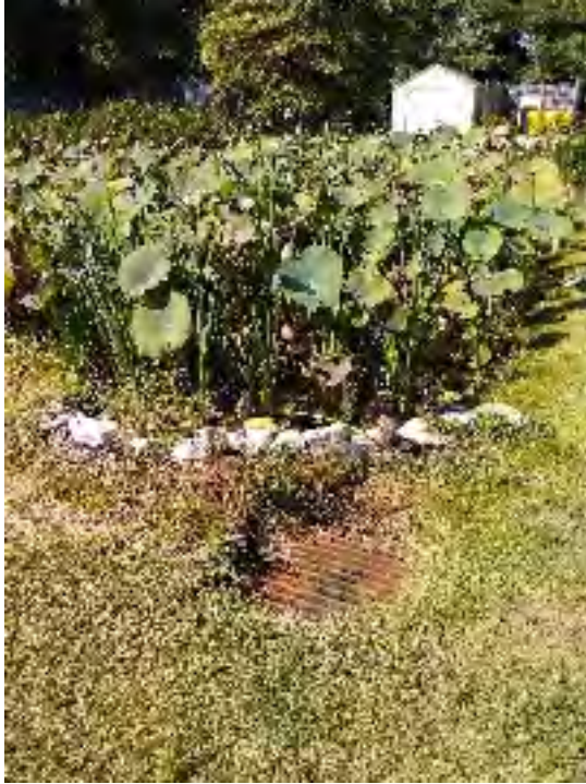
Figure 4: Stormdrain inlet draining western pond
