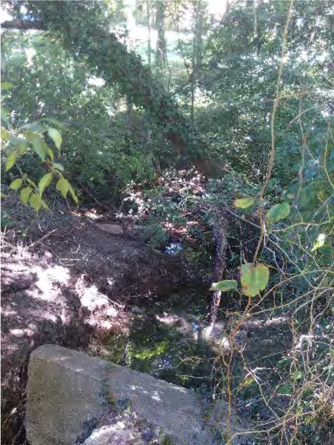
Figure 2: Erosion surrounding Outfall L090021 and downstream
