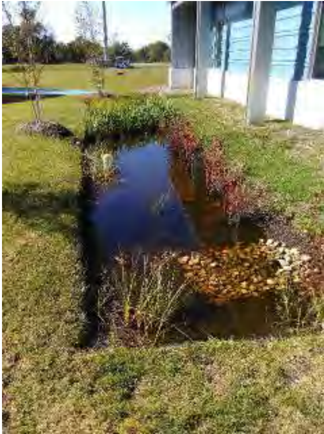
Figure 14: Newly installed BMP north of new training building.
