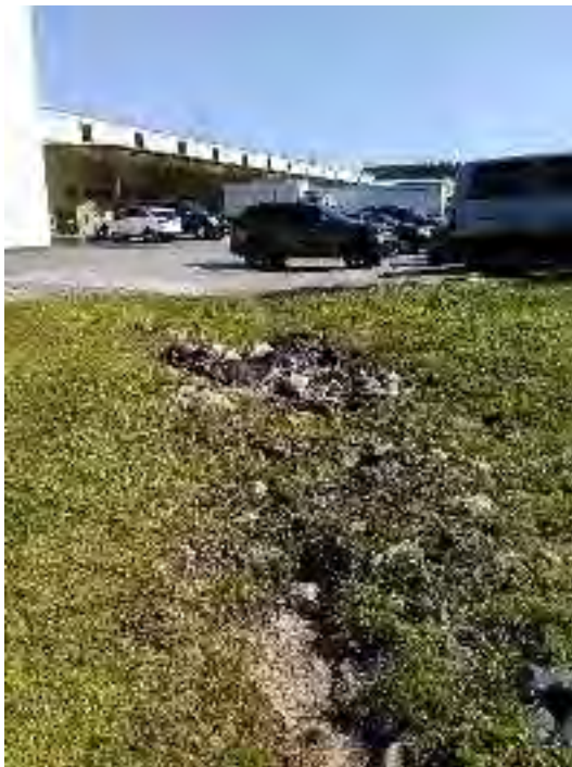
Figure 3: South parking lot drainage channel and grass/rip rap lined channel.
