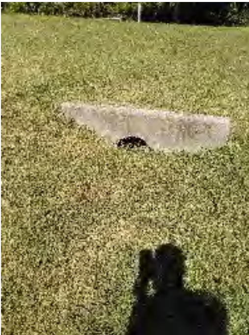
Figure 3: Concrete headwall at the end of the grass conveyance channel.
