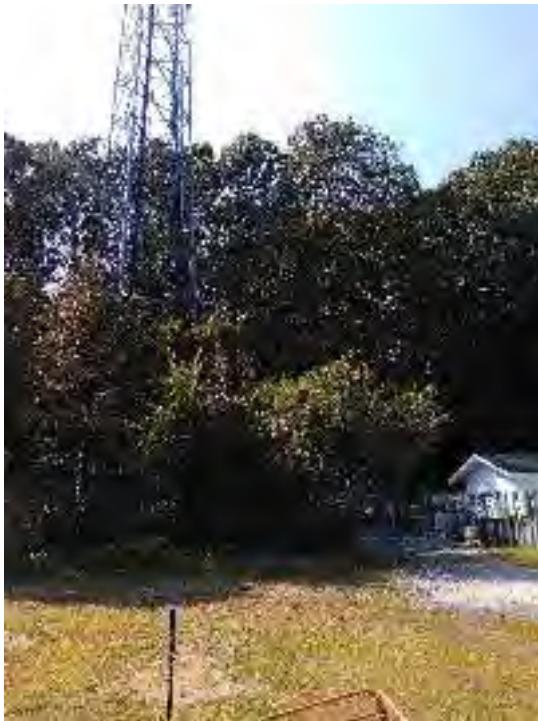
Figure 2: Radio tower on adjacent property.
