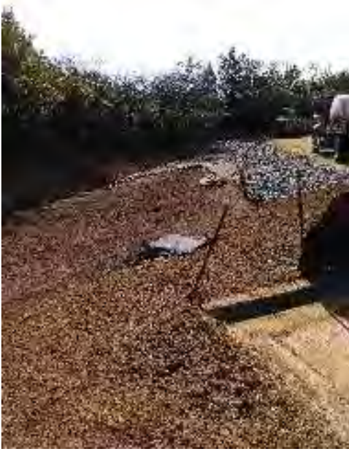
Figure 4: Fresh earthwork done in rear of property.
