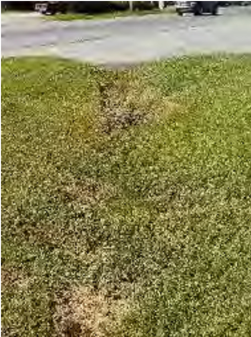
Figure 2: Curb cut entrance to grass conveyance channel on eastern edge parcel.
