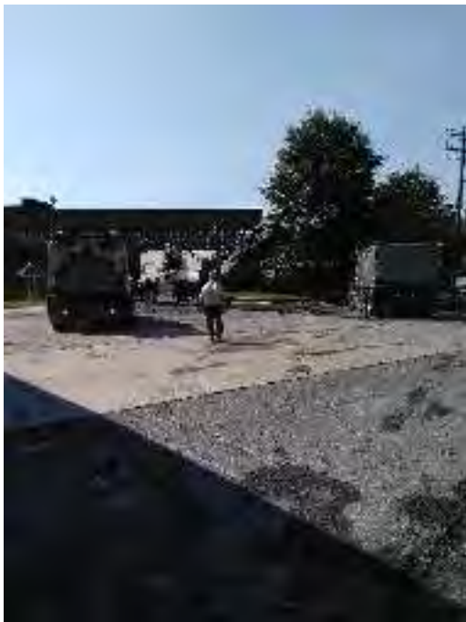
Figure 3: Front driveway pad undergoing construction.
