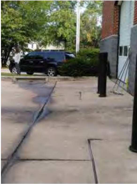
Figure 4: Vehicle Washing Area located immediately behind the Brooklyn Fire Co. 31 Station.
