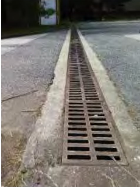
Figure 2: Trench Drain
