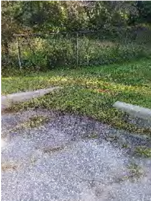
Figure 2: rear parking lot drainage through curb cut.
