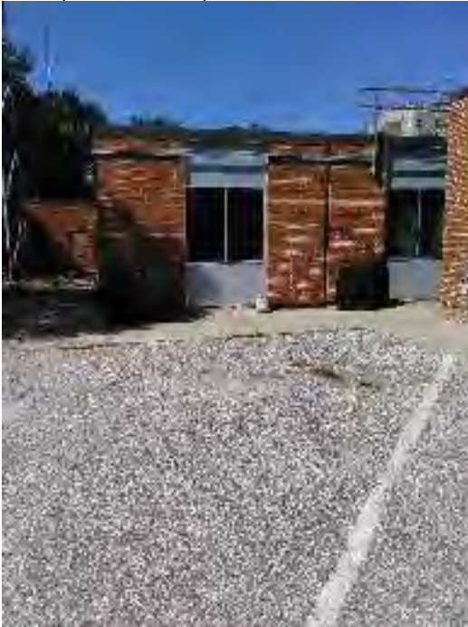
Figure 2: Improper liquid storage
