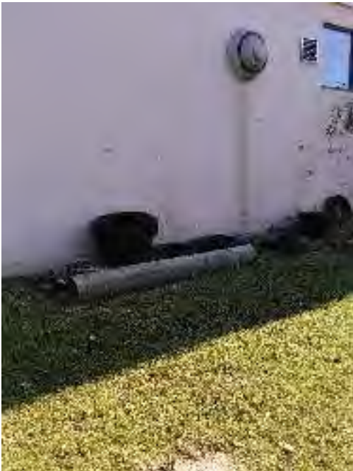
Figure 9: Improper bulk solid storage along north edge of property.
