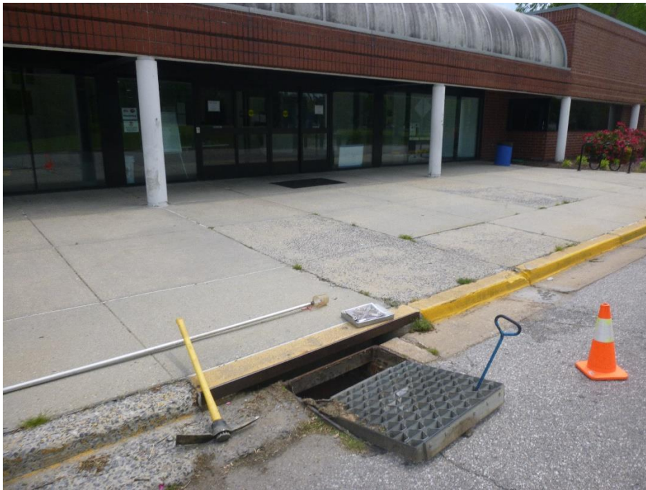
Figure 4. Inlet in front of Arundel Olympic Swim Center
