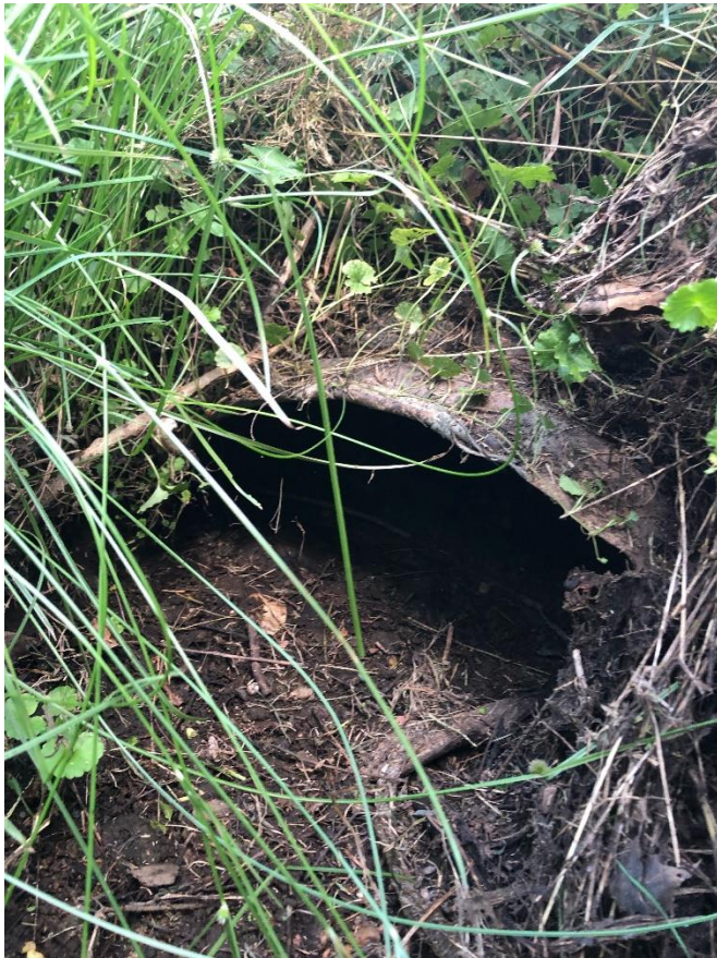
Figure 1. A view of the outfall Q34O002
