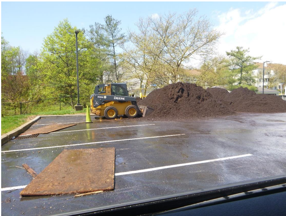
Figure 1. A view of an uncovered pile of mulch stored on the parking lot approximately 15 feet from an inlet (center left)
