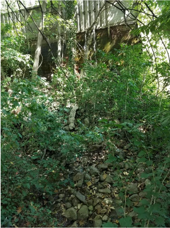
Figure 2. A view of the steep slope immediately adjacent to the retaining wall; note the flowing water passing between the bottom of the privacy fence and the top of the wall (top center)
