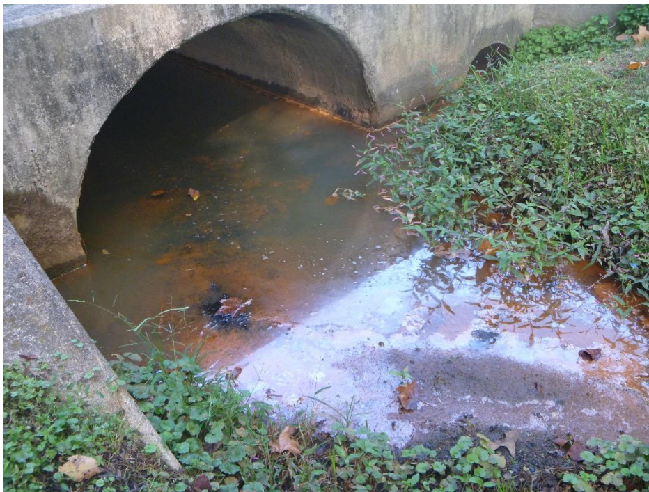
Figure 1. Conditions at outfall O22O014 on September 27; note the sheen on the water and the clumps of orange deposits — both indicate colonies of iron-oxidizing bacteria
