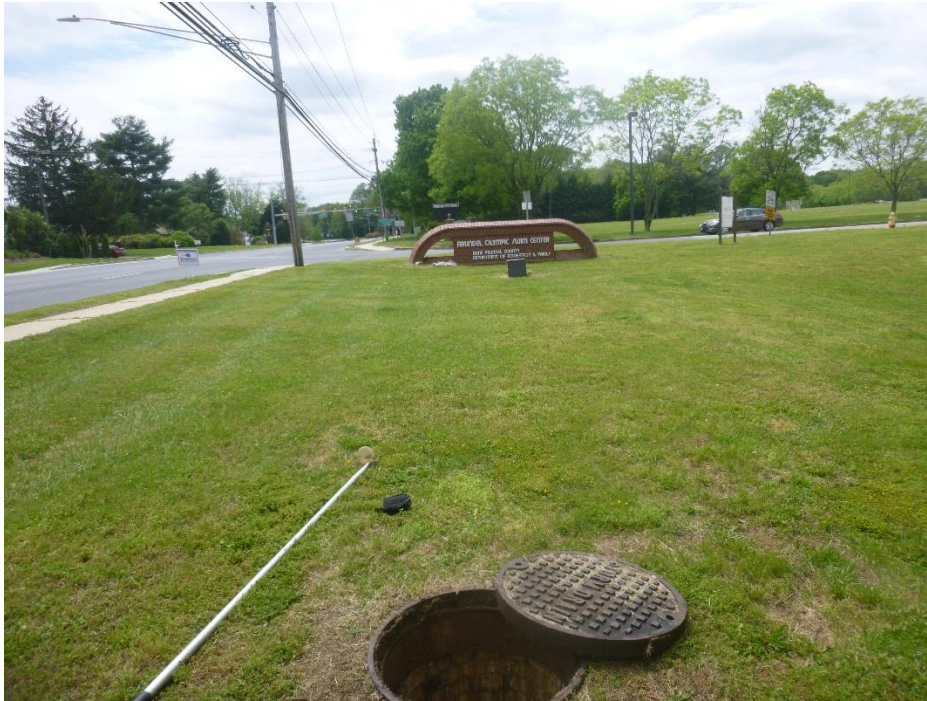
Figure 2. Junction manhole near intersection of Riva Road with Fred Stauffer Lane
