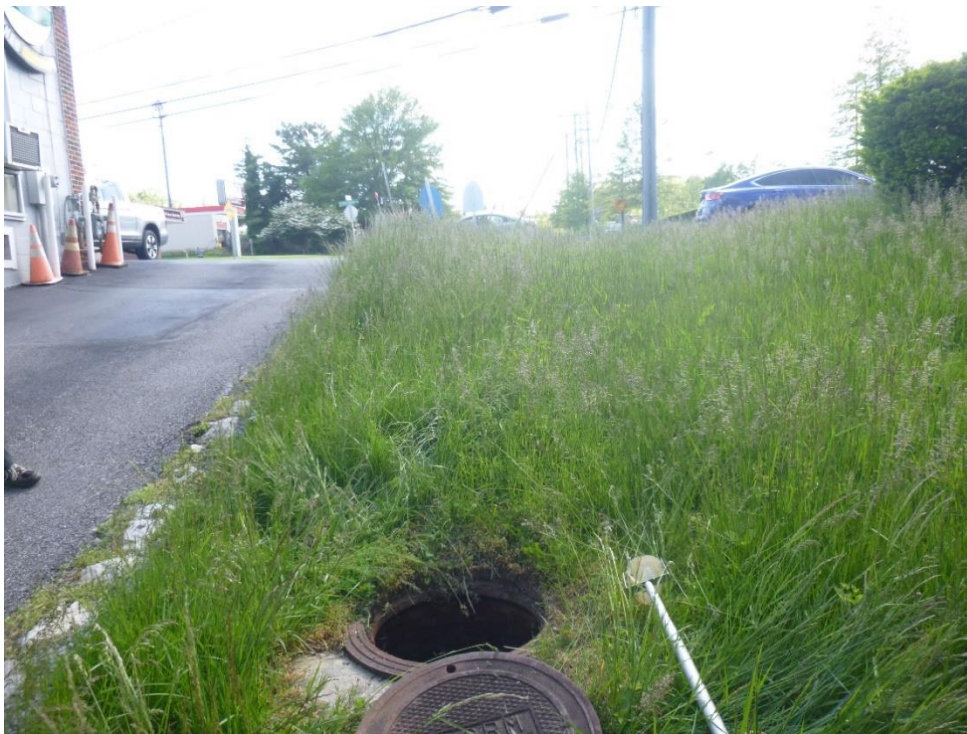
Figure 2. Manhole immediately up-network from outfall T16O006
