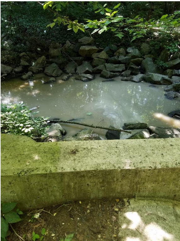
Figure 2. A view of the grey discharge (center right) expanding into the plunge pool; grey foamy globules are evident between the rocks close to the outfall opening
