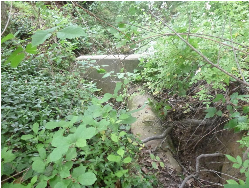
Figure 1. A view of the eroded ground behind the endwall (background) and along the connected pipe (foreground) of outfall L23O001
