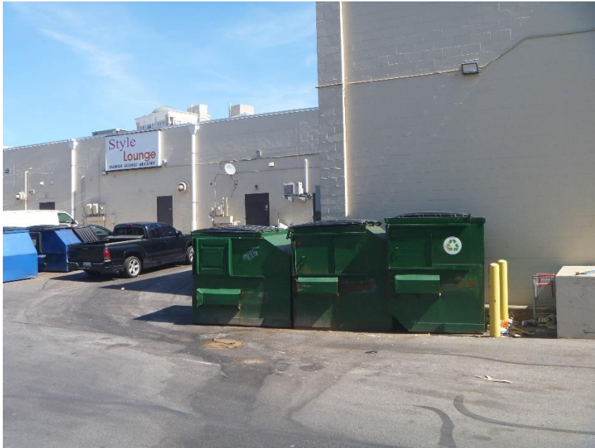
Figure 3. A view of several stain paths (left and bottom center) behind the Restaurante Jalapeños restaurant; the inlet that received the drainage from this area of the pavement was out of the photograph, below the bottom center
