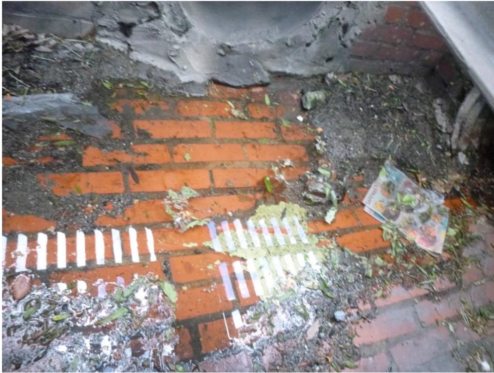
Figure 3. Flowing water observed in inlet on north side of Arnold Road
