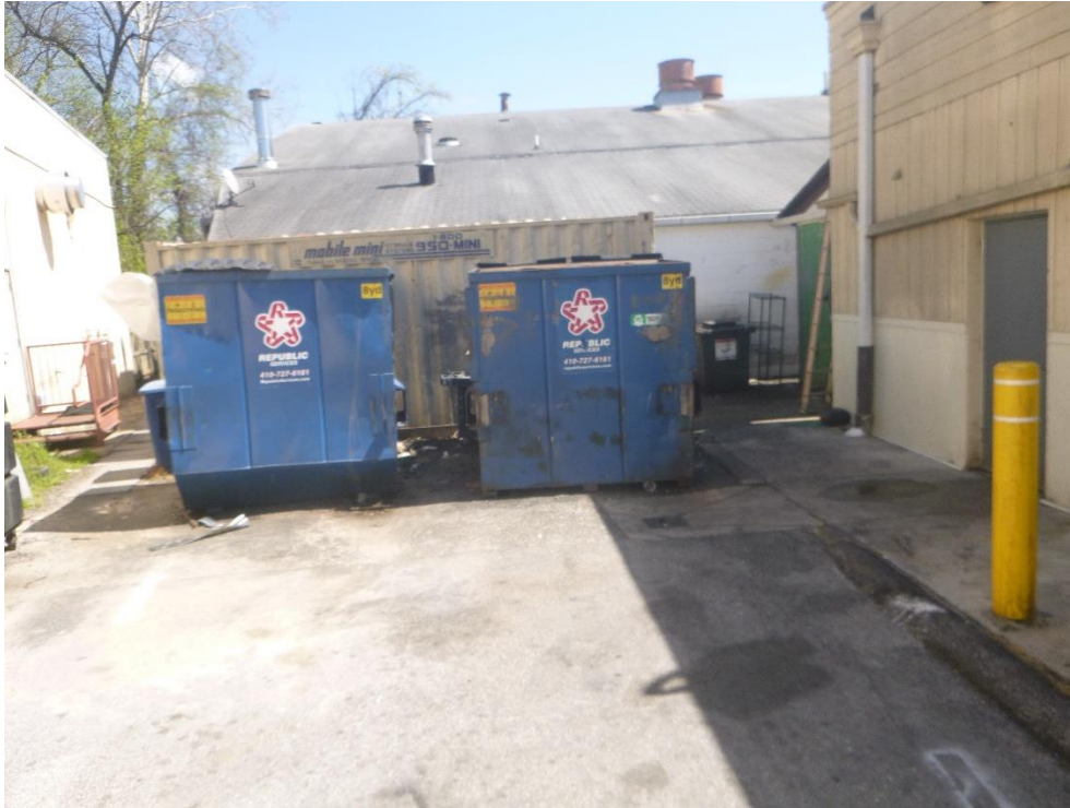
Figure 4. A view of the uncovered storage area for the dumpsters and grease bin; note the grated drain in front of the dumpster shown on the right
