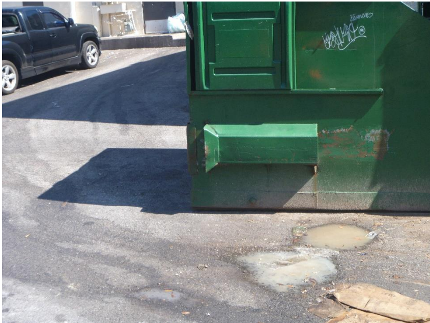
Figure 2. Three puddles found on the pavement near the dumpster closest to the kitchen grease bin seen in Figure 1; one puddle was cloudy, beige liquid with a white sheen; the other two appeared to be solidified grease; note the arc-shaped stain path on the left leading from the door (left background)
