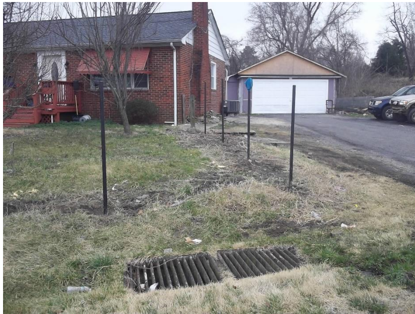
2/22/2023 Inspection – Catch basin with gray tinged water
