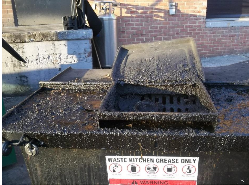
3/20/2023 Inspection – Grease on top of grease bin
