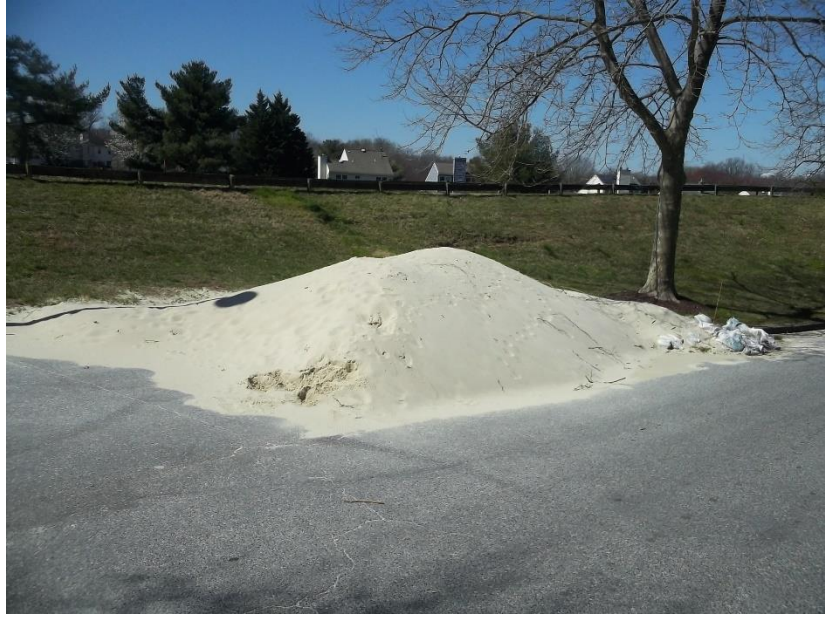
3/20/2023 Inspection – Uncontained sand pile
