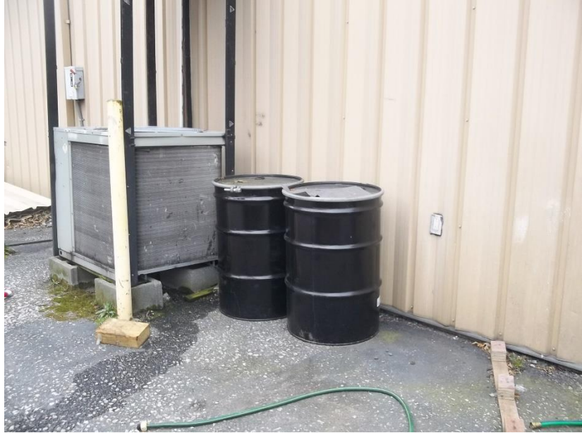
3/10/2023 Inspection – Chemical drums behind the building
