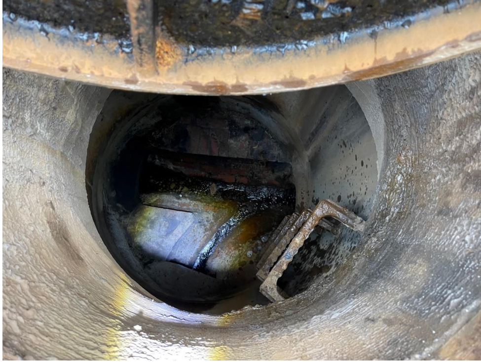
3/20/2023 Inspection – Next upstream manhole from above, wet but not flowing.
