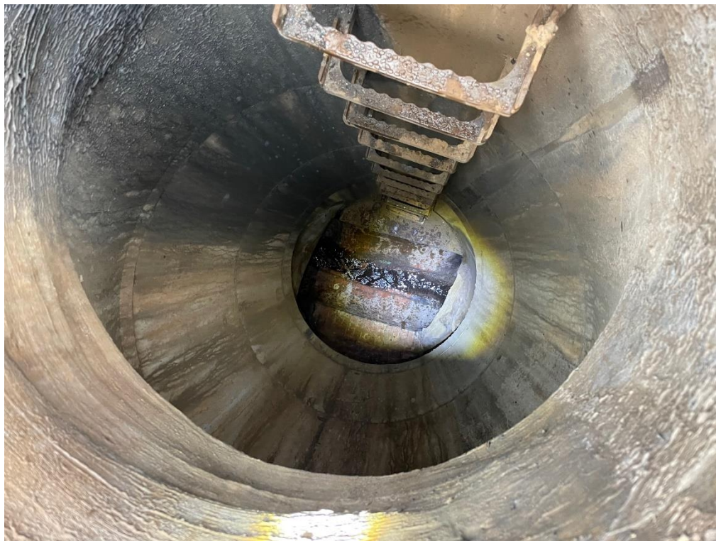
3/20/2023 Inspection – Upstream of outfall C100001, top of observed flow.
