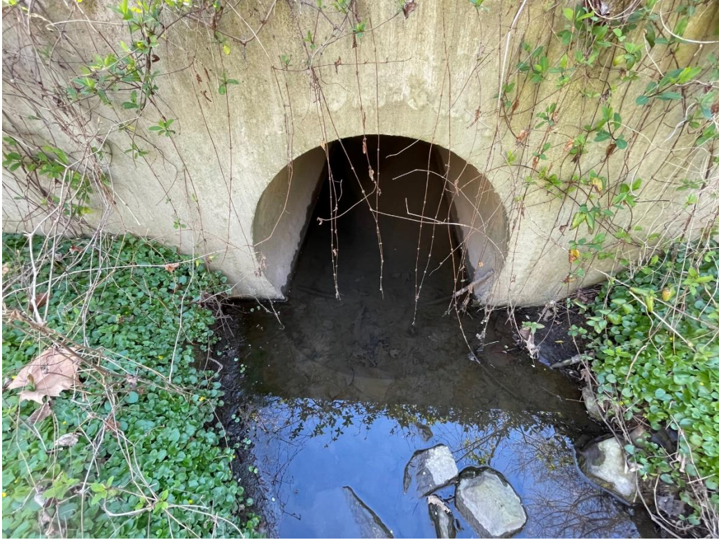
P1 3/30/2023 Inspection – Outfall K020001 overview.
