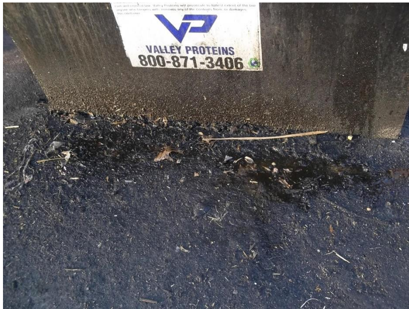
3/20/2023 Inspection – Grease on pavement
