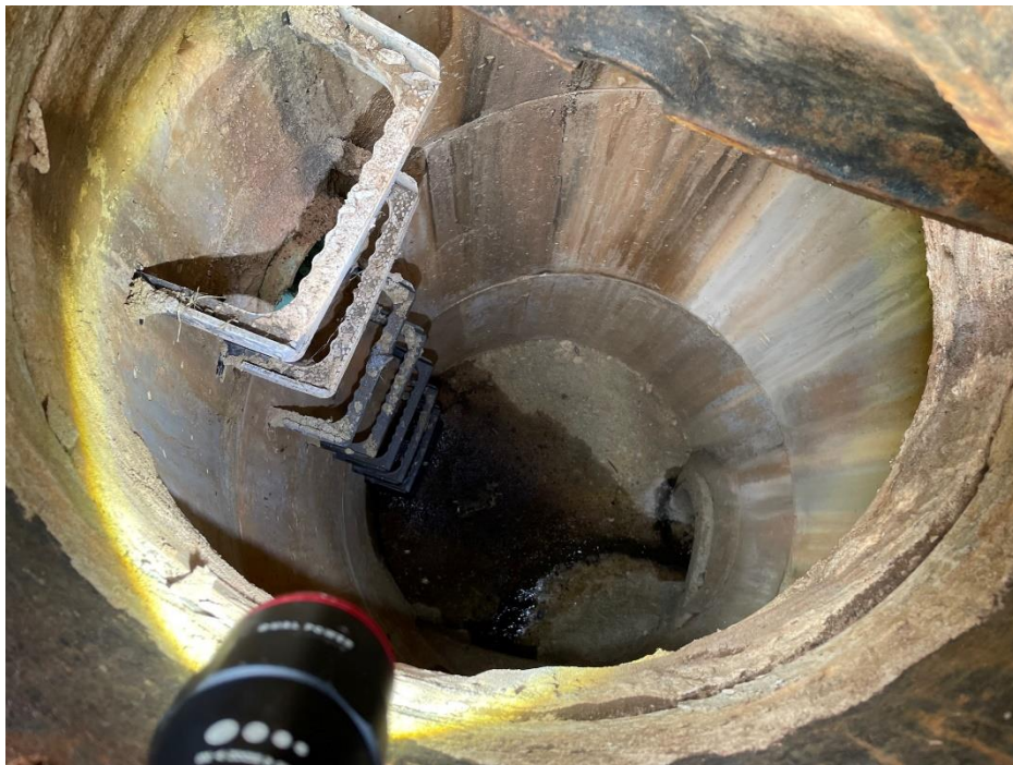
3/22/2023 Inspection – Sampled manhole upstream of right pipe.
