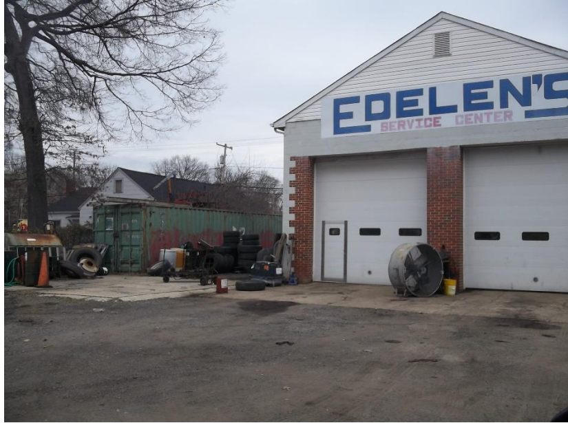
3/10/2023 Inspection – Staining on the pavement
