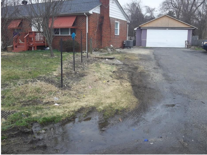
2/22/2023 Inspection – Garage with alleged bathroom draining to storm drain
