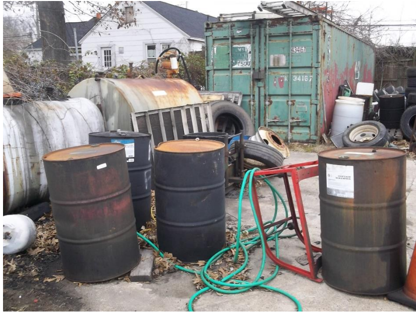
3/10/2023 Inspection – Chemical drums not properly store under cover with staining on the pavement
