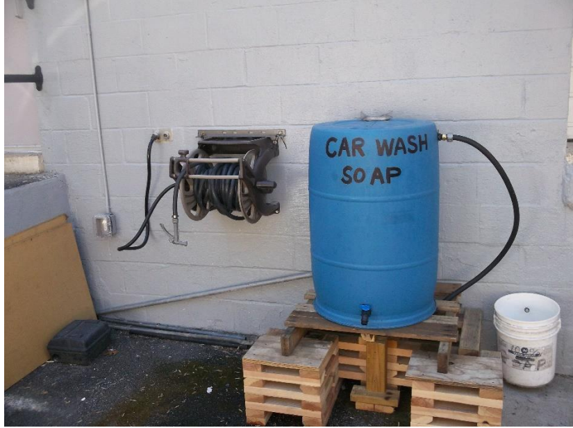
3/7/2023 Inspection – Car washing equipment
