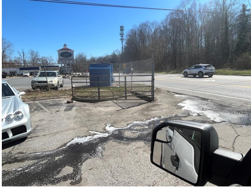
3/7/2023 Inspection – Washwater draining to roadway
