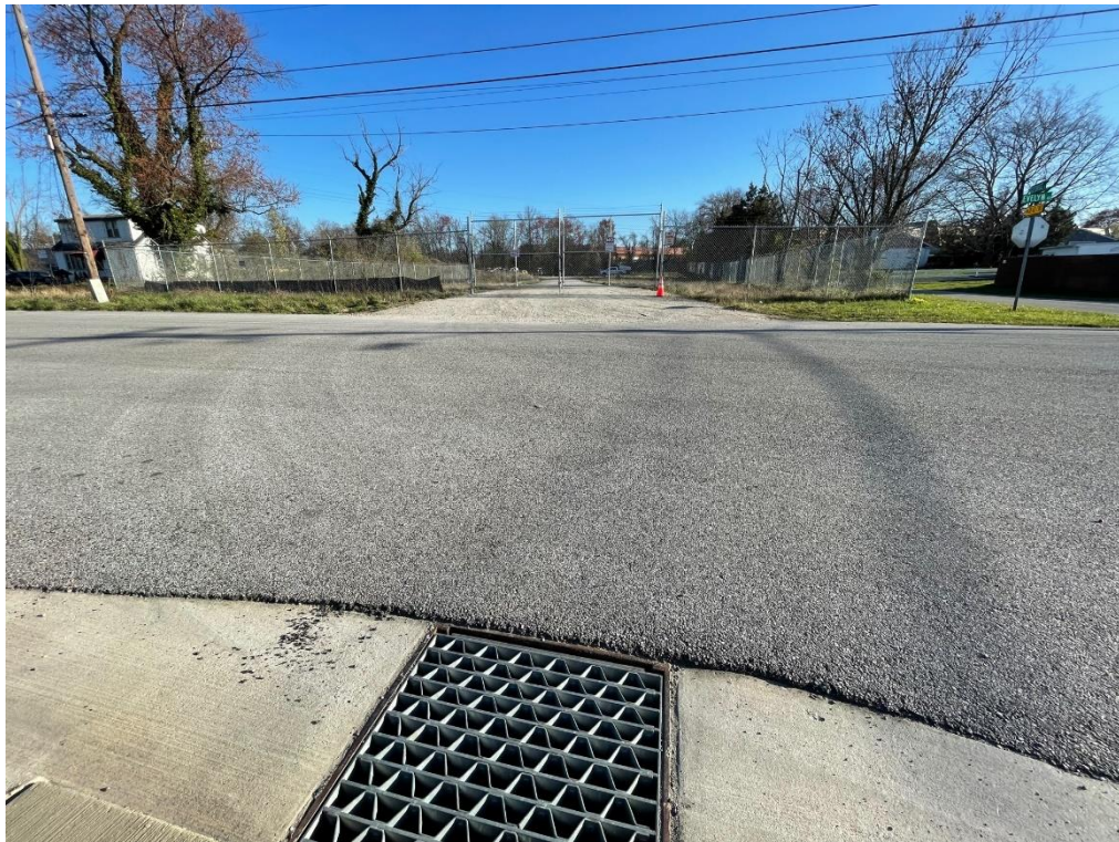
P4 3/30/2023 Inspection – Drainage area of the above inlet.
