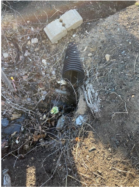
P7 3/30/2023 Inspection – Sampled pipe.
