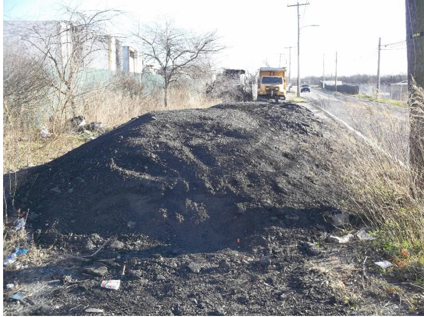
3/7/2023 Inspection – Uncontained stockpile
