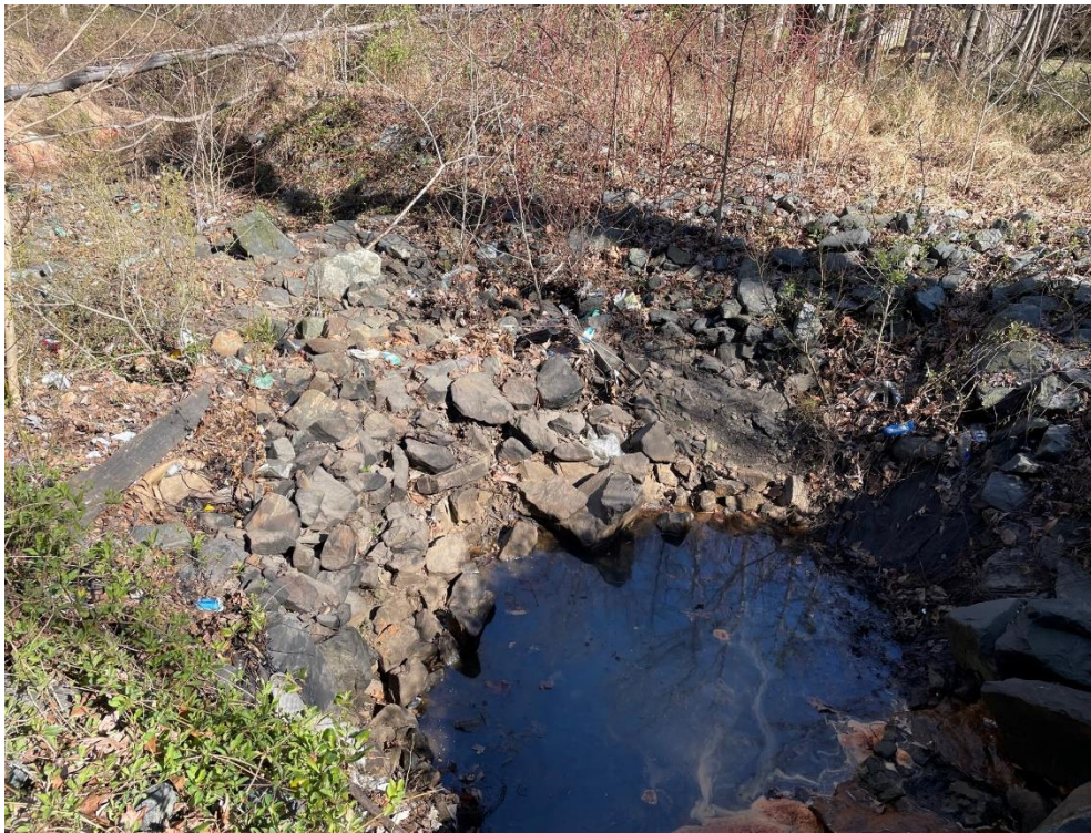
3/15/2023 Inspection – Outfall B110011 downstream, plunge pool.
