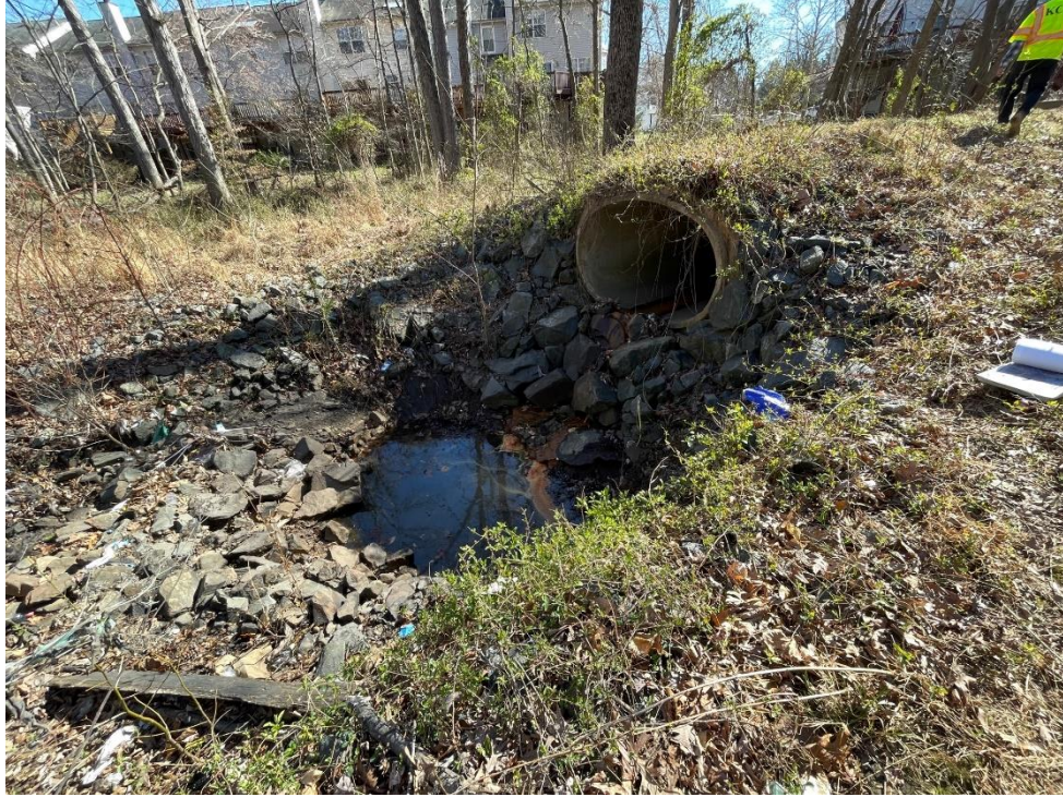
3/15/2023 Inspection – Outfall B110011 overview.
