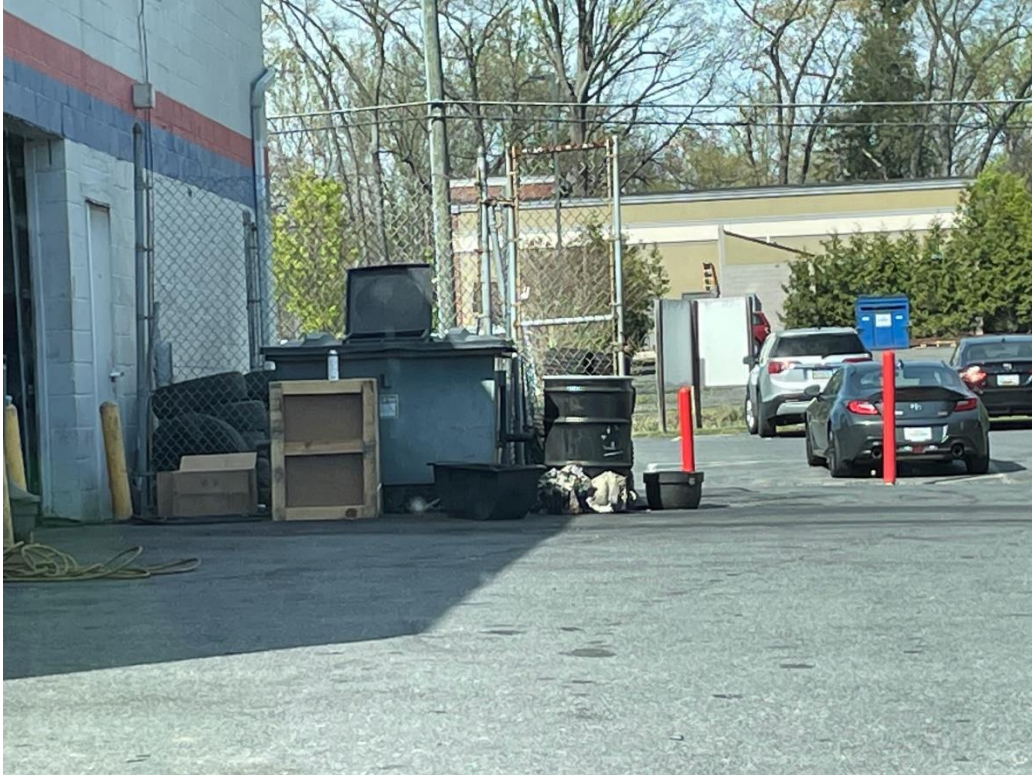
4/11/2023 Inspection – Staining on pavement and open waste grease bin.
