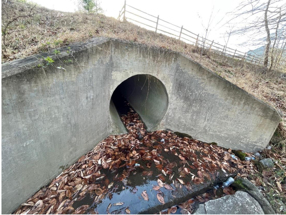
3/20/2023 Inspection – Outfall C100001 overview.
