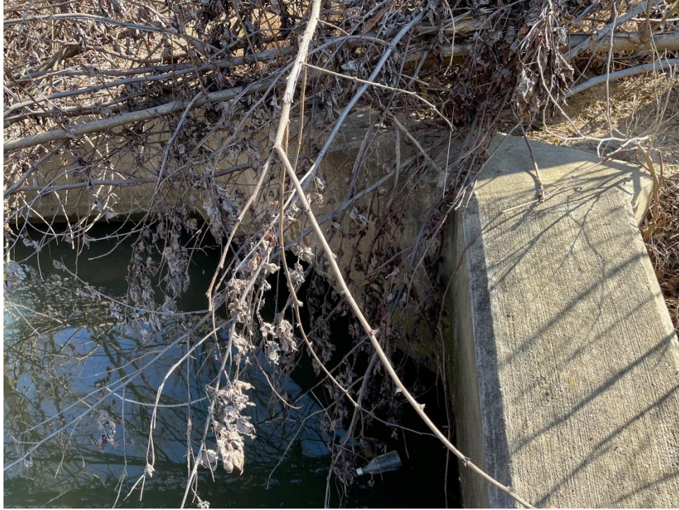
3/21/2023 Inspection – Outfall F08O032 overview.
