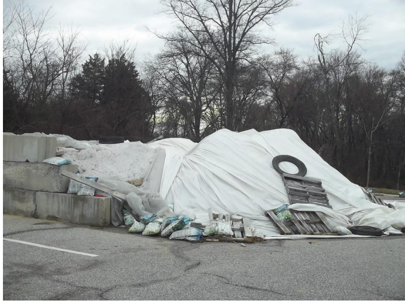
2/23/2023 Inspection – Exposed salt pile
