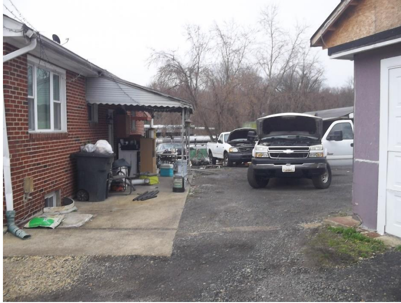
2/22/2023 Inspection – Vehicle maintenance
