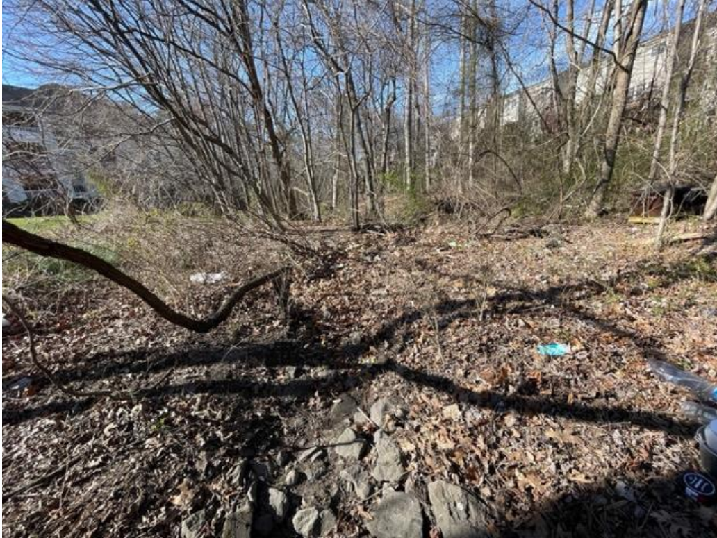
3/16/2023 Inspection – Downstream view from Outfall C11O029.
