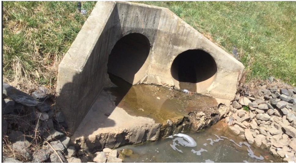
3/21/2023 Inspection – Outfall F07O003 overview.
