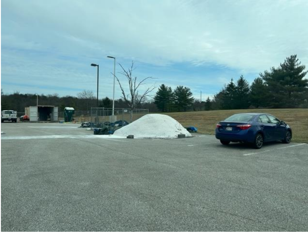
2/27/2023 Inspection – Uncovered salt pile.
