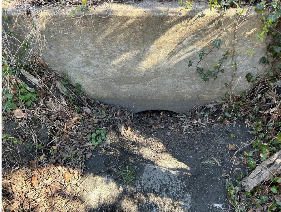
3/15/2023 Inspection – Outfall R200011 overview.
