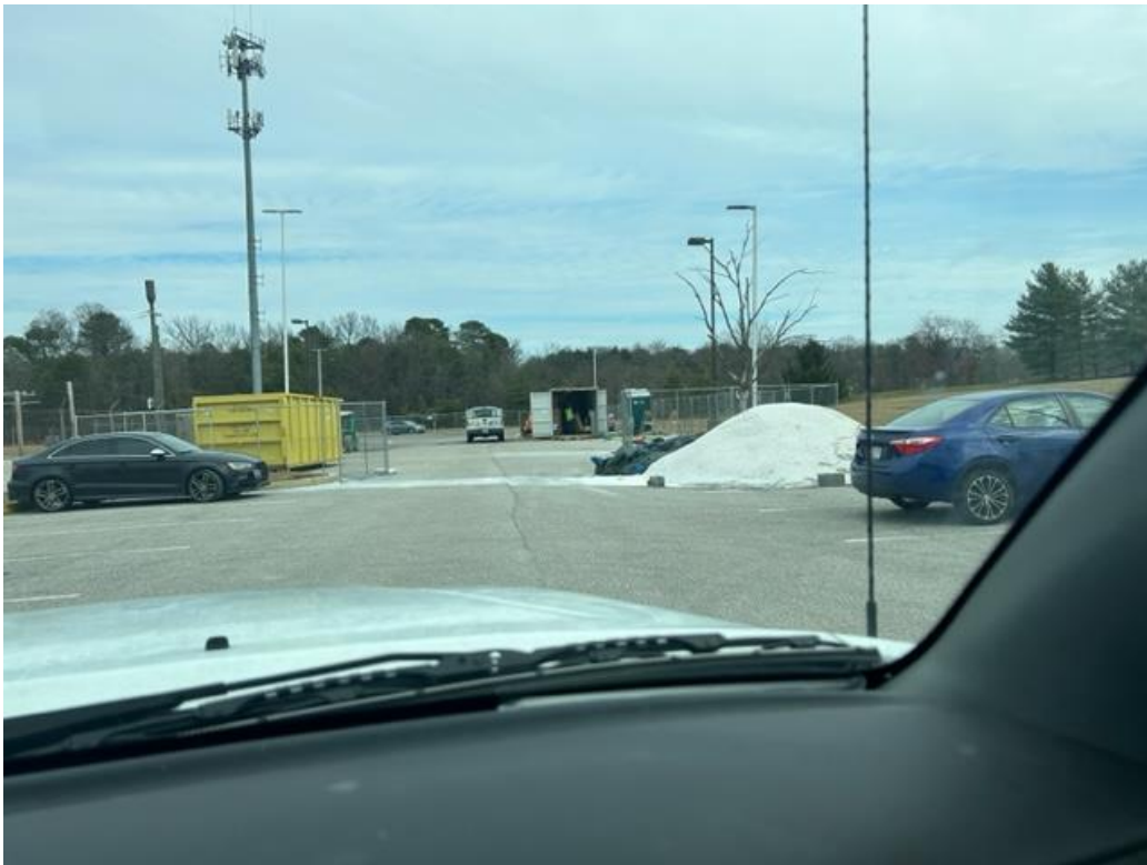
2/27/2023 Inspection – Salt stains from uncovered salt pile.
