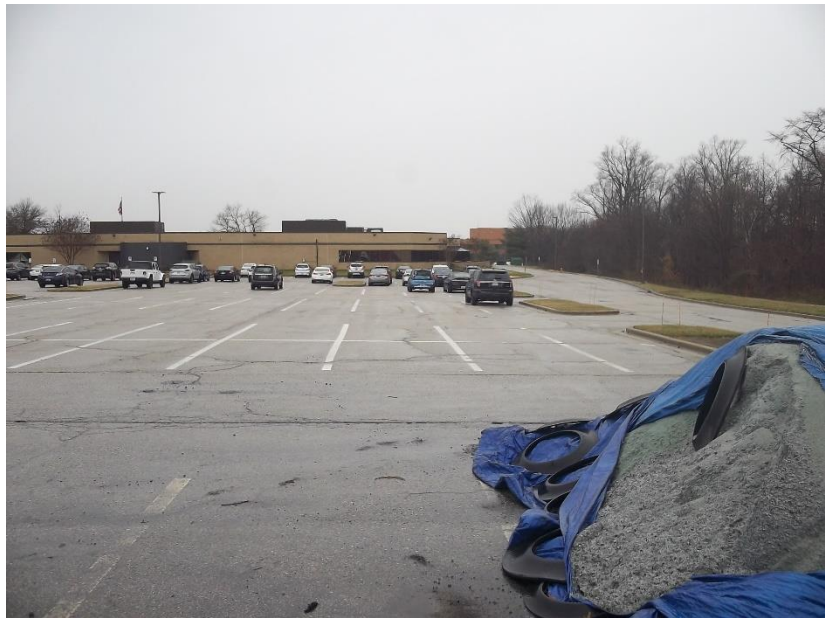
2/22/2023 Inspection – Exposed salt pile
