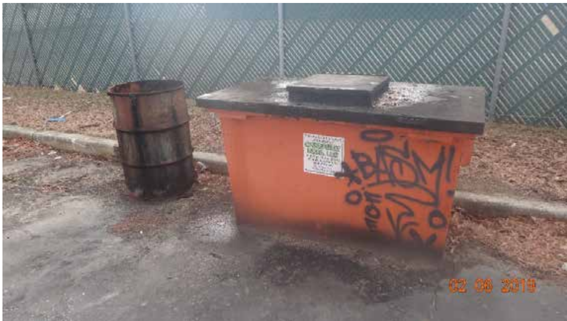
Figure 1. A kitchen waste grease bin found with dark grease stains on the pavement surrounding the bin, behind several restaurants in the Mountain Road Plaza shopping center on February 6; note the open drum to the left in the photograph
