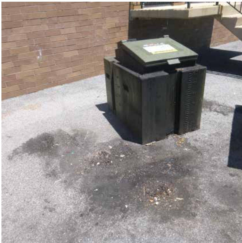
Figure 1. A kitchen waste grease bin found on July 9; note the dark grease stains on the pavement near the bin
