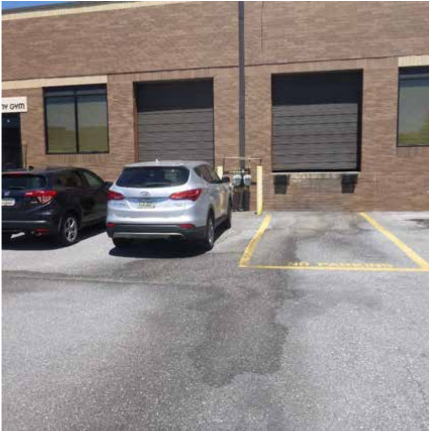
Figure 2. A view of stains on the pavement that extended from a loading dock door; this section of the parking lot was immediately adjacent to the area shown in Figure 1 (upper right edge)
