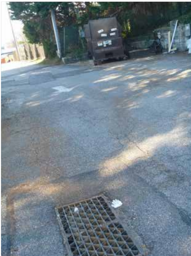
Figure 3. Evidence of residue from dumpster operations flowing to a nearby inlet
