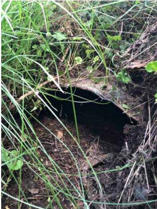
Figure 1. A view of the outfall Q34O002
