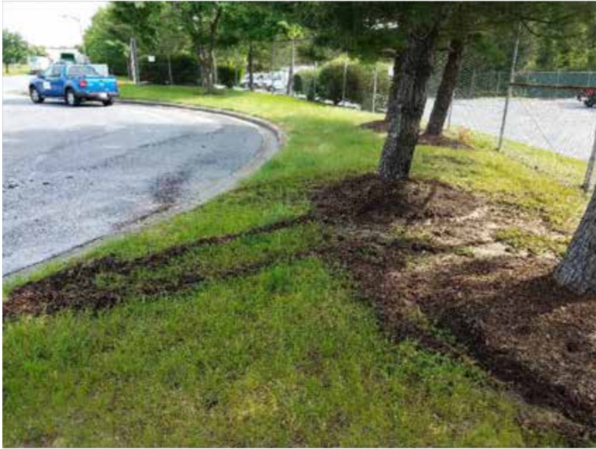
Figure 5. A view of disturbed mulch at the cul-de-sac; the mulch appears to have been pushed from the right side of the photograph, at the fence line
