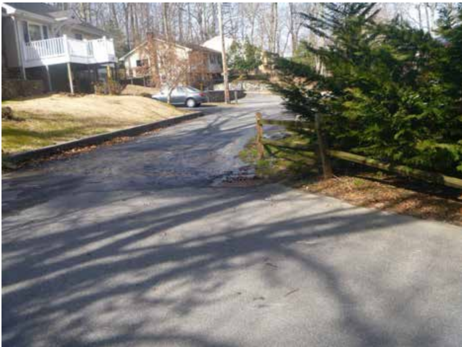
Figure 2. Evidence of a hose discharge (from the residence on the left) entering an inlet near 510 Hoot Owl Road; the source of the water was a backyard pool
