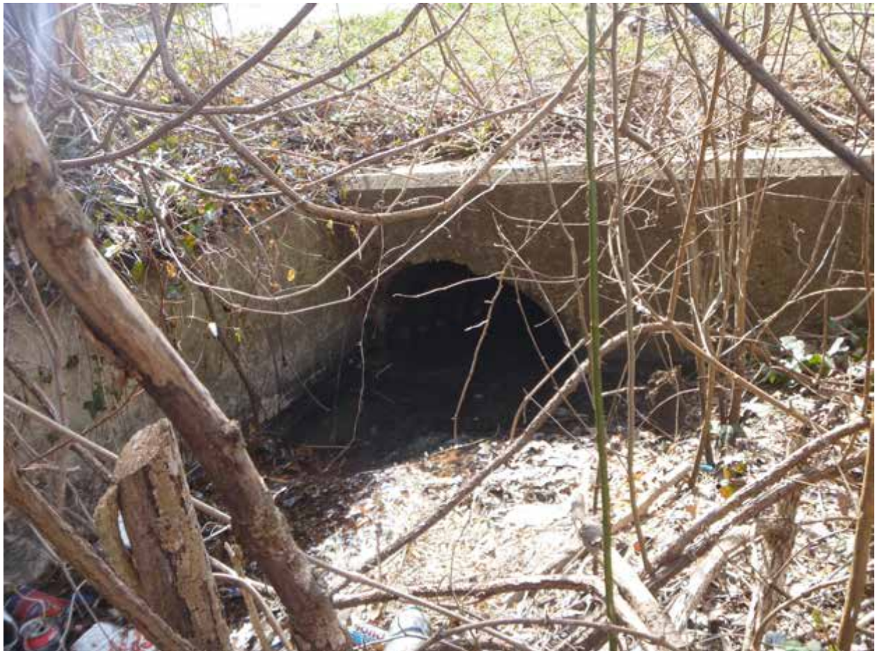
Figure 1. A view of conditions at Outfall T16O006 on March 7, 2019
