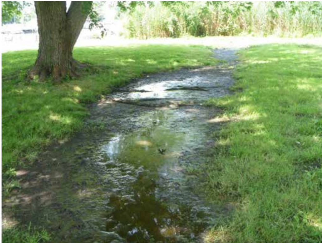
Figure 4. A view of the flat plain that receives and distributes the discharge from the outfall see in Figure 1 and the drainage ditch seen in Figure 2; Rockhold Creek is visible in the background of the photograph
