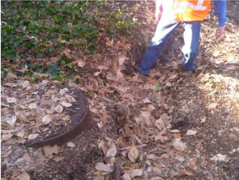
Figure 1. Evidence of soil subsidence immediately adjacent to the manhole
