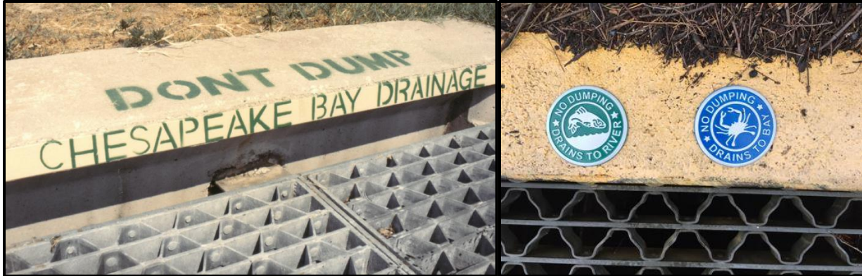
Figure 7. Storm drain stencil (left) and medallion (right) used by Anne Arundel County.
