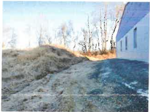
Stockpile altered drainage to sediment trap
