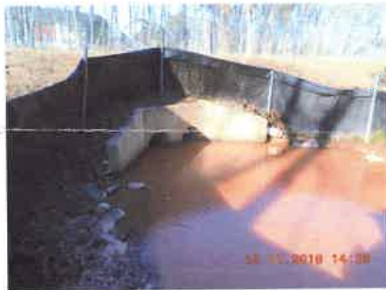
Basin outfall discharged suspended clays
