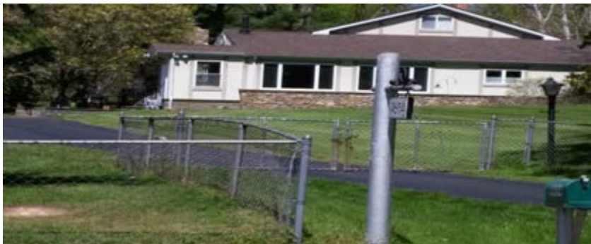
Close-up of the downspout. Note that runoff flows onto vegetated area and then to wooded areas.
