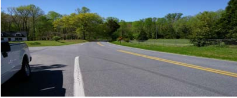
Open section road disconnection to vegetated area
