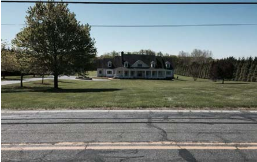
Roadway sheet flow to vegetated filter strip area
