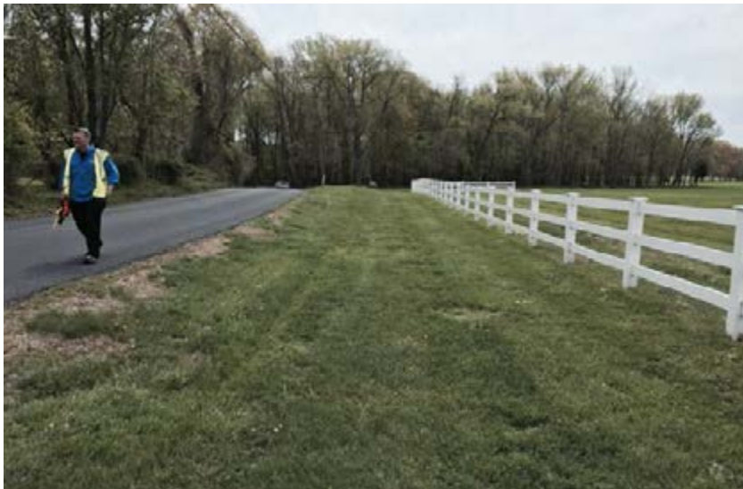
Flat, wide bottom representative roadside swale- This discharges into a wooded conservation area
