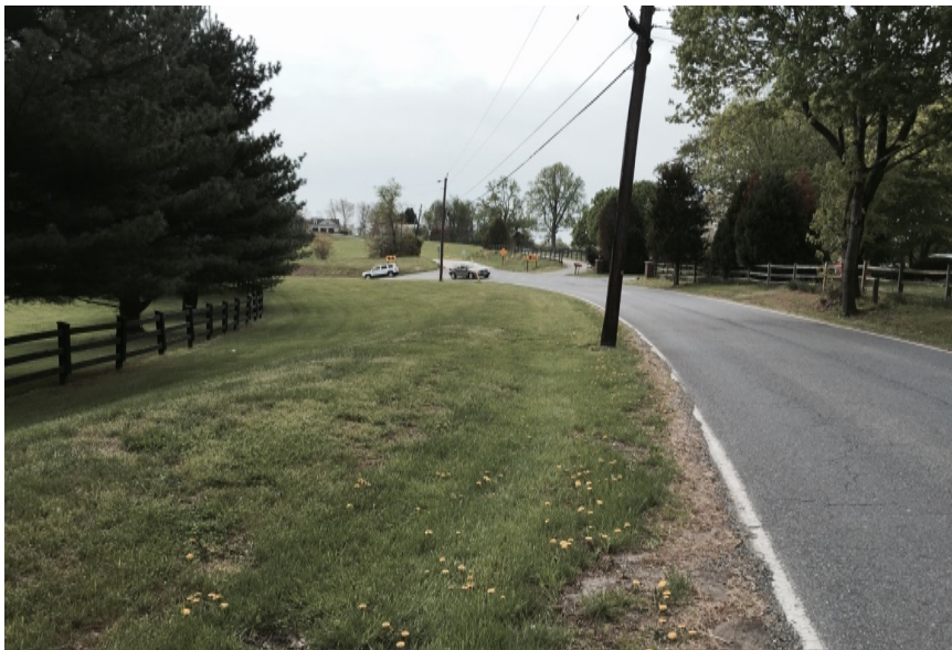
Road impervious disconnection and sheet flow to vegetated/grassed areas
