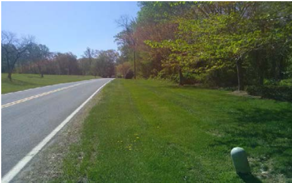
Vegetated swale along the open section road (South along St. Stephens Road). See field notes and sketch for ridge line and flow in the swales. Note that the swale slope is less than 4%.
