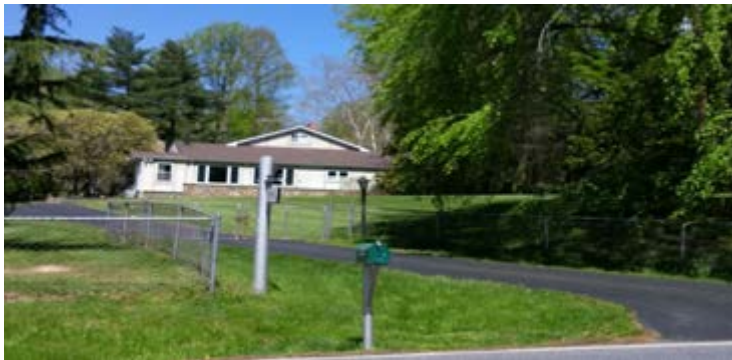
Rooftop disconnection onto vegetated area.
