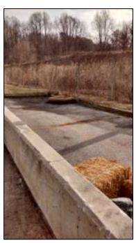
Concrete berm and coir log at at-grade stormwater inlet
