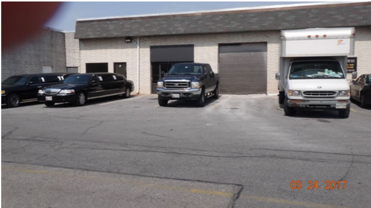
Figure 8. Evidence of possible previous washdown activity, associated with a tile fabrication business, which carried and deposited white particulates (leading away from the closed bay door; right center)
