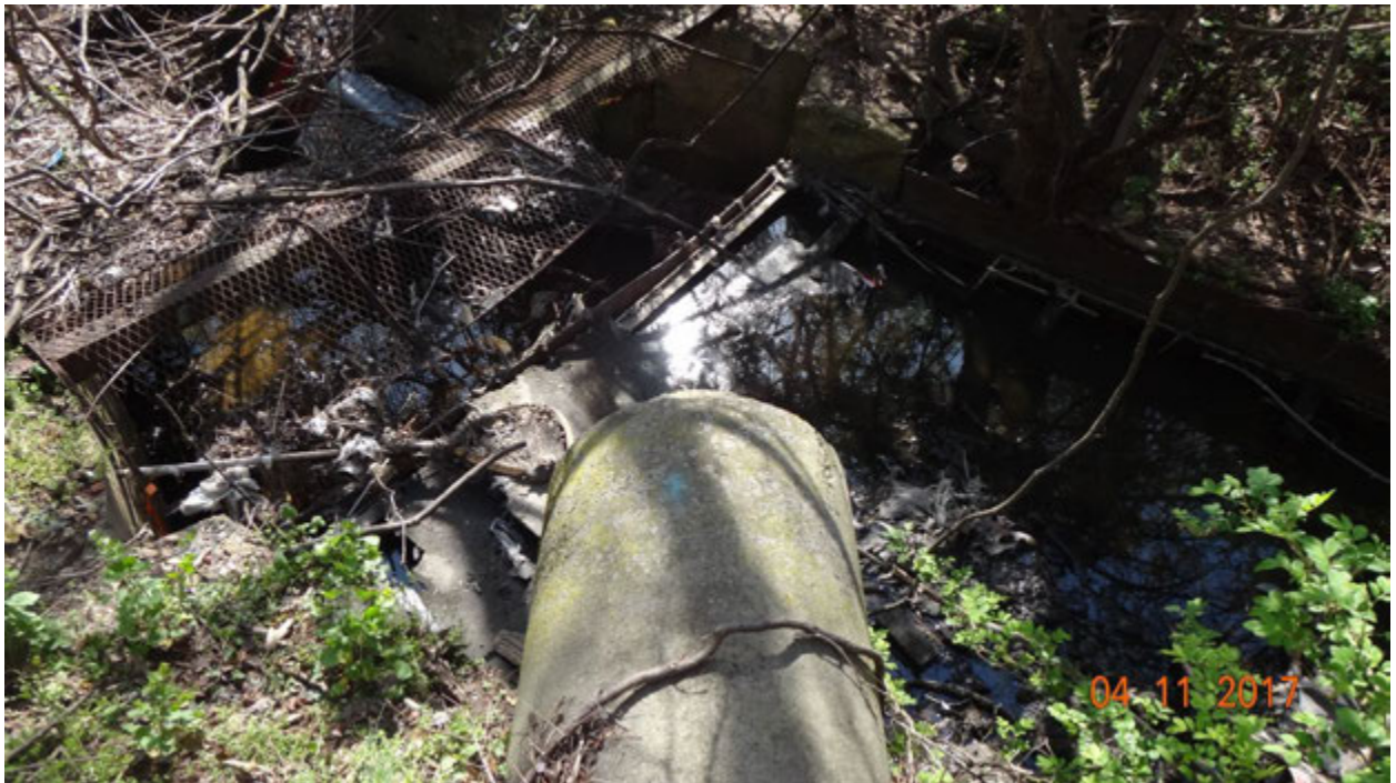
Figure 2. View of part of a super-structure constructed over the stream that supported expanded metal panels (left) and large sheets of plywood (center, under and in front of the pipe in the foreground); the grey plastic seen in the stream (upper left) is an exposed portion of a broken shopping cart
