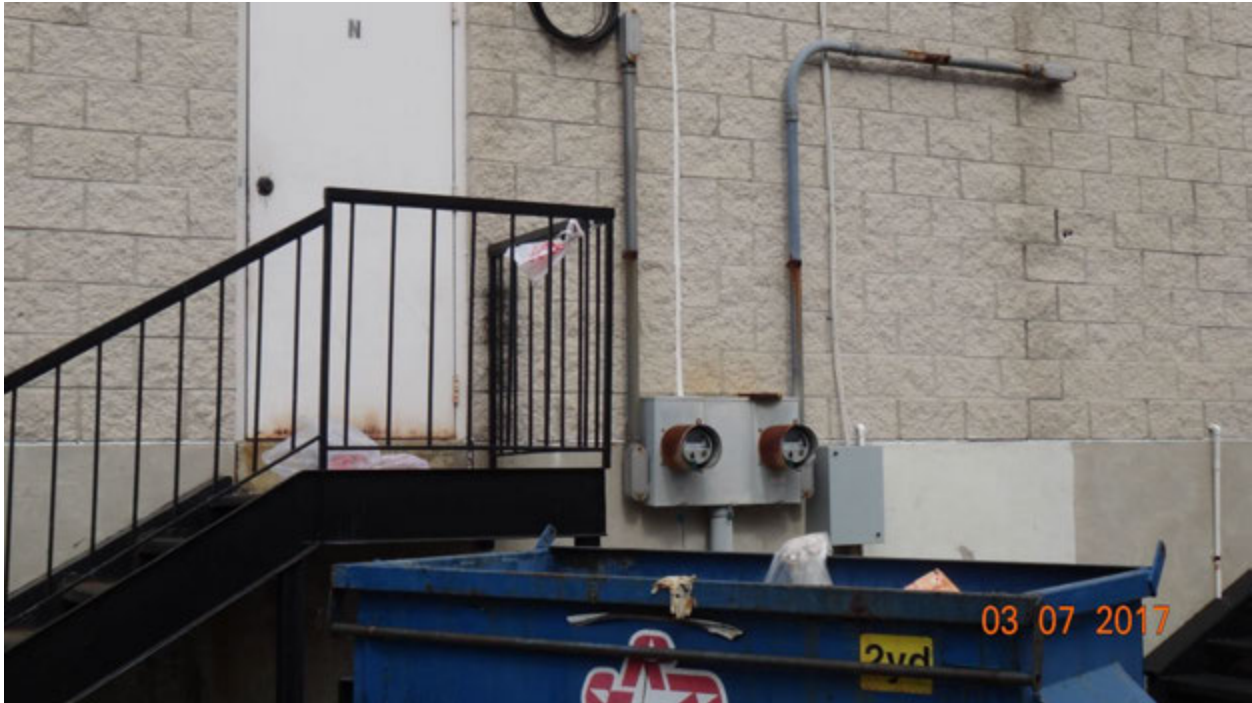
Figure 2. An open dumpster and loose trash behind the rear door for Suite N
