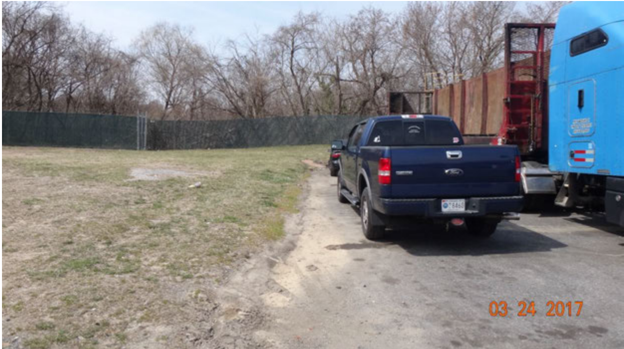
Figure 7. Evidence of accumulating sediment at the southwest edge of the parking lot; the flows associated with the stain reported in Figure 6 passed under the blue tractor-cab (right)
