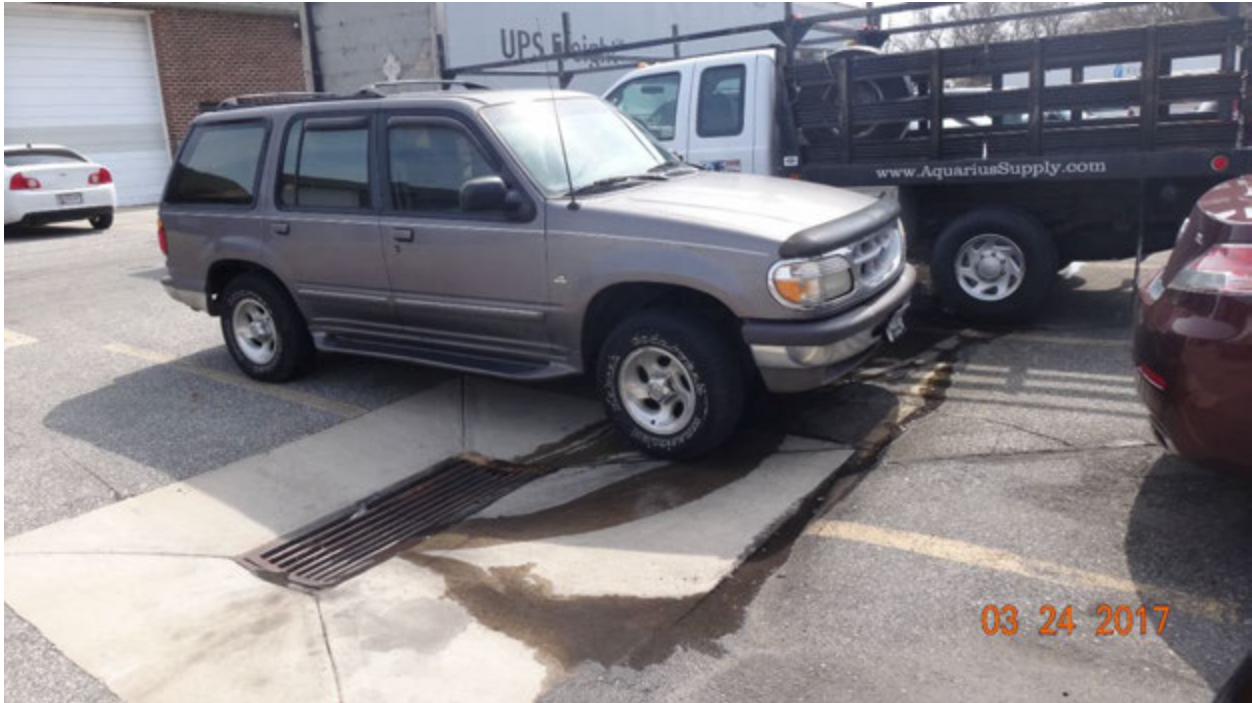
Figure 3. Excessive runoff from Bay 2 washdown activity entering a grate inlet
