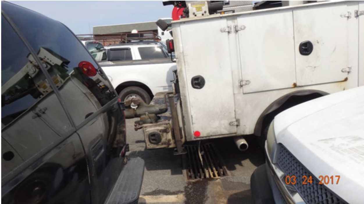
Figure 5. Evidence of fresh (wet) and previous (dried) stains indicating tainted runoff entering the grate inlet from the south (foreground); the fresh stain was associated with the runoff shown in Figure 4
