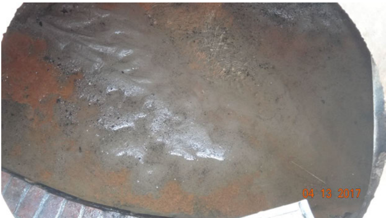
Figure 2. View inside the third manhole
