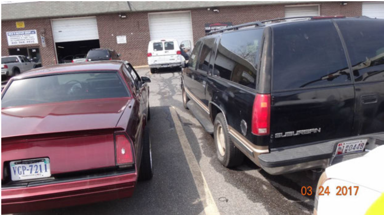
Figure 4. Fresh wet stains suggesting recent washdown activity (not observed) on the center-west side of the 512 building
