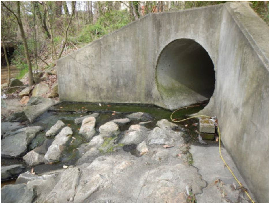
Figure 1. Conditions at outfall R20B5O005 (the secured wire was part of the apparatus in place for a different study); note the signs of green algae growth in the pipe and on the rocks in the plunge pool
