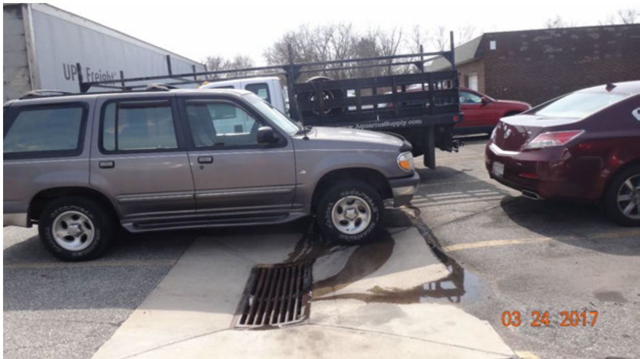
Figure 4. Evidence of the excess wash water from the vehicle washing entering the storm drain
