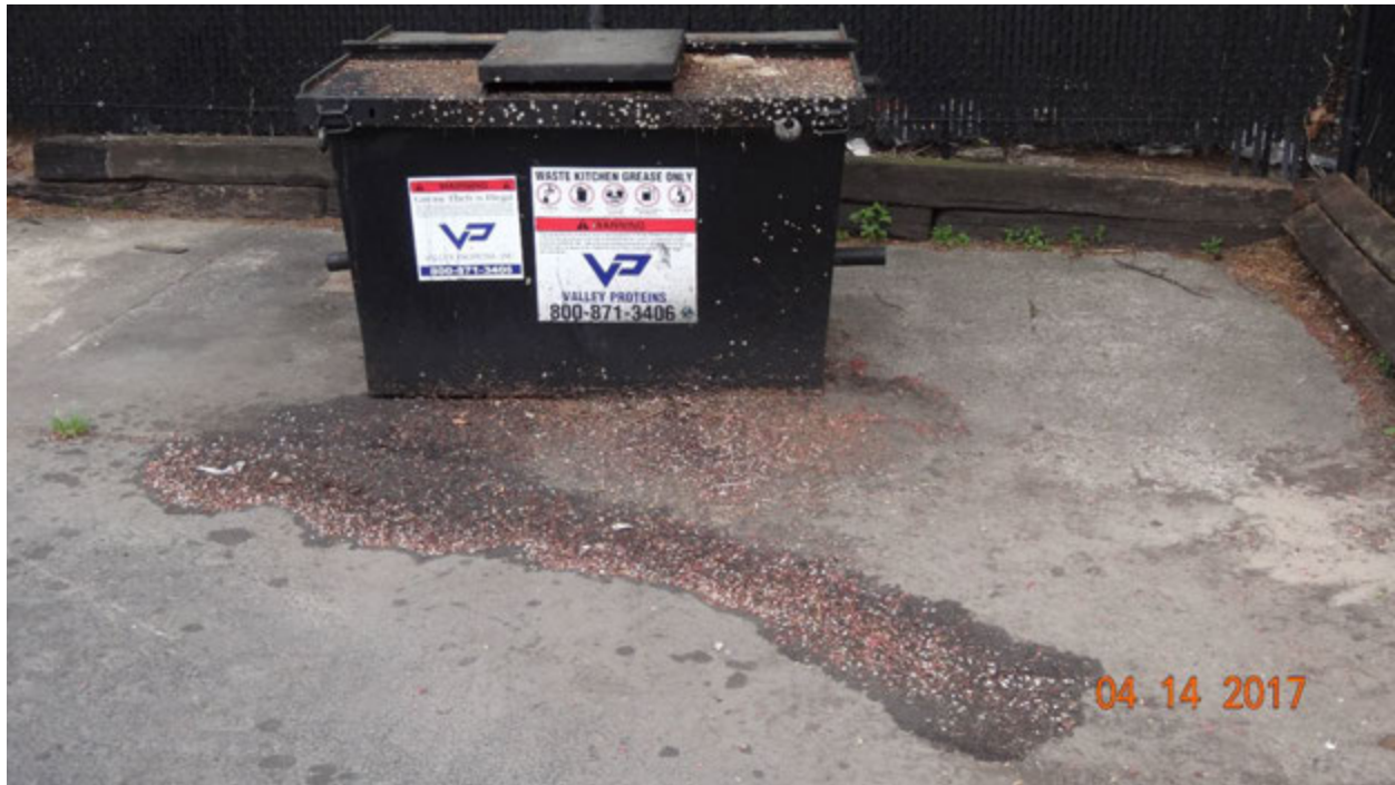
Figure 2. Evidence of a leak or a spill distributing waste grease to the pavement adjacent to the container
