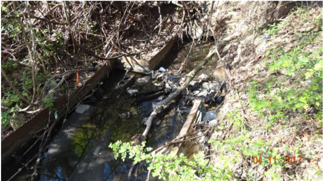
Figure 1. An apparently fortified channel with plywood decking forming part of the sides (left)
