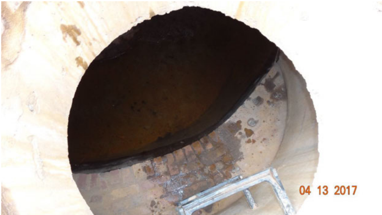
Figure 3. View inside the fourth manhole
