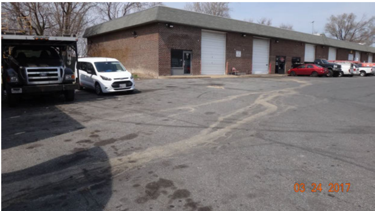
Figure 6. Evidence of runoff from a previous washdown activity that carried sediment; the grate inlet receiving this runoff is at the southwest corner of the lot (off the left side of the photograph)
