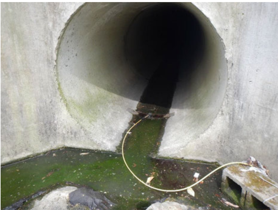
Figure 2. View of the flowing effluent at outfall R20B5O005 (the secured wire and sensor were part of the apparatus in place for a different study); note the signs of green algae in the pipe and the plunge pool
