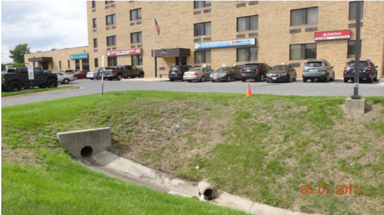
Figure 2. View of the channel in front of the building at 200 Hospital Drive; note the small pipe entering the channel at an angle from the direction of the building (outfall M08E8O003 is seen to the left)
