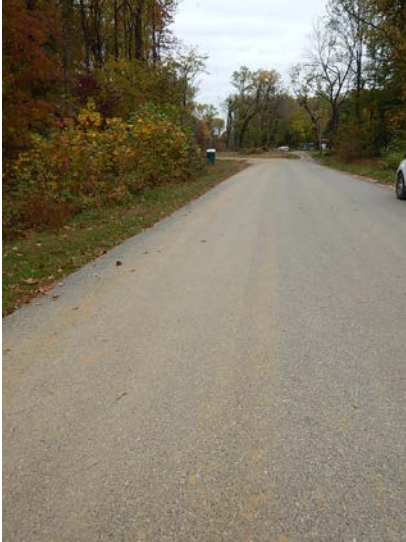
SCE required maintenance; tracking on roadway
