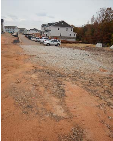
SCE was being short-circuited; maintenance required
