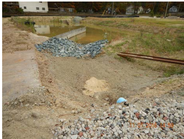
Install outlet protection for culvert
