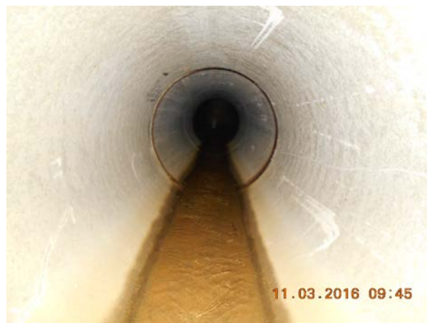
Sediment observed leaving site from sediment basin
