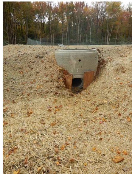
Modified dike discharges to concrete structure
