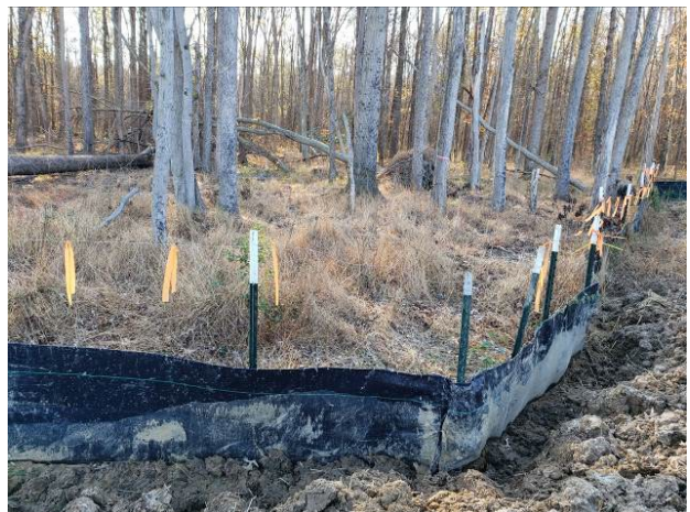
Repaired RSF (County submitted 11/19/2022)
