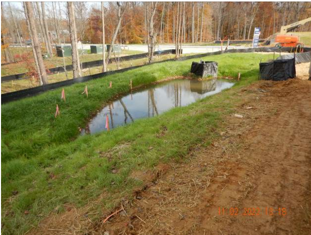
Unstabilized area above micro-bioretention
