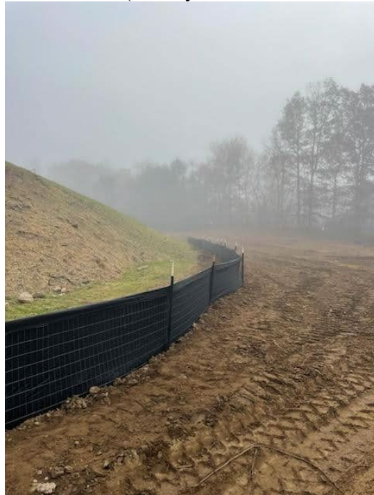
Installed RSF (County submitted 11/15/2022)
