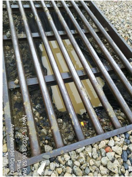
Cleaned out wash rack (County submitted 11/15/2022)
