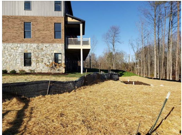
Stabilized area (County submitted 11/15/2022)
