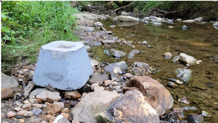
Figure 3: Sediment trap design. Top: schematic representation of the sediment trap in stormflow conditions. Bottom: picture of sediment trap in stream during baseflow conditions.
