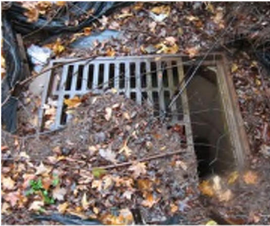
Damaged Grate
