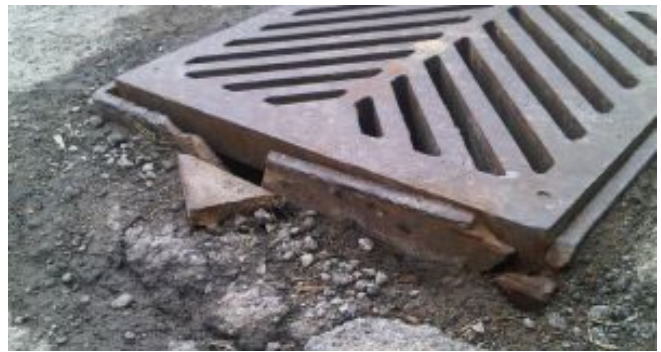
Damaged Frame
