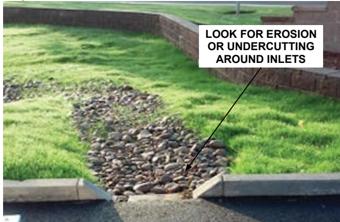
Inlet to a rock-lined swale.
