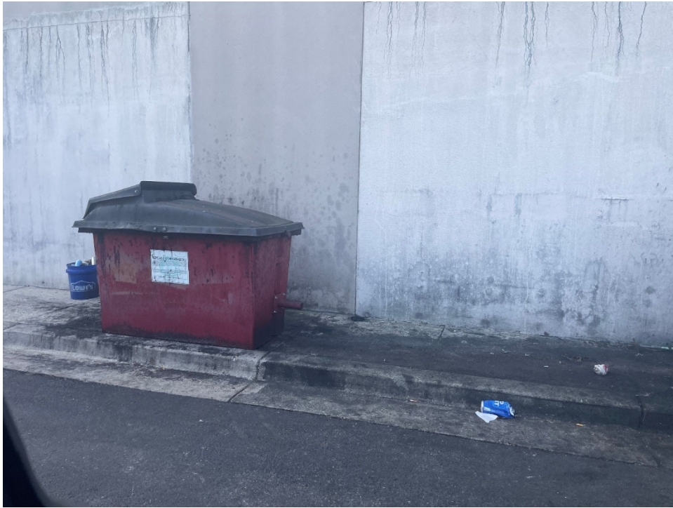
2/8/2024 Inspection – Grease staining on grease bins and pavement.
