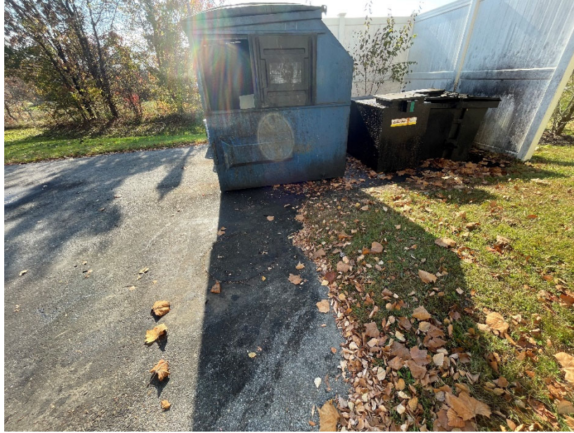
11/9/2023 Inspection – Dumpster containment, pavement stains.
