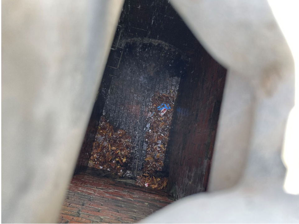
11/30/2023 Inspection – Inlet interior.
