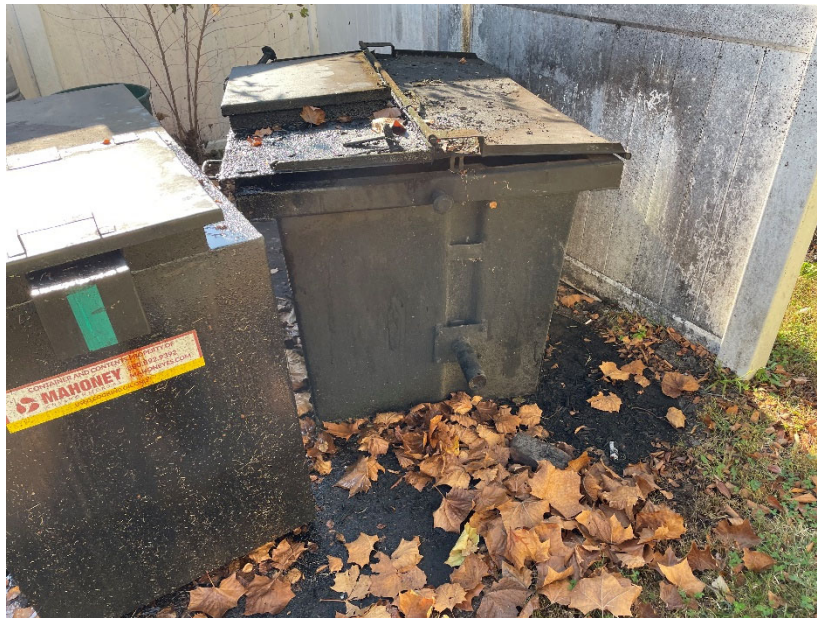
11/9/2023 Inspection – Grease spill and staining from past spills.
