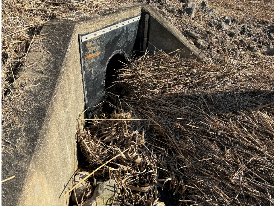
02/09/2024 Inspection – Upstream side of N05G3000001 sample point.
