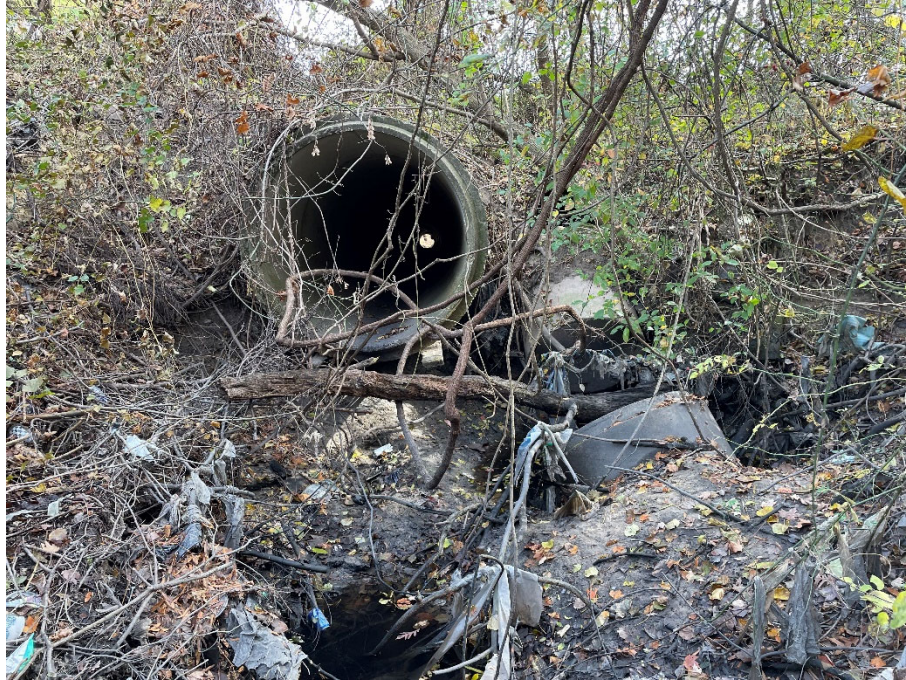
11/15/2023 Inspection – Overview of culvert (left) and Outfall M11A3000001 (right).
