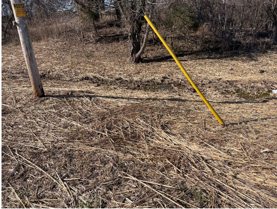
02/09/2024 Inspection – Swale at Northern Recycling Center.
