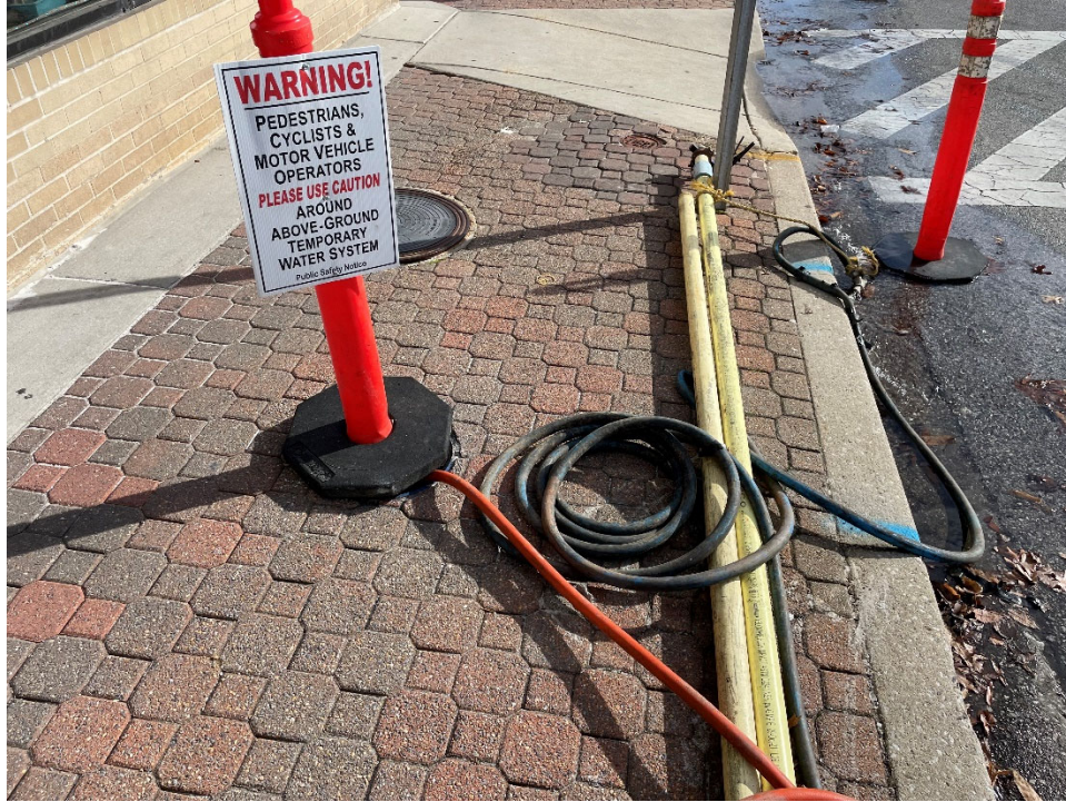
11/30/2023 Inspection – Water line meter connection.
