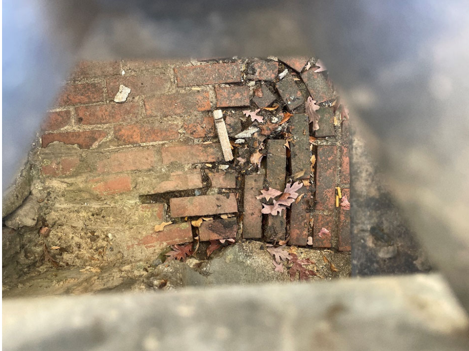
Inside next upstream inlet from manhole on 11/16/23.
