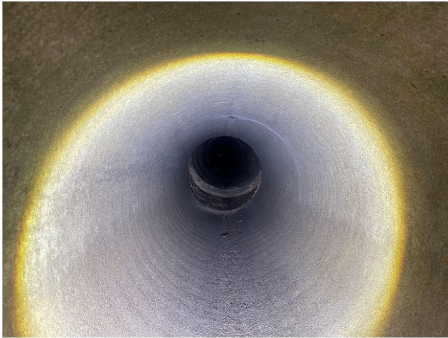
12/01/2023 Inspection – Outfall N04E7O00008 barrel.
