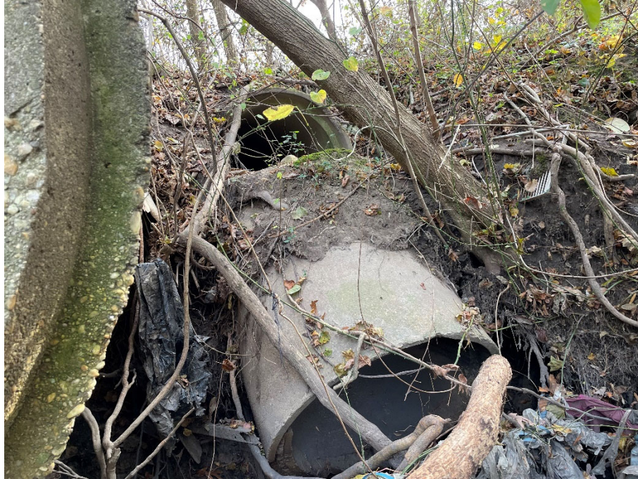
11/15/2023 Inspection – Outfall M11A3O00001 overview.
