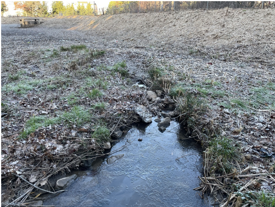
Outfall B11G7O00012 downstream.
