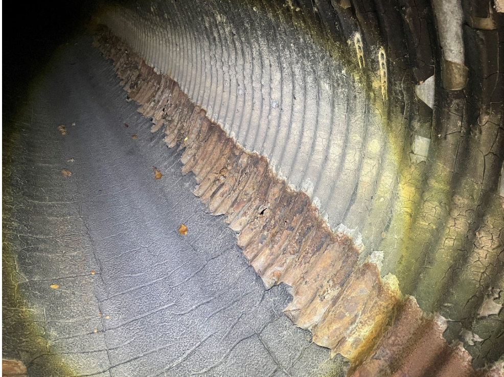
11/15/2023 Inspection – Outfall M08C8O00011 barrel pipe.
