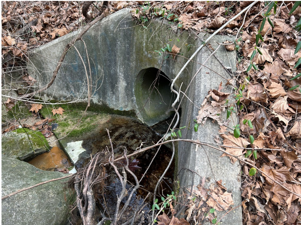
2/8/2024 Inspection – Overview of N07G8O00030.
