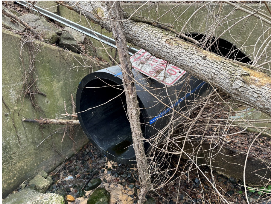
02/09/2024 Inspection – Overview of N05G3000001 sample point.
