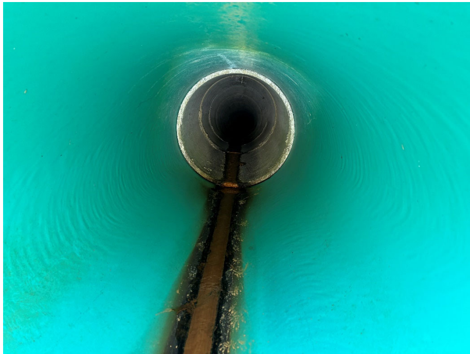
02/09/2024 Inspection – O04A8O00001 inside pipe.
