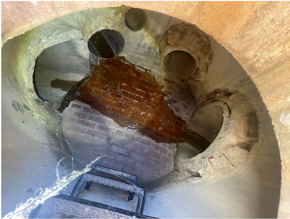
Inside manhole upstream from Outfall M08C8O00003 on 11/16/23.
