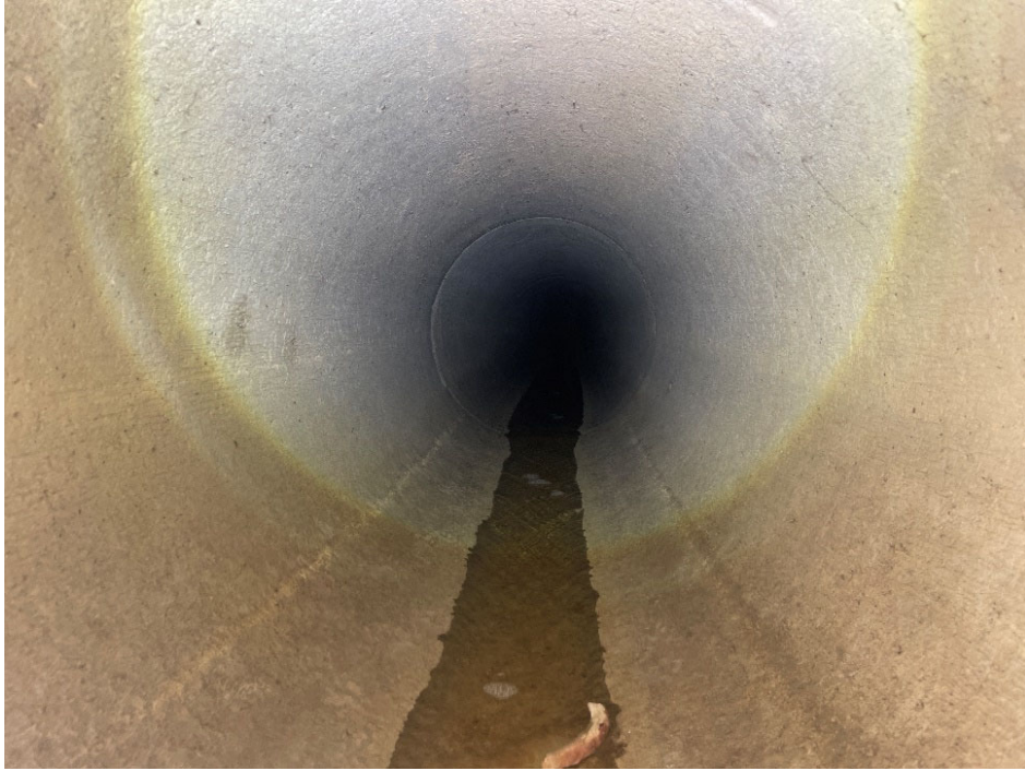
Inside Outfall M08C8O00003 pipe on 11/16/23.
