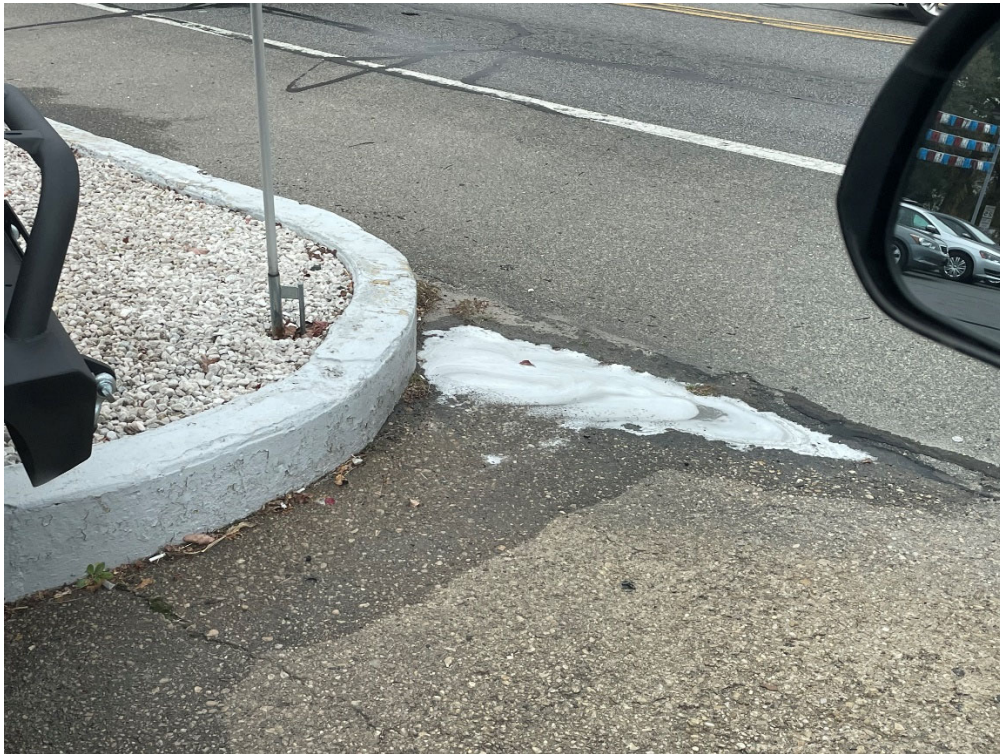
11/7/2023 Inspection – Soapy water running off into MD 177.
