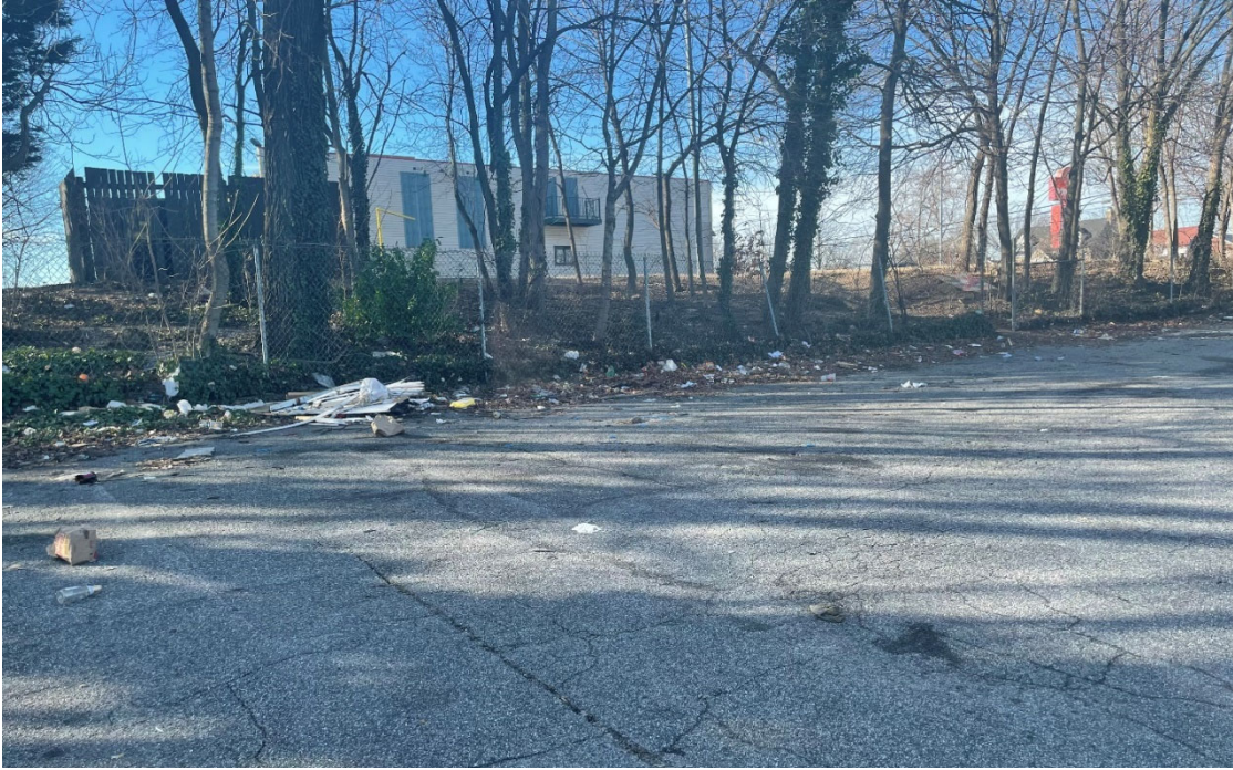
2/8/2024 Inspection – Public dumping along fence line of parking lot.
