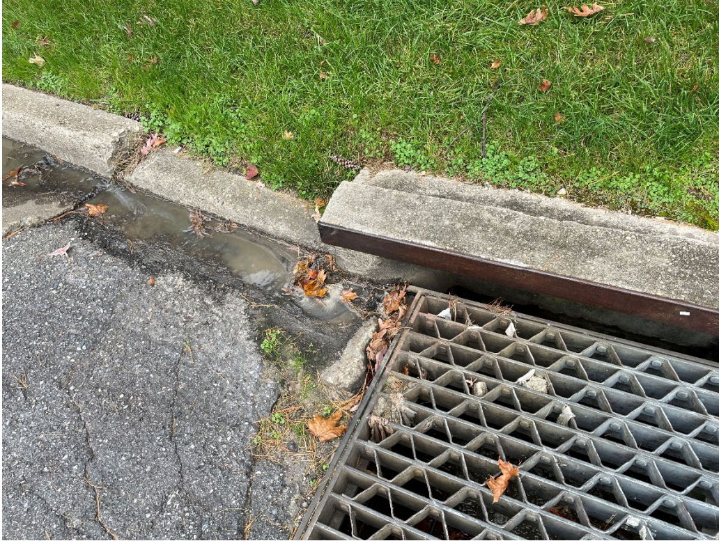
11/7/2023 Inspection – Greasy wash water entering storm drain.
