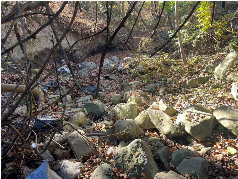
11/15/2023 Inspection – Outfall M08C8O00011 downstream.
