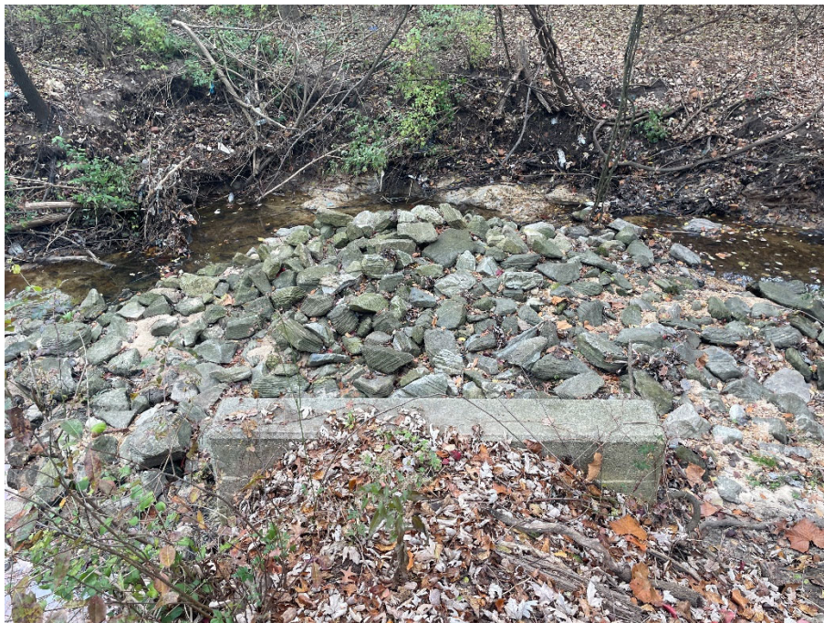
12/01/2023 Inspection – Outfall N04E7O00008 downstream.
