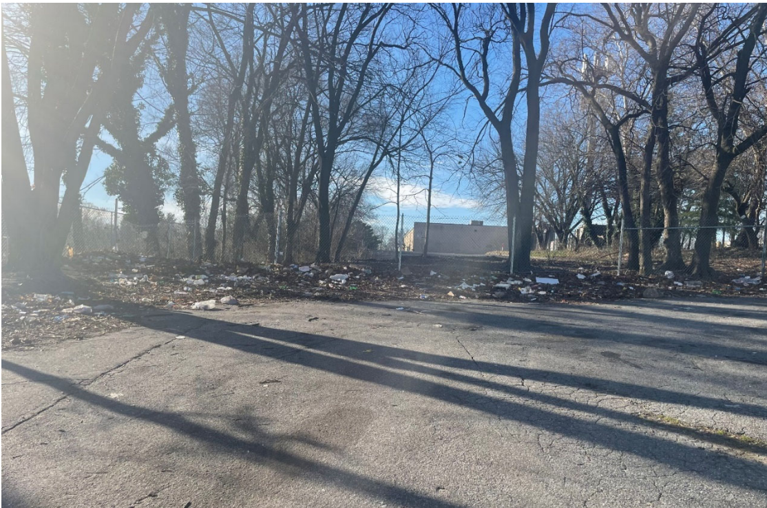
2/8/2024 Inspection – Public dumping along fence line of parking lot
