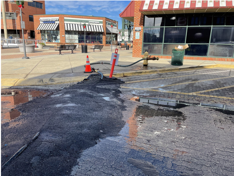
11/30/2023 Inspection – Fire hydrant connection.
