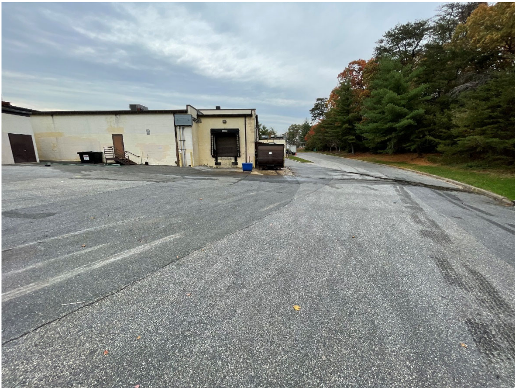
11/7/2023 Inspection – Overview of area.
