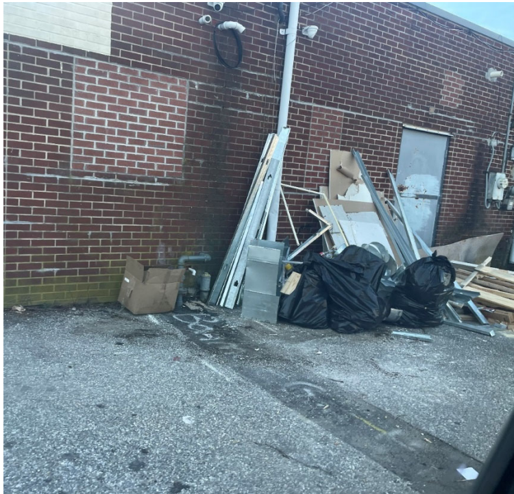
2/8/2024 Inspection – Trash and building material debris behind Village Liquors.
