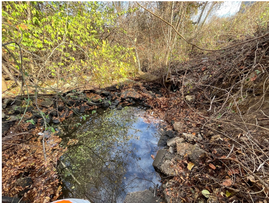
11/30/2023 Inspection – Downstream of Outfall M06C1000001.
