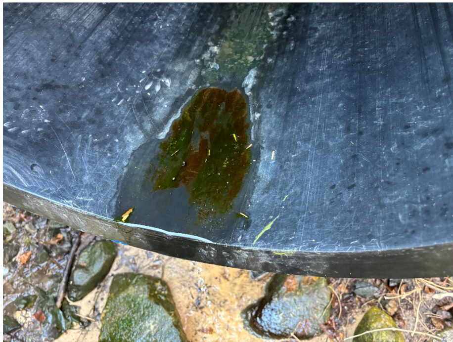
02/09/2024 Inspection –N05G3000001 sample point close-up.
