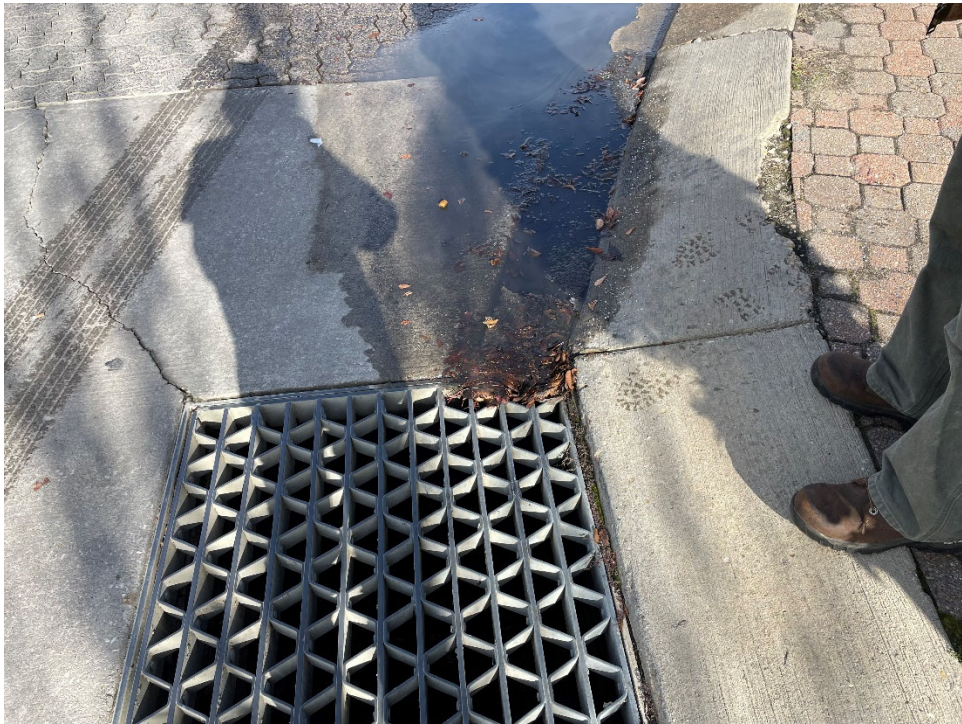
11/30/2023 Inspection – Water draining into inlet.
