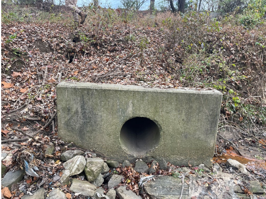
12/01/2023 Inspection – Outfall N04E7O00008 overview.
