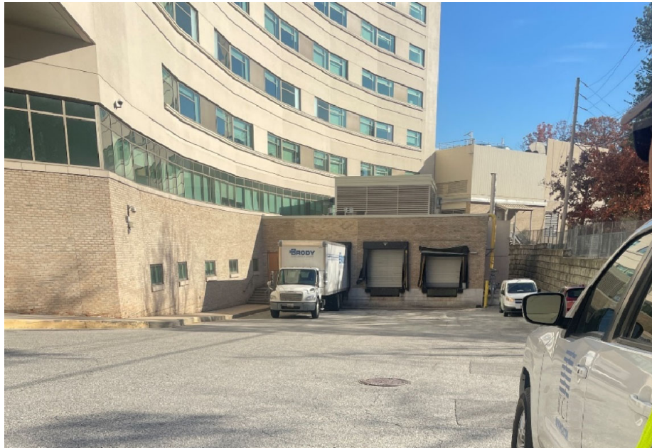
Overview of flow source area on 11/16/23.
