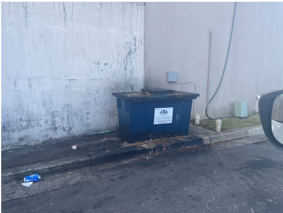
2/8/2024 Inspection – Grease staining on pavement and grease on top of bin.
