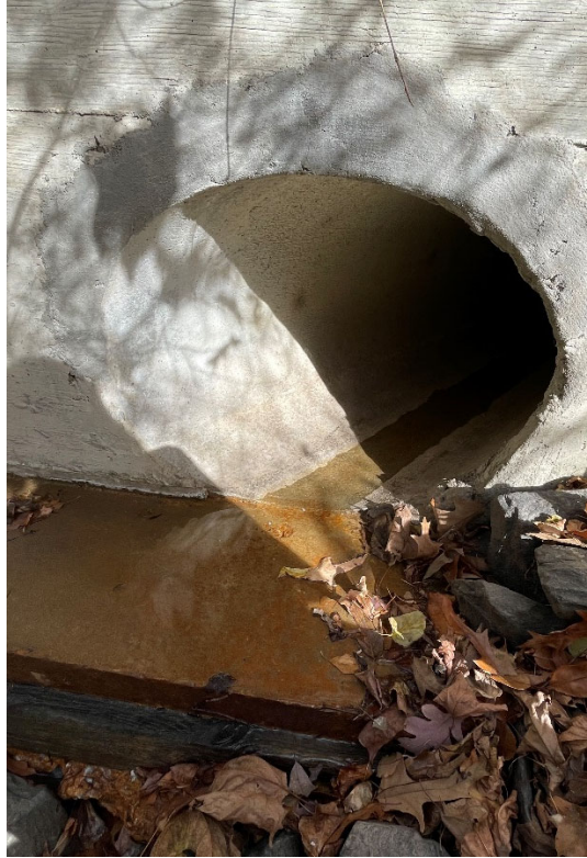
Outfall M08C8O00003 on 11/20/23 (1 st inspection).
