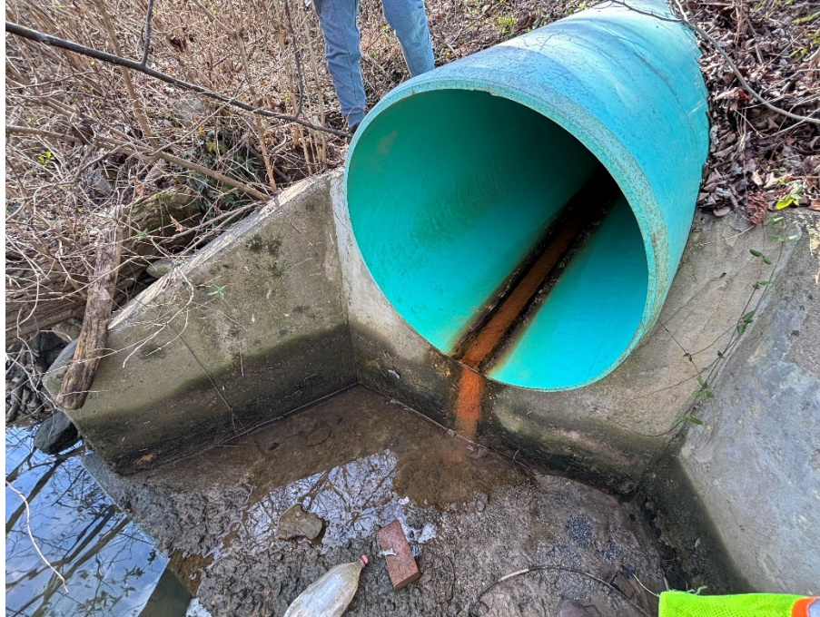
02/09/2024 Inspection – Overview of O04A8O00001.
