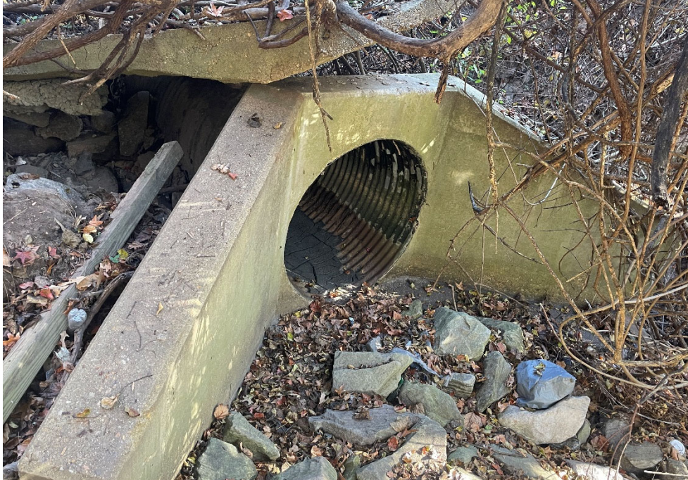
11/16/2023 Inspection – Overview of Outfall M08C8O00011.
