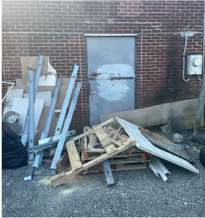
2/8/2024 Inspection – Trash and building material debris behind Village Liquors.
