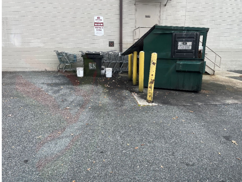
11/7/2023 Inspection – Grease bin and staining.
