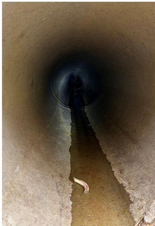
Inside Outfall M08C8O00003 pipe on 11/17/23.
