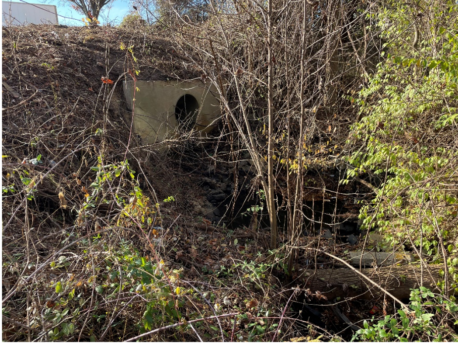
11/30/2023 Inspection – Overview of M06C1000001.
