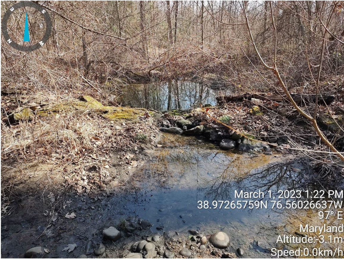
Step pool conveyance facing southwest along the channel. Area appears stable with no signs of erosion.
