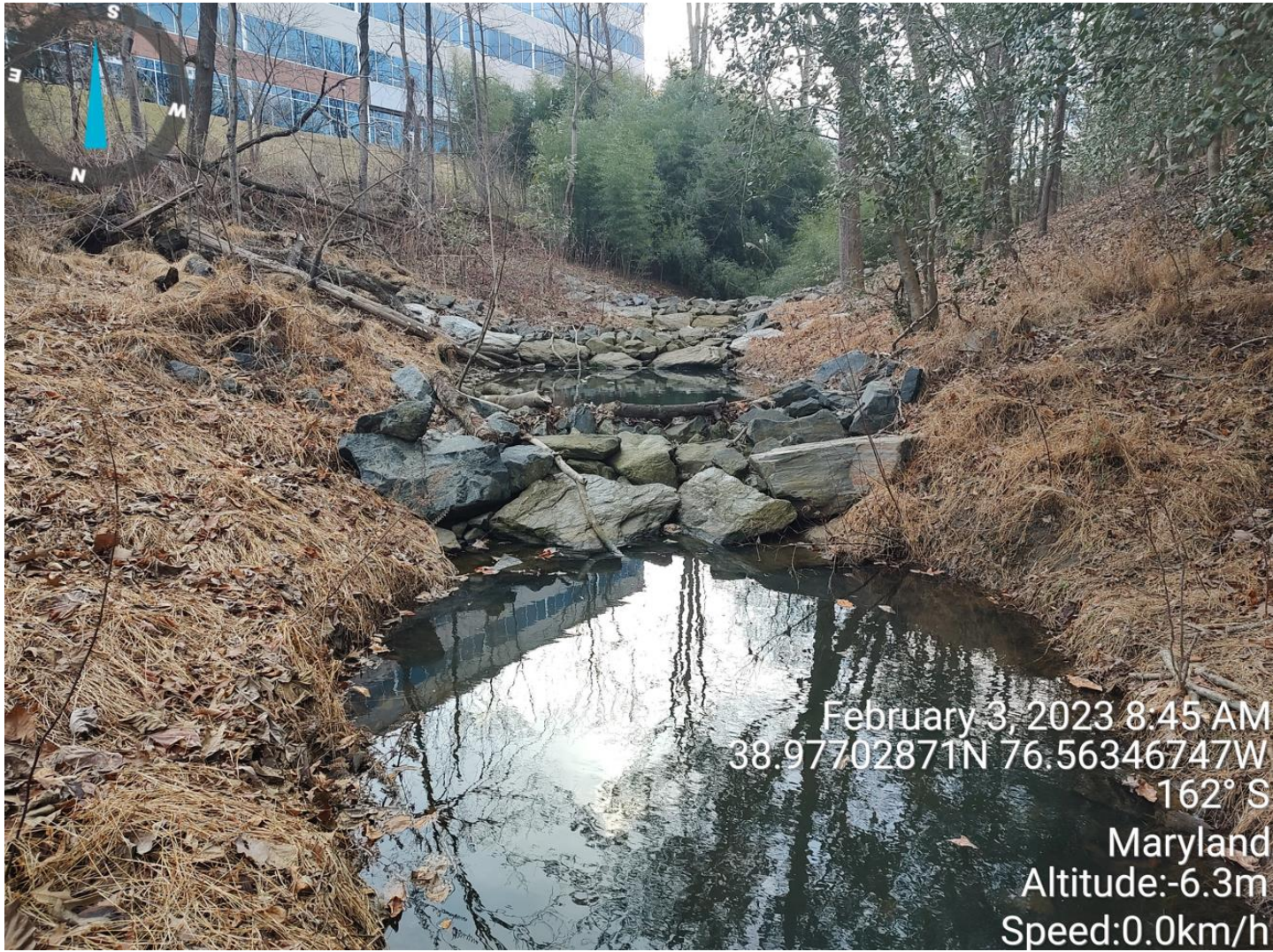
Upstream view of Broad Creek with step pools and check dams shown. This is located near the hypothetical POI
