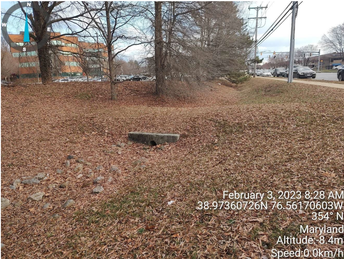
View of the roadside swell with a culvert along Riva Road, adjacent to the Project property. The area appears stable. No erosion is present.
