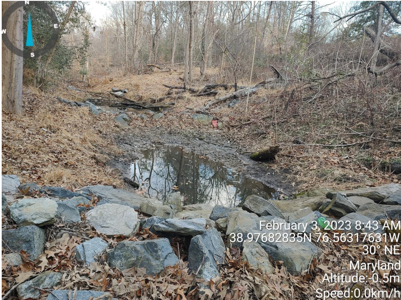
Downstream View of Broad Creek; Check dam and step pool can be seen in picture
