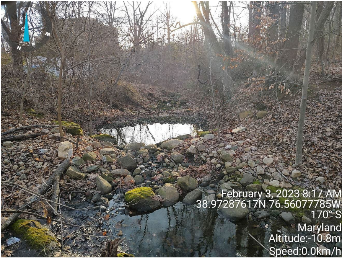
Step pool conveyance facing south along the channel. Area appears stable with no signs of erosion.
