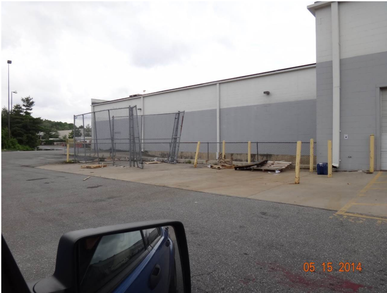
Figure 2. Scattered and broken pallets and loose cardboard found behind the building
