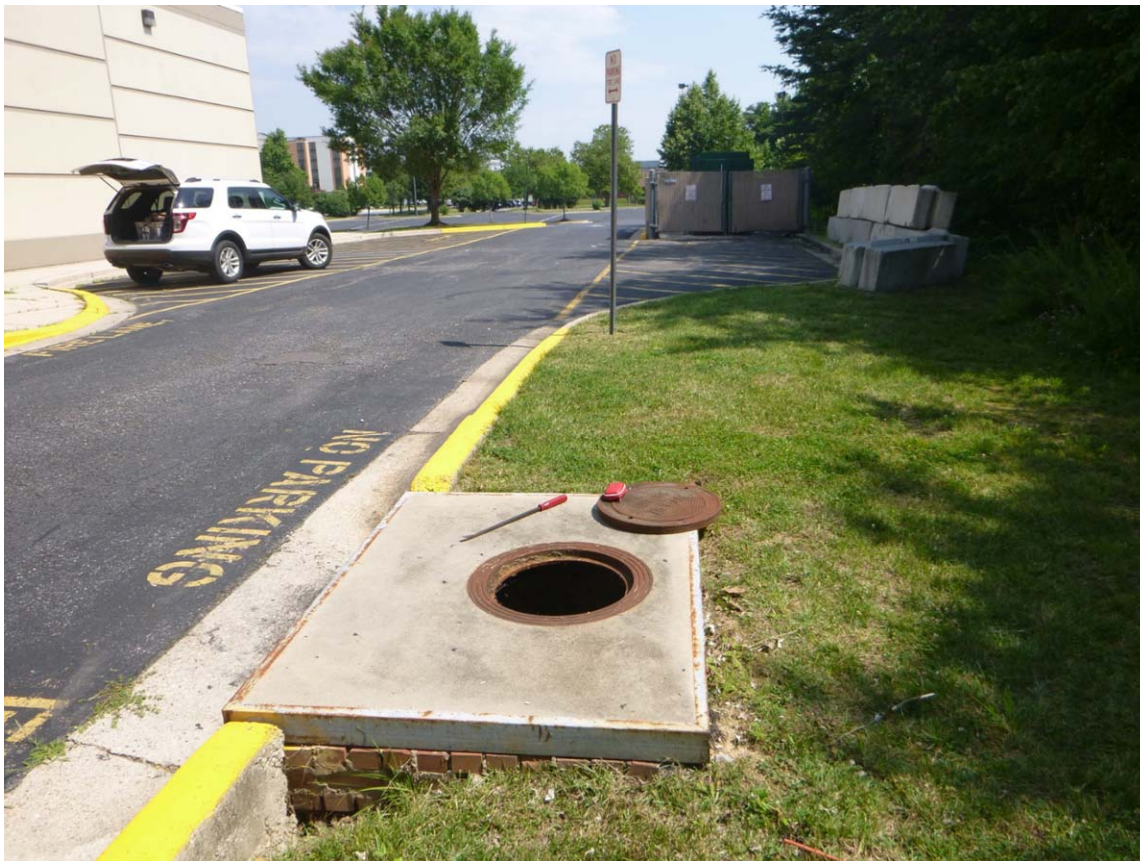
Figure 1. Curb inlet with manhole cover removed; dumpsters in the background are slightly up-grade to the inlet
