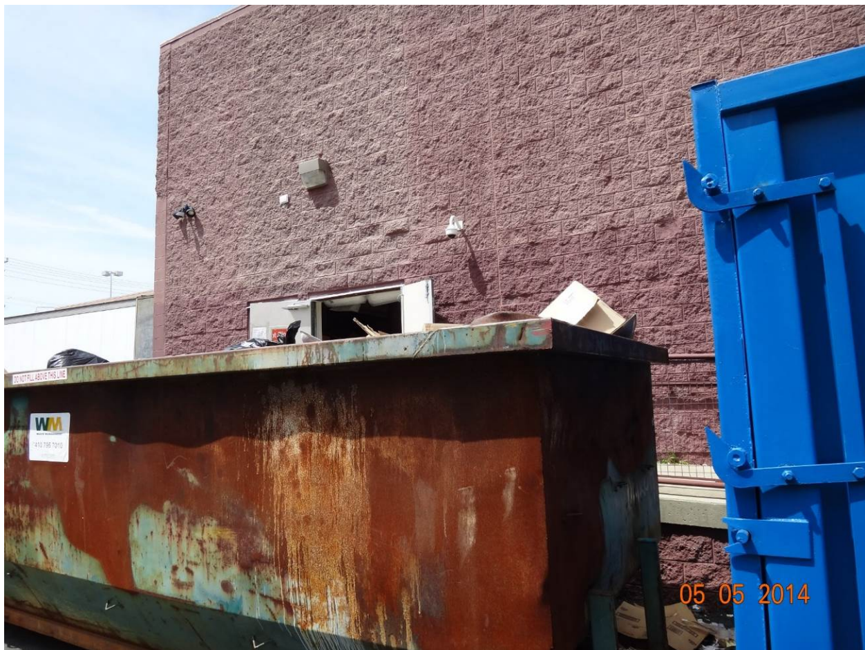
Figure 1. Full roll-off dumpster alongside the Target building
