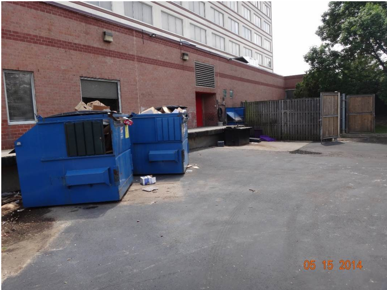
Figure 5. Overflowing dumpsters, behind 1300 Concourse Drive
