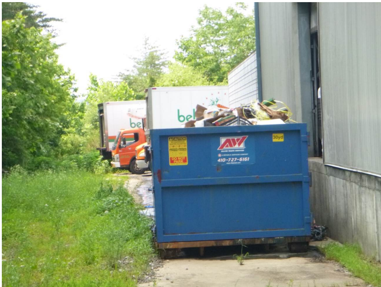
Figure 1. Roll-away dumpster found behind the Belair Produce building actively leaking fluid
