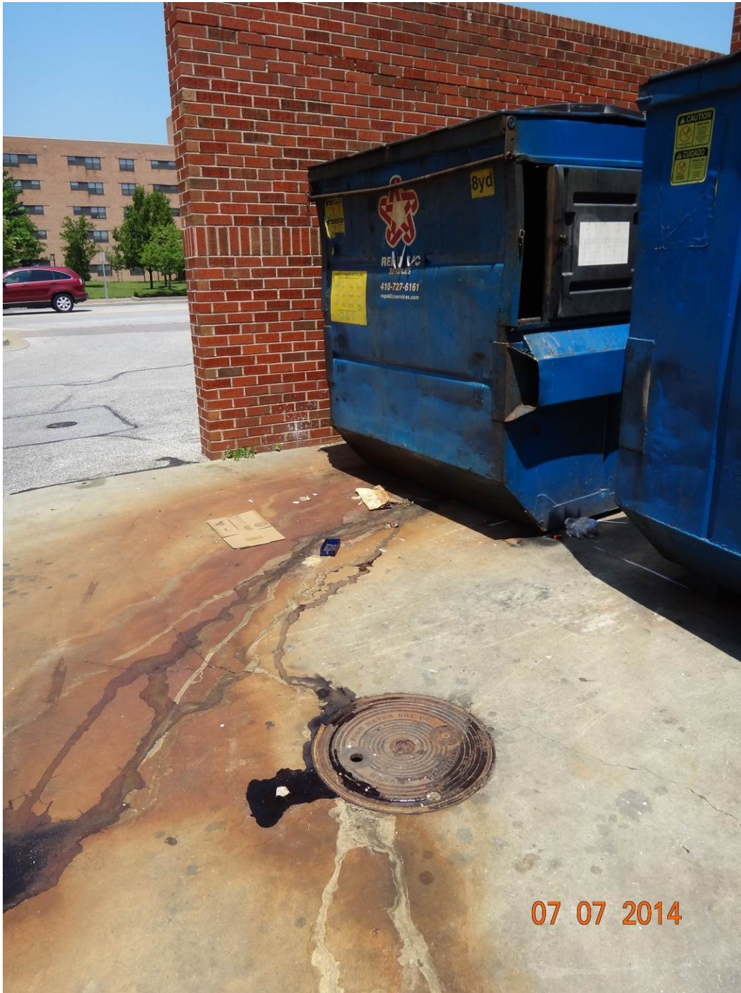
Figure 2. Evidence of liquid leaking from dumpsters
