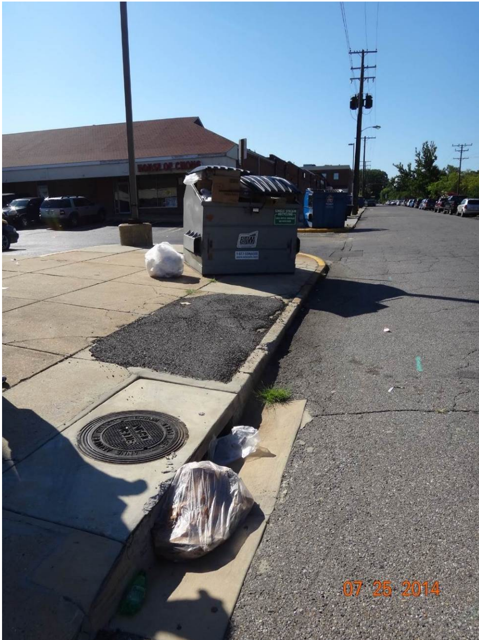
Figure 1. Debris observed alongside the dumpster and blocking the storm drain inlet
