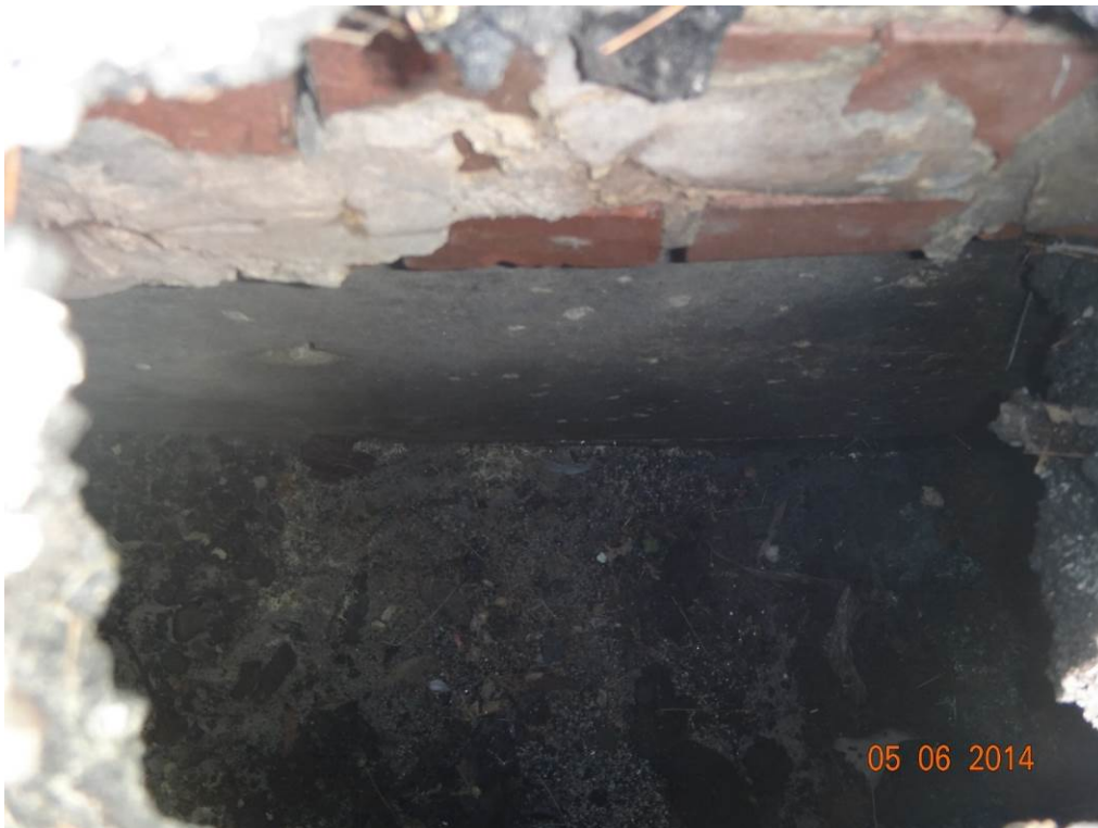
Figure 3. Interior of catch basin as viewed through the hole
