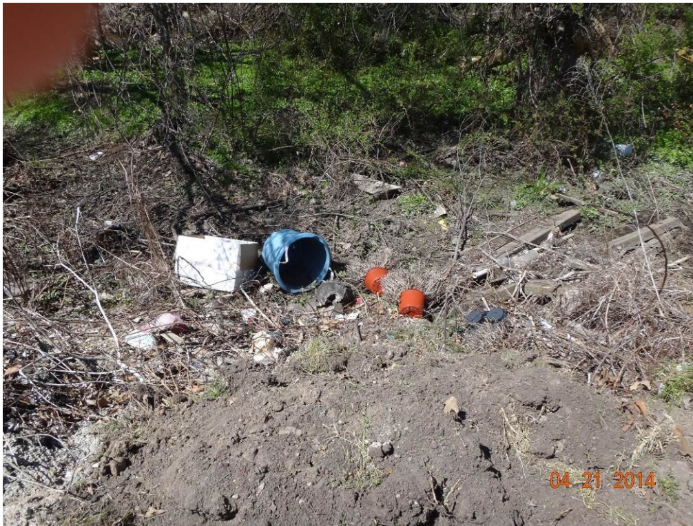
Figure 1. Dumping area in floodplain of Sawmill Branch
