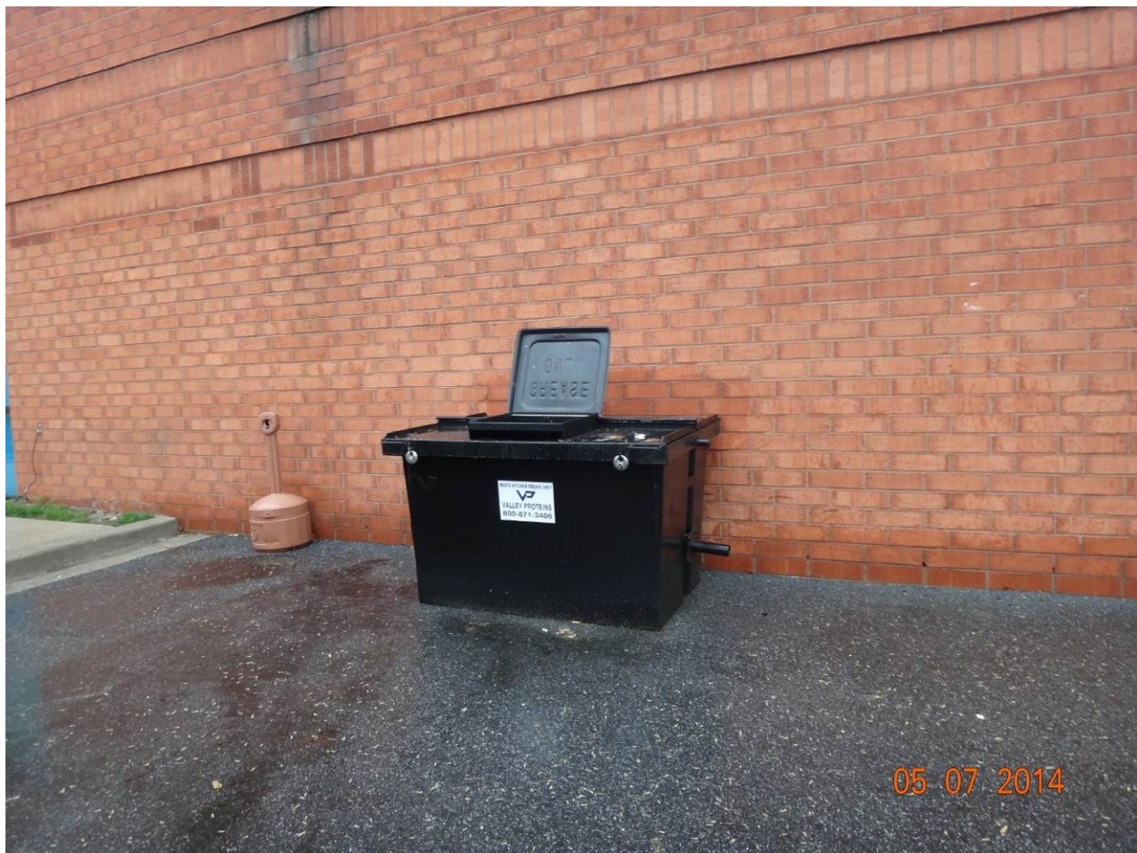
Figure 1. Open waste grease disposal container
