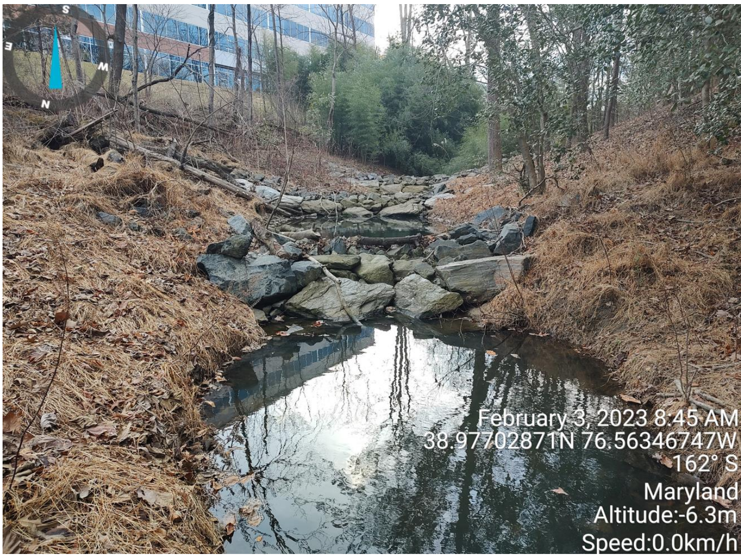
Upstream view of Broad Creek with step pools and check dams shown. This is located near the hypothetical POI
