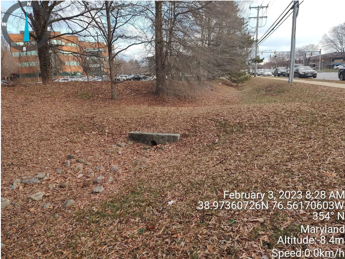
View of the roadside swell with a culvert along Riva Road, adjacent to the Project property. The area appears stable. No erosion is present.
