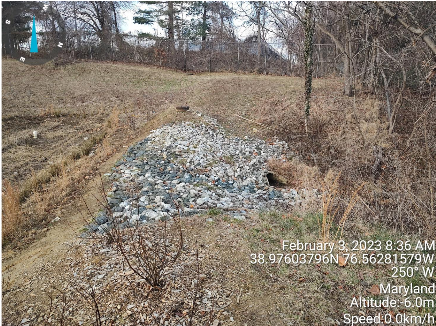
Stones located in stormwater basin
