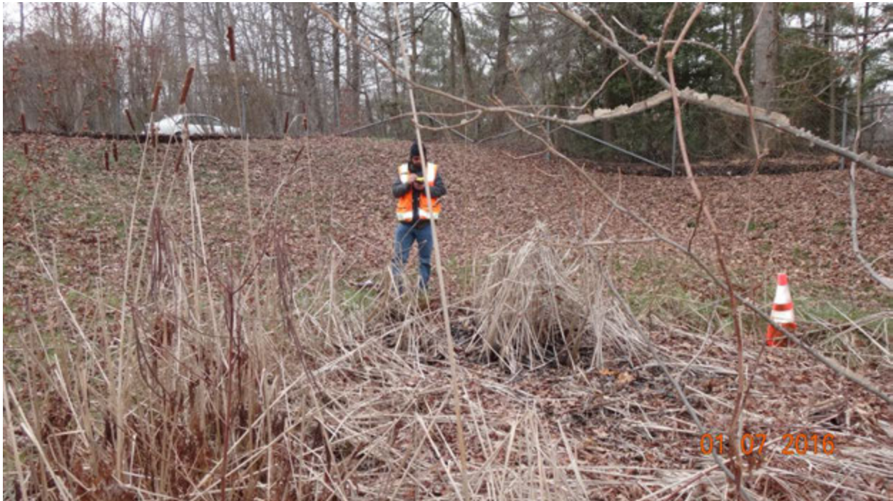
Figure 2. A member of the field team documenting conditions at the outfall which is located directly in front of him; the orange cone is the same marker as is seen in Figure 1
