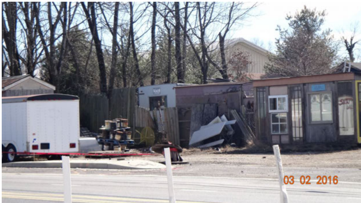
Figure 1. Photograph of some of the conditions in the lots at 2829 and 2827 Jessup Road; note the dilapidated "snowball" building and the discarded furniture
