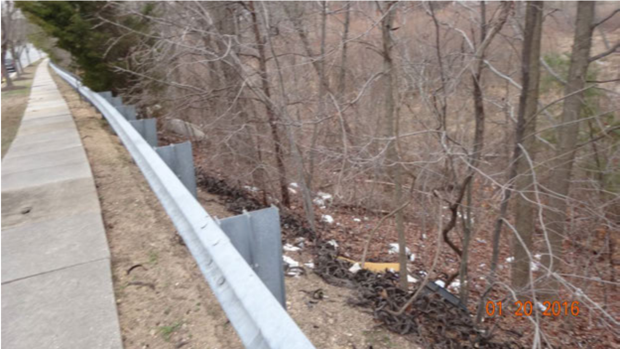
Figure 6. Photograph of some of the extensive debris deposited on the hillsides along the north side of Crossroads Drive; the stream is in the ravine to the right of the view
