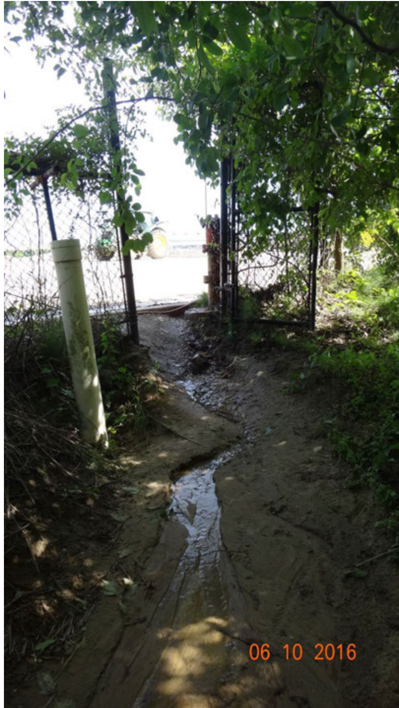
Figure 4. Excess wash water flowing out of a small gate in the fence bordering the race track maintenance area; note the red post hydrant to the right just inside the entrance
