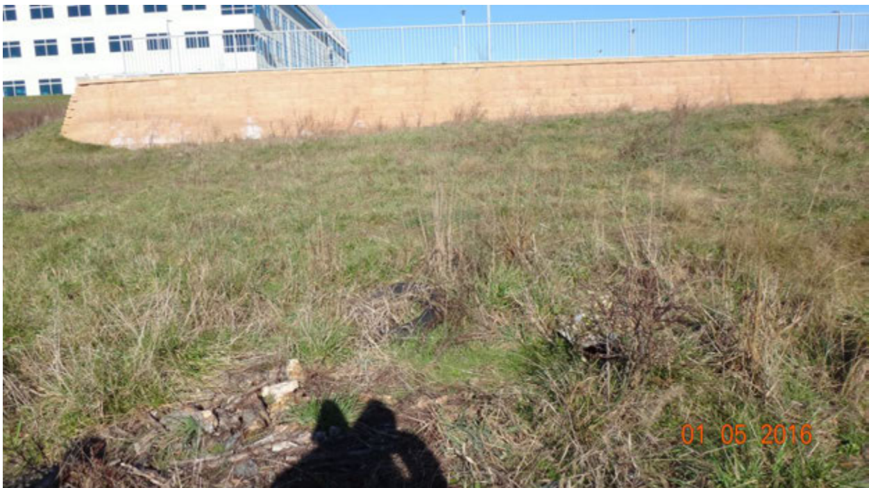
Figure 3. Photograph showing the crushed outfall C10E4O001 (seen as a silver object under vegetation in the lower center right) in context with the new building at 8201 Dorsey Run Road; note the brown vegetation on the upper left of the photograph which indicates the east end of the long drainage ditch behind the three adjacent parking lots
