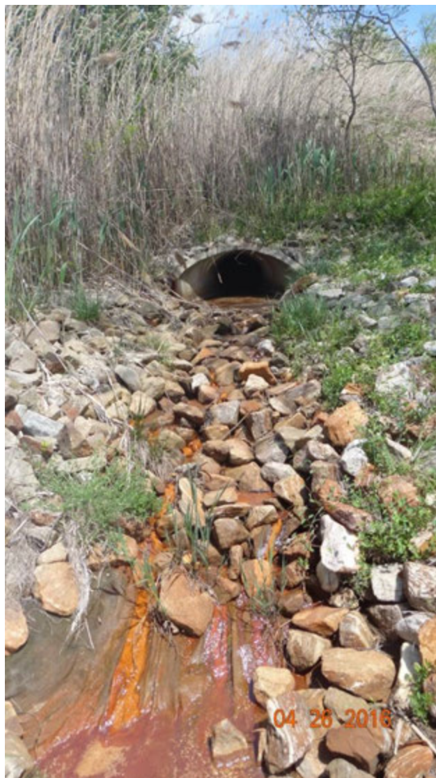
Figure 1. Outfall Q06H3Onew as observed on April 26, 2016; note the orange iron flocculent
