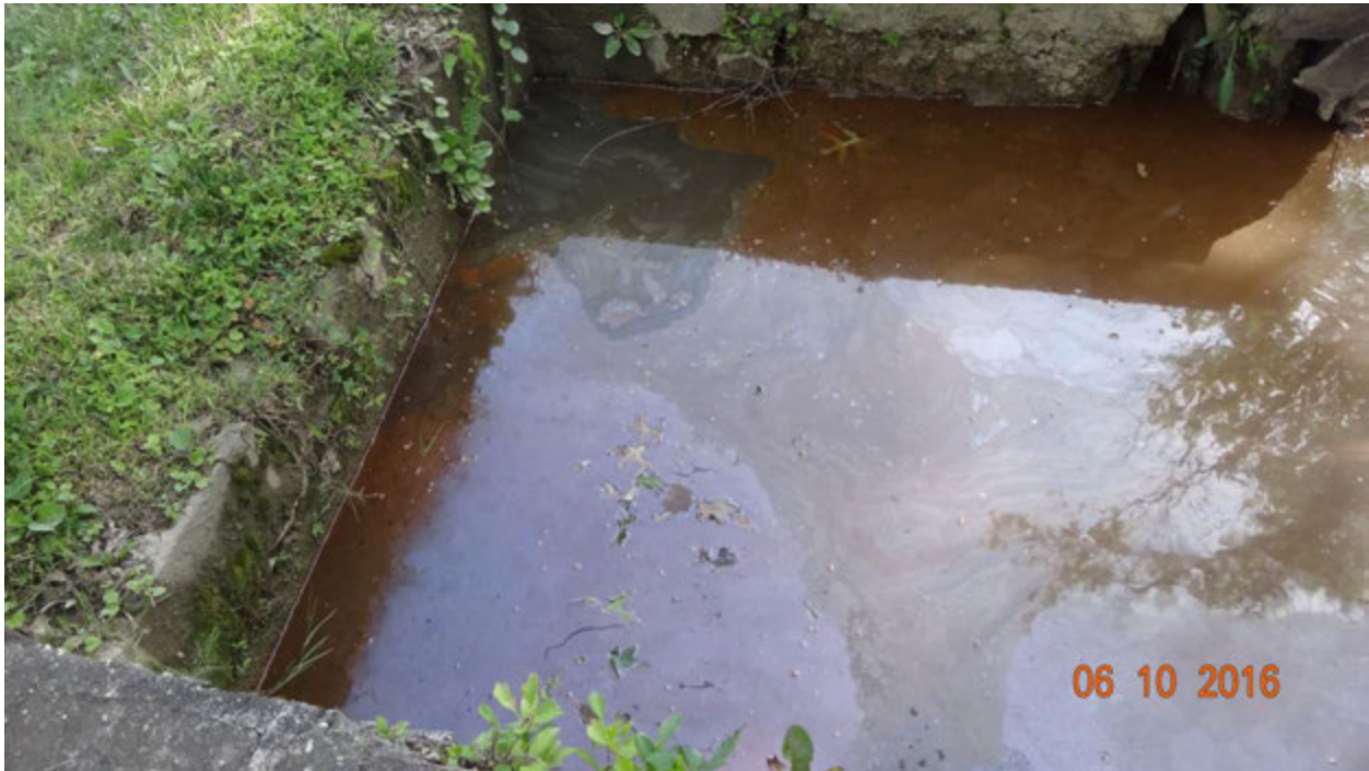
Figure 2. Observed conditions in the pooled water at outfall A11C7O001; note the orange color and the oil sheen
