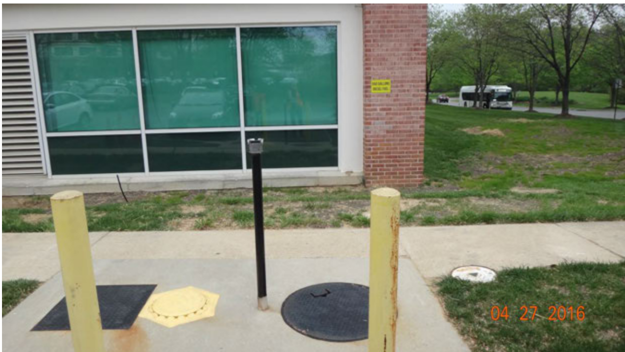
Figure 2. A yellow sign (upper center-right) indicating fuel storage mounted on the building at 1302 Concourse Drive; the sign reads, "550 gallons diesel fuel." Evidence of new grass and loose straw can be seen on the right side of the photograph.
