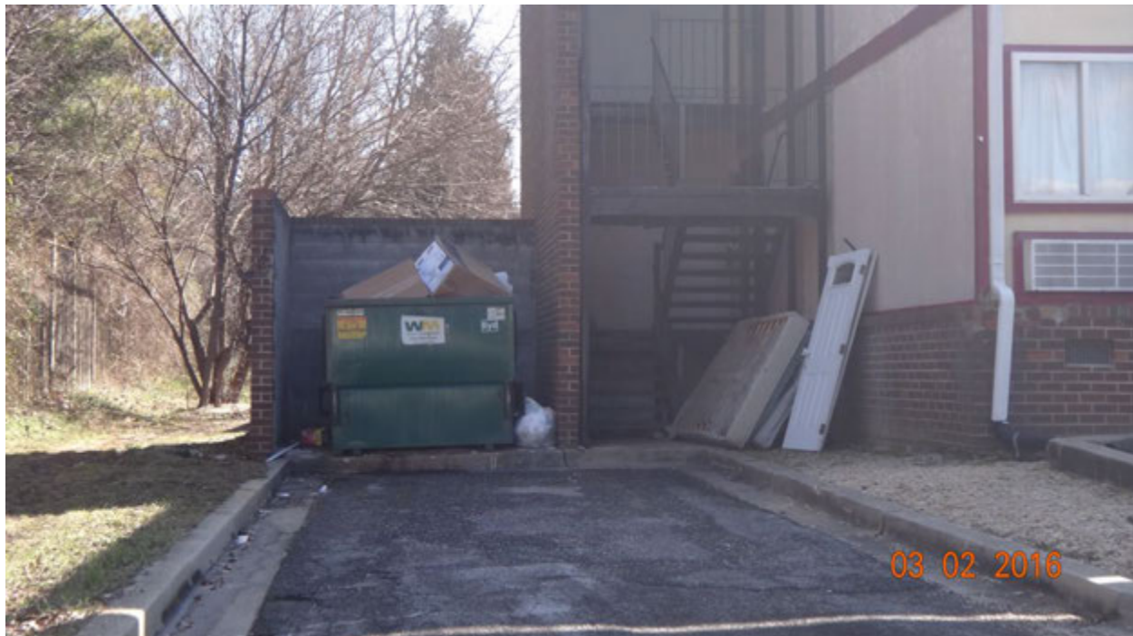
Figure 1. An open, overfilled dumpster with debris scattered around it found near the Red Crown Inn on March 2; note the large debris stored alongside the building, near the stairwell
