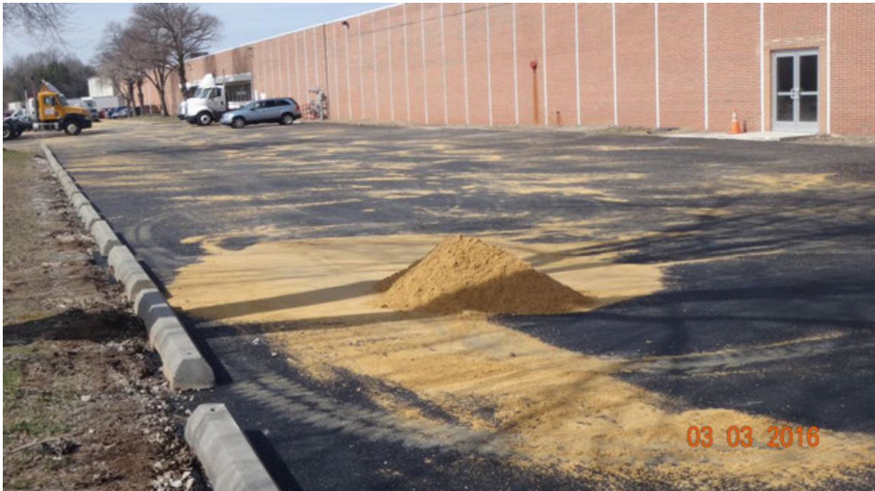
Figure 1. A pile of sand found in the warehouse parking lot on March 3 (foreground); note that the sand had also been distributed throughout the parking lot (background)
