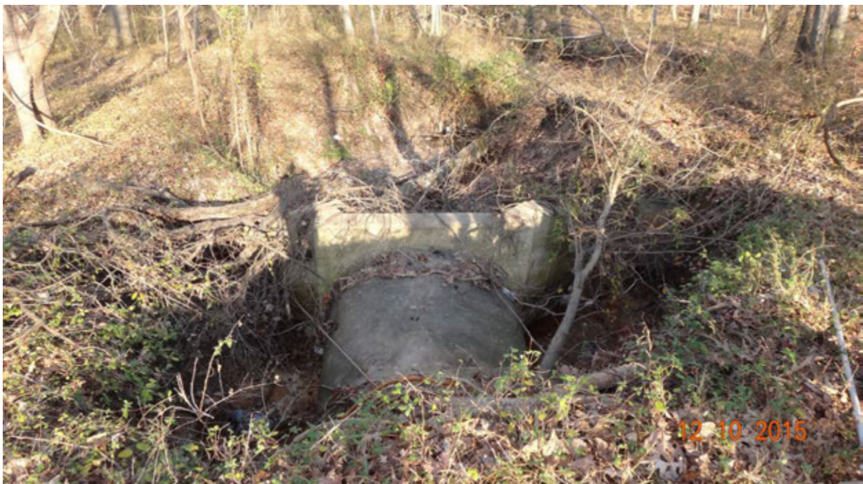
Figure 5. Photograph taken facing approximately northeast (standing over Section 3); note erosion on the bank opposite the End Section
