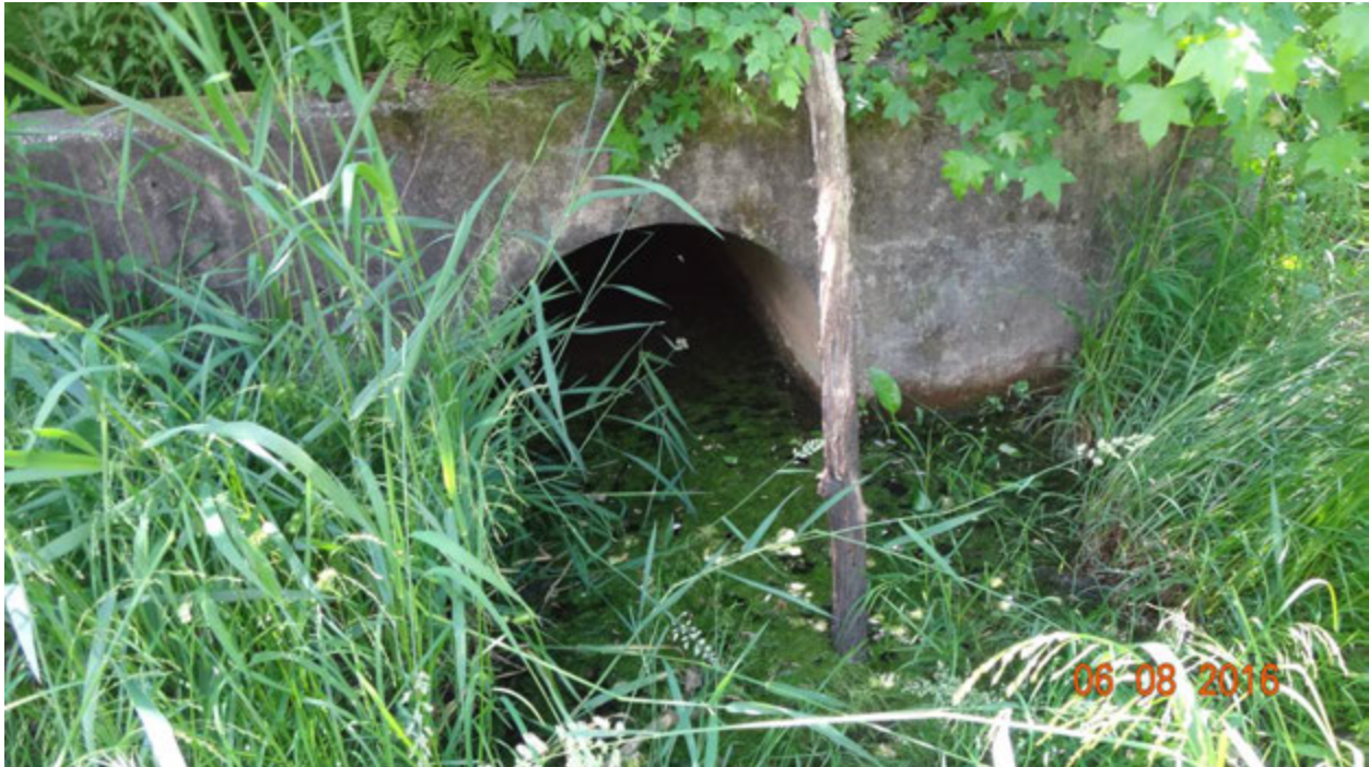
Figure 1. Outfall I12E1O001 as observed on June 8, 2016; note the extensive algae growing in the plunge pool
