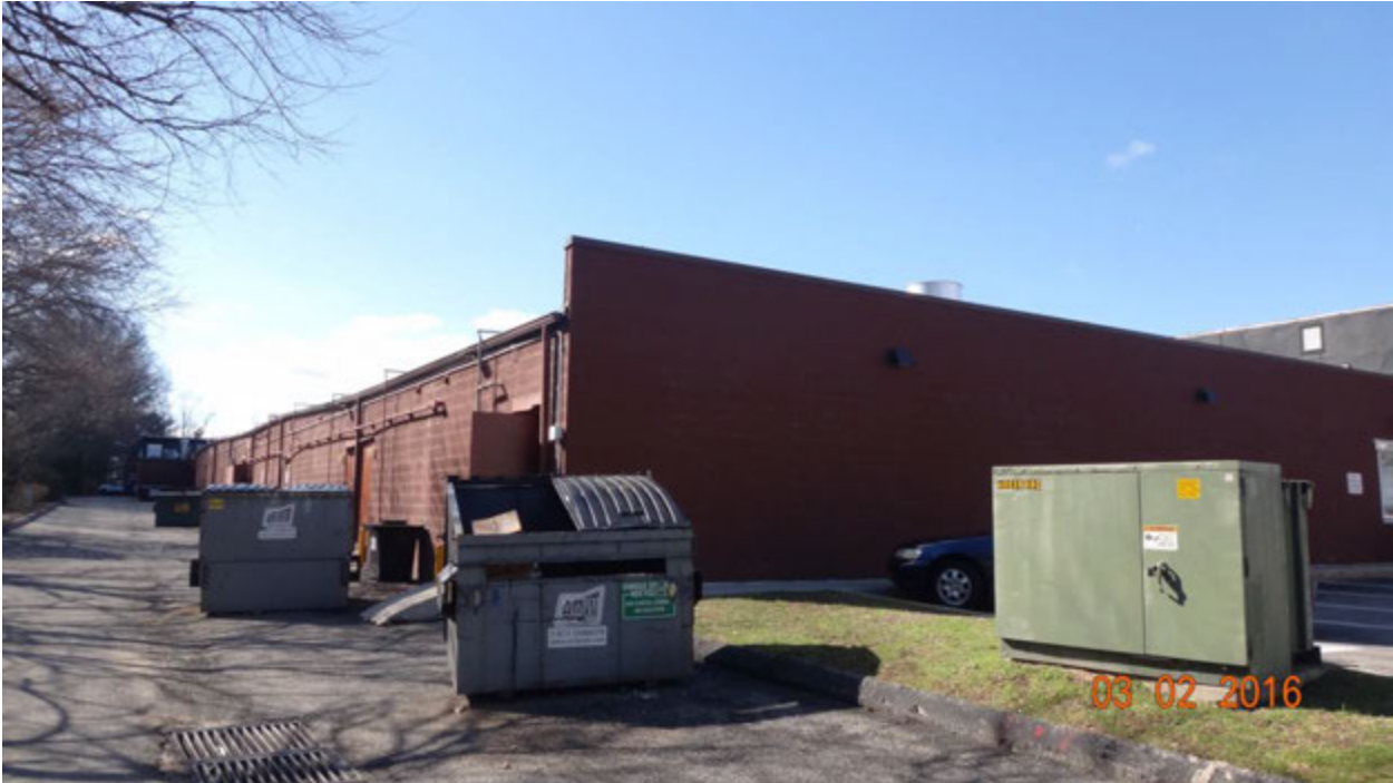
Figure 2. Open dumpster found near storm drain
