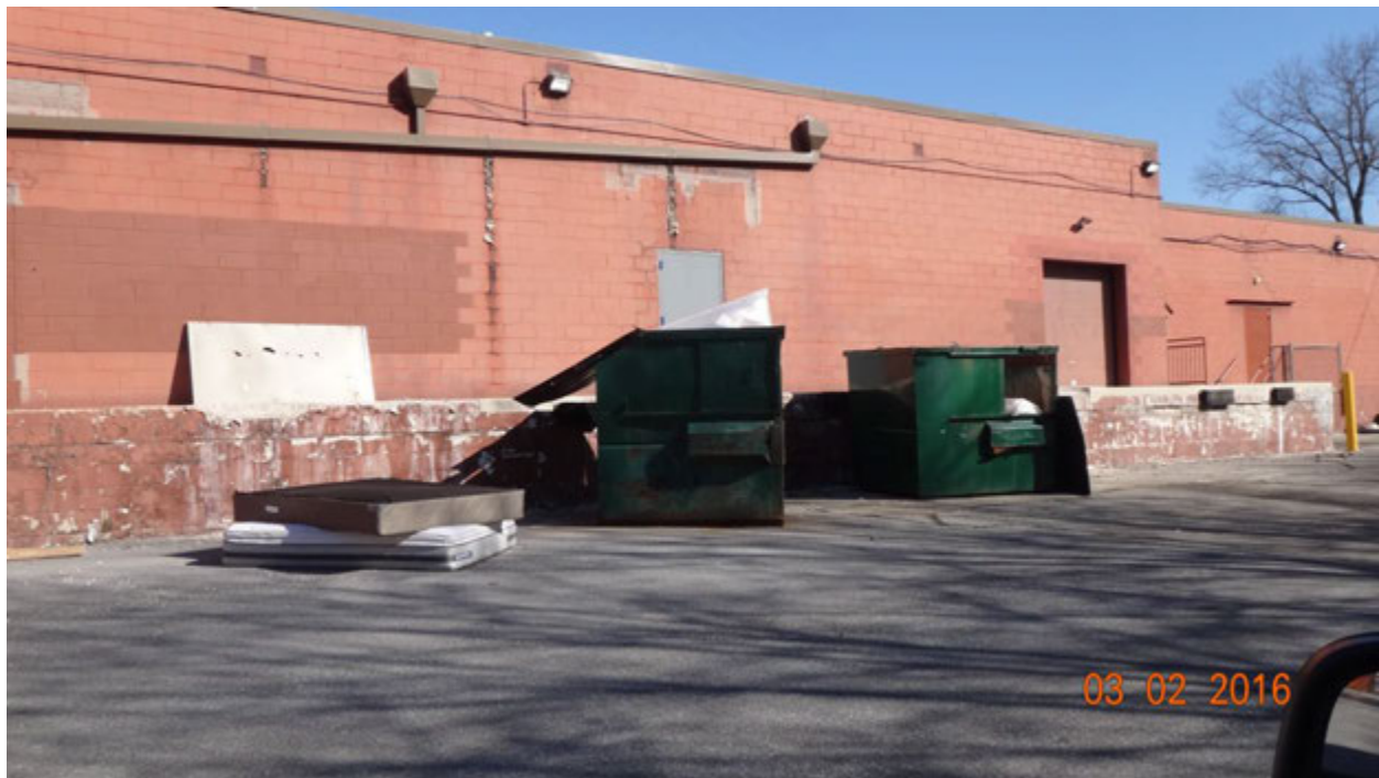
Figure 1. Two open dumpsters with large pieces of debris near them found behind the Aaron's Rentals store
