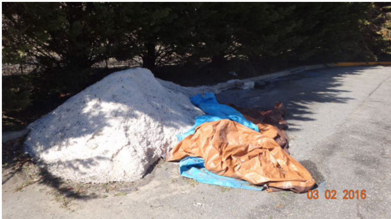
Figure 1. A large, uncovered pile of road de-icing salt found on March 2; the tarps did have weight stones available at the time of the site visit
