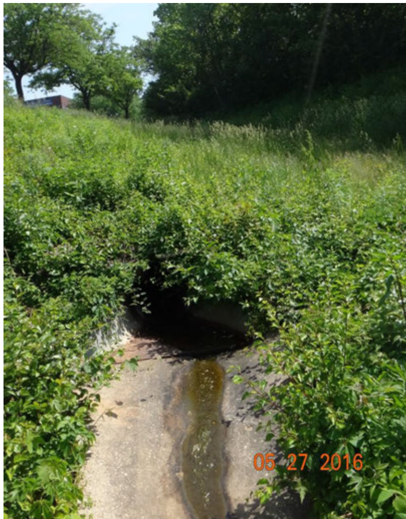
Figure 1. Outfall I04F3O014 with flowing discharge as observed on May 27, 2016
