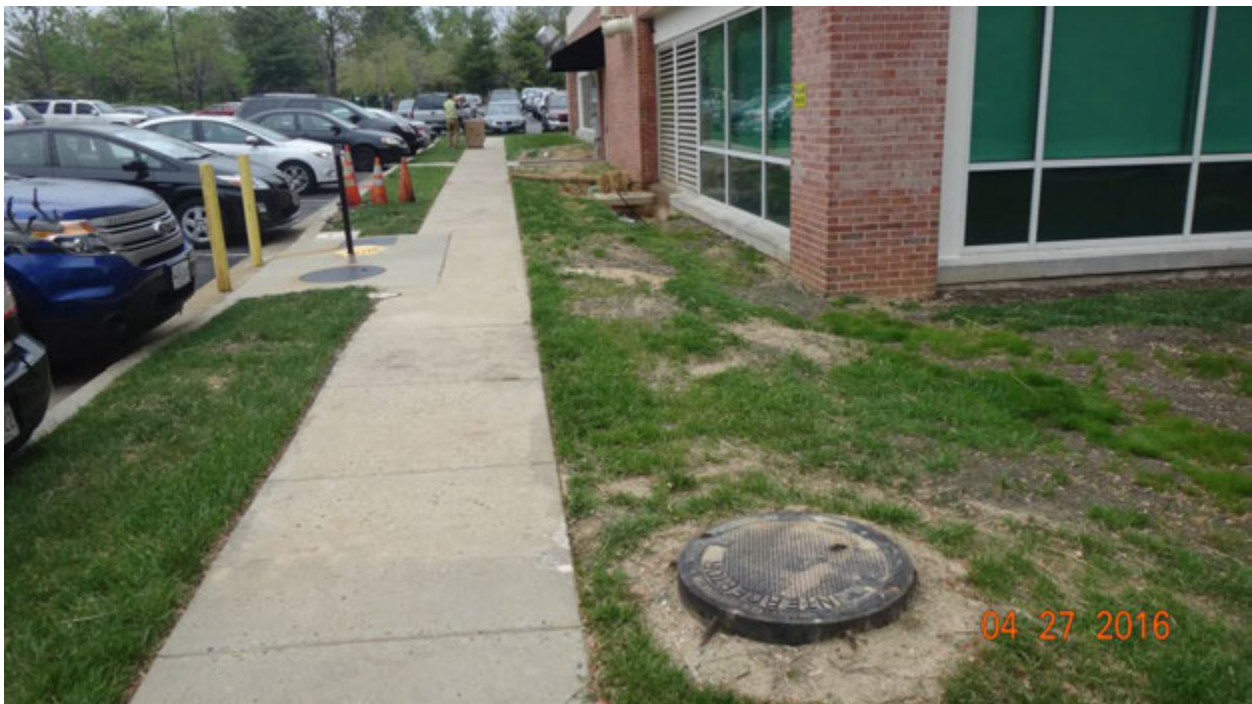
Figure 4. View showing the relative location of the yellow sign, on the near corner of the building, and the hole with the exposed lines (upper center, under the windows)
