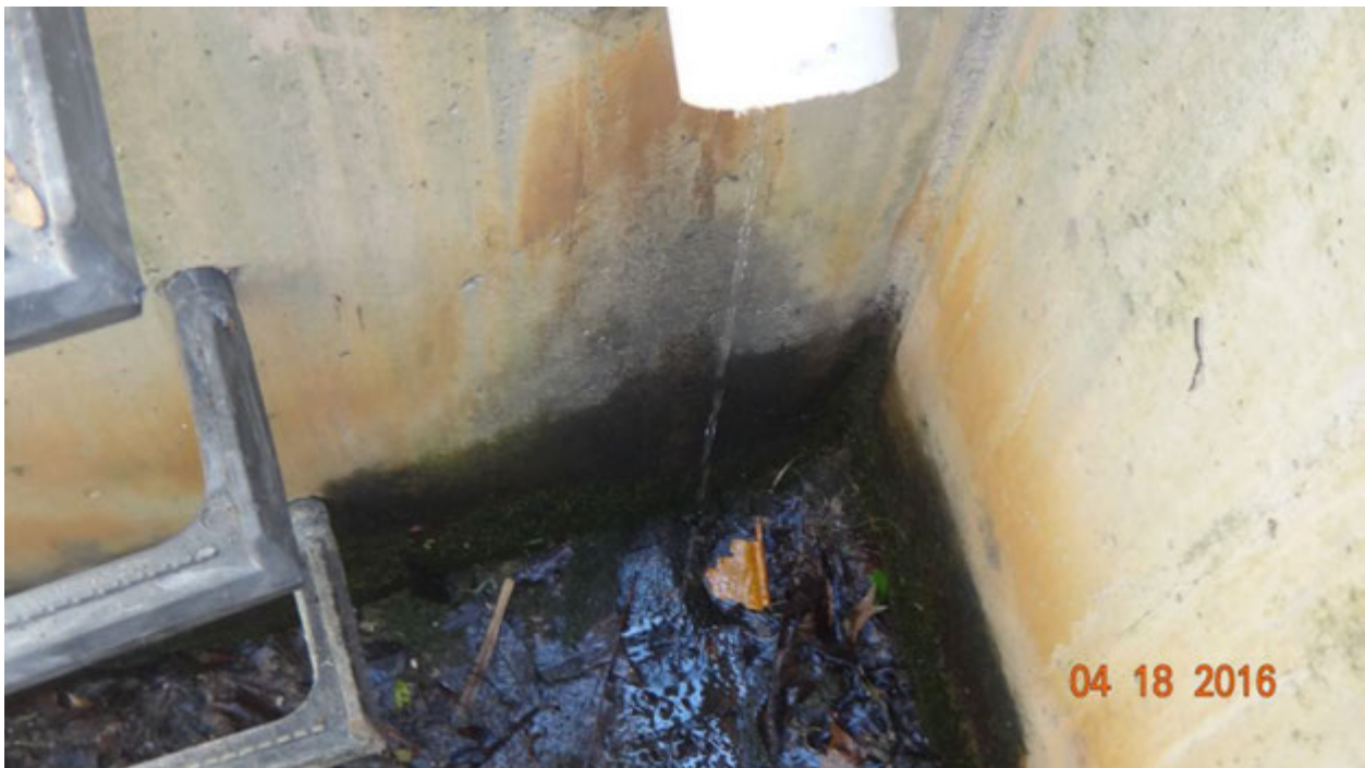
Figure 3. Trickleing effluent from the PVC pipe observed on April 18
