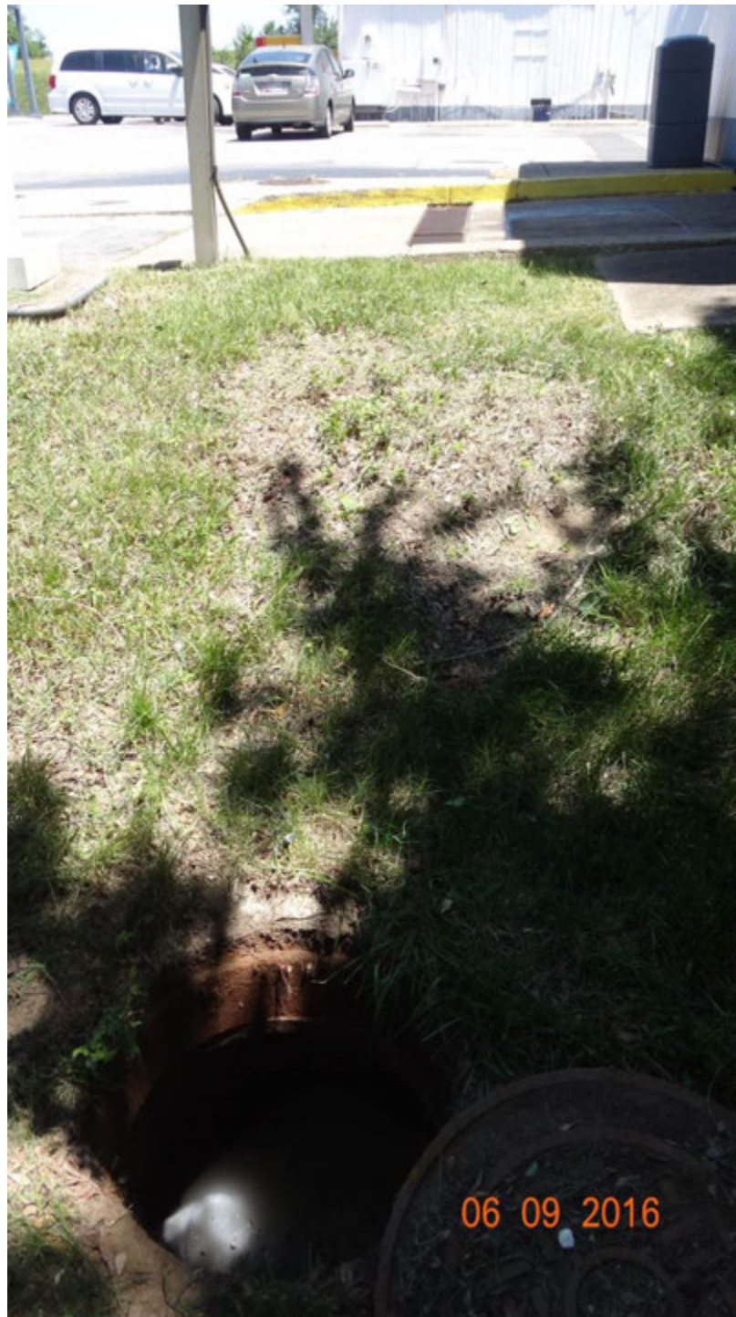
Figure 6. The relative location of the third manhole (lower left) to the exit for the car wash (top right, just outside of the view)
