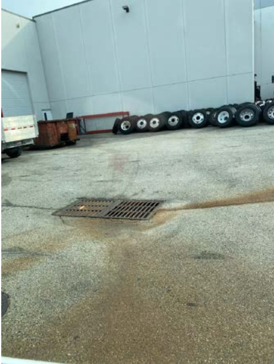
3/1/2022 Inspection – Location of storm drain inlet.
