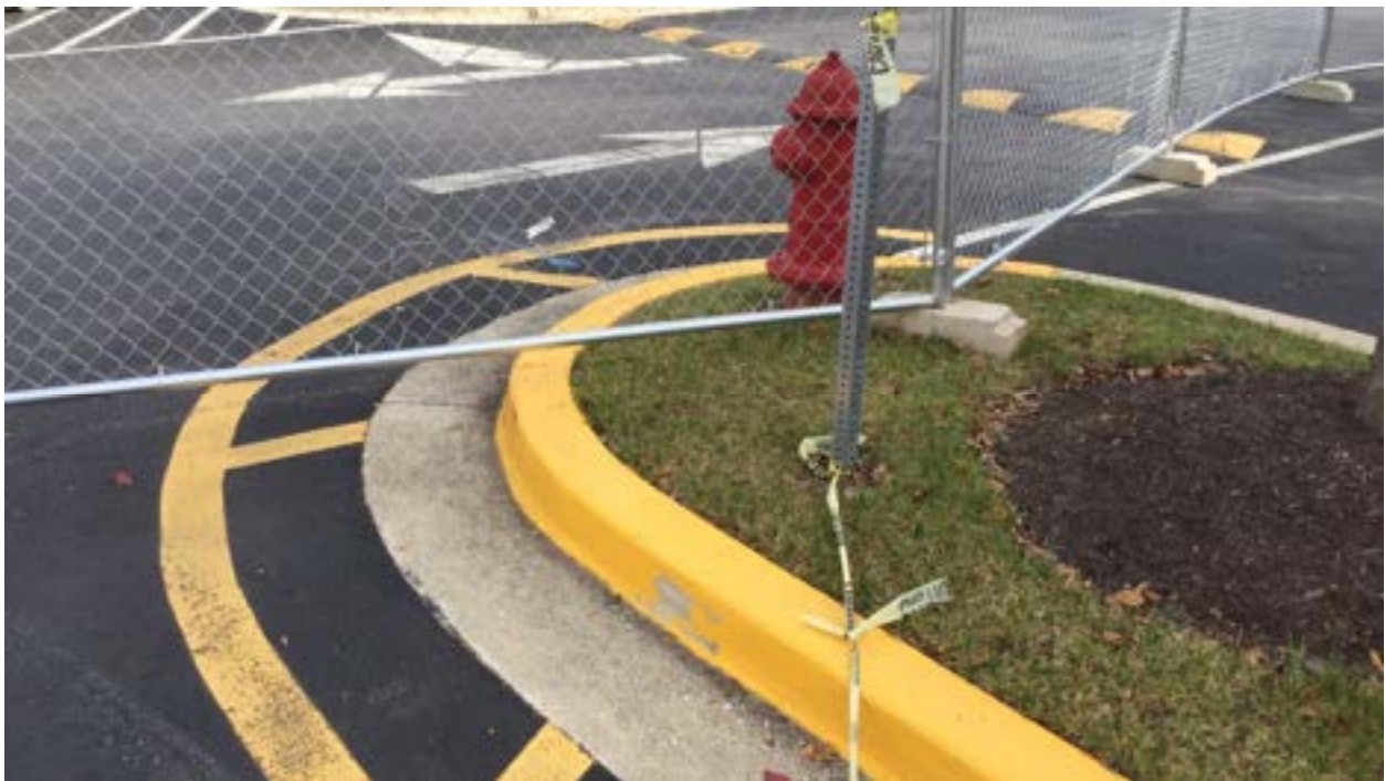
11/11/2021 Follow-Up Inspection – Fire hydrant no longer leaking.
