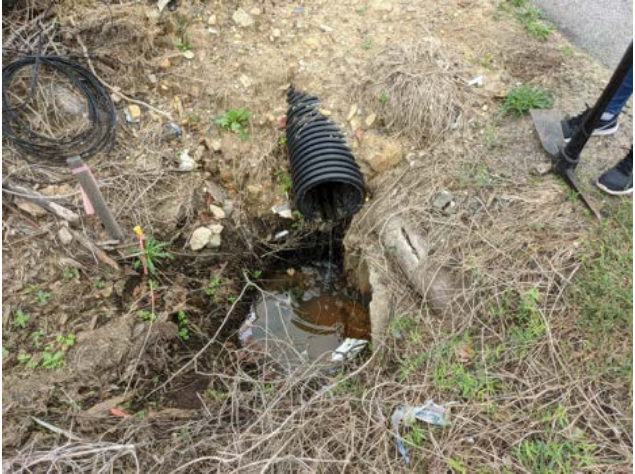
10/13/2021 Inspection – HDPE pipe where sample was taken. Upstream from outfall K02O001.
