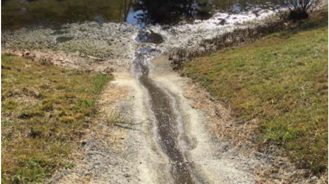
11/10/2021 Inspection – Downstream of outfall G06O006, showing visible flow.
