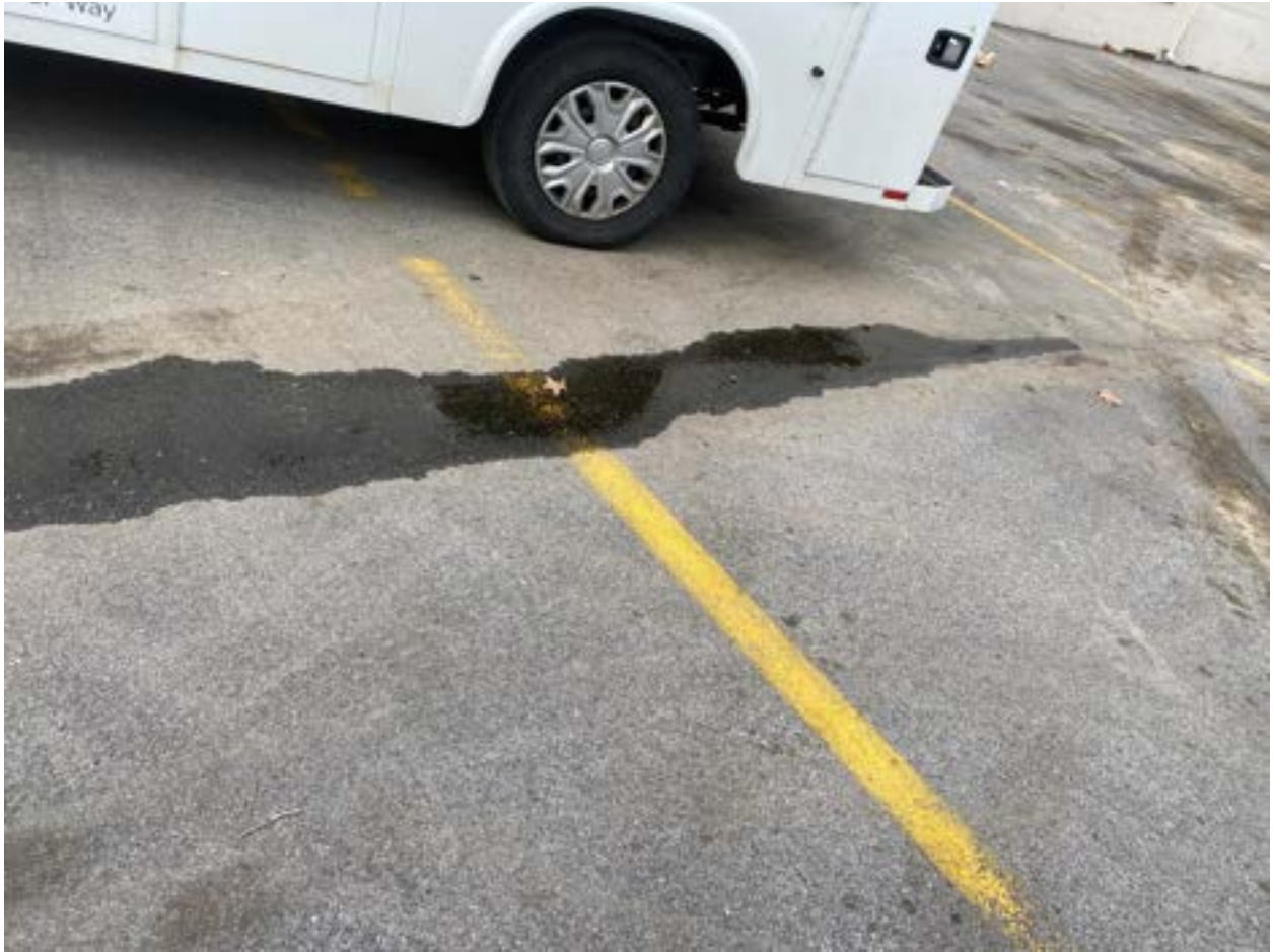
3/1/2022 Inspection – Oil flowing in the direction of a storm drain
