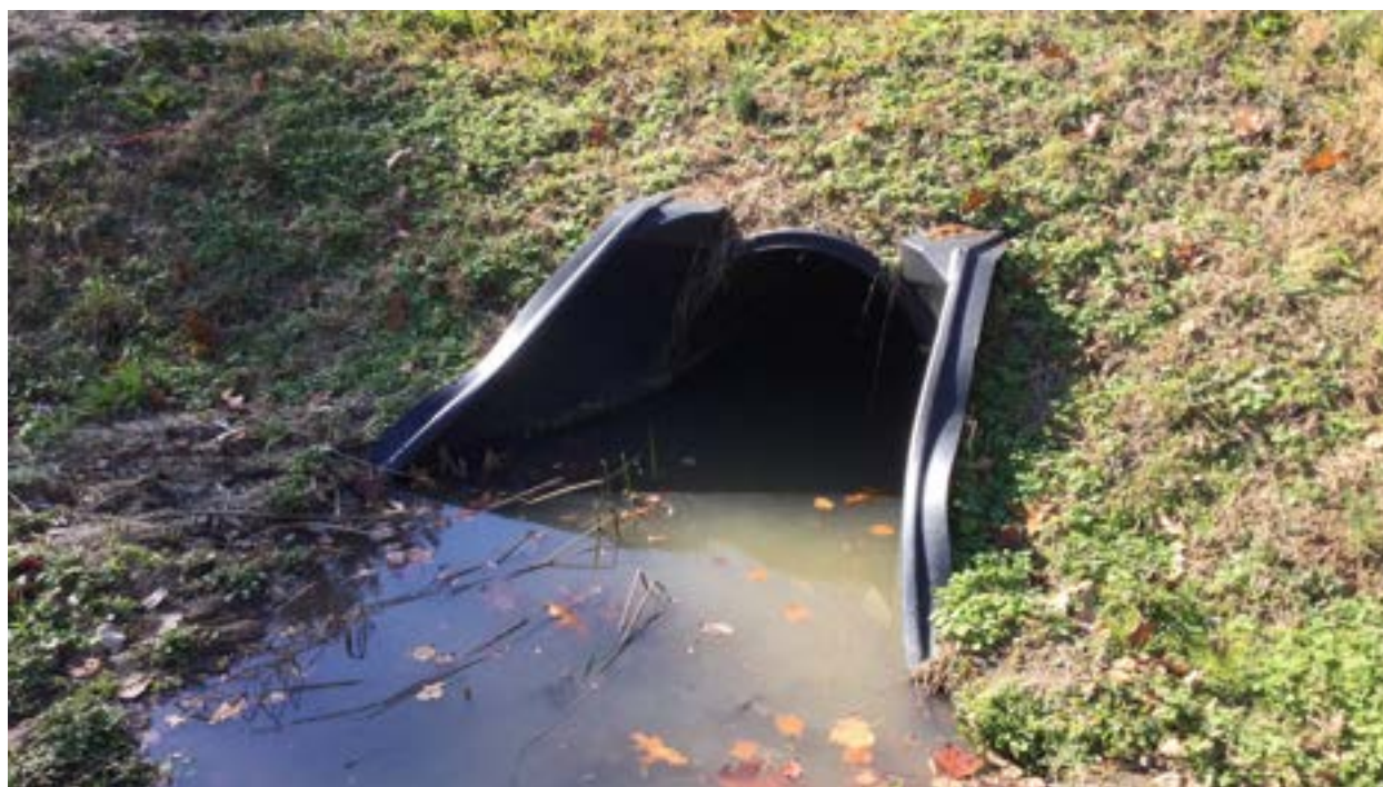
11/18/2021 Inspection – Overview of outfall J07O019.
