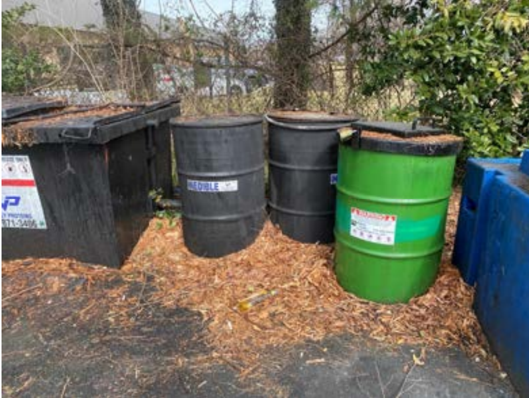
3/1/2022 Inspection – Location of uncovered kitchen grease drums.
