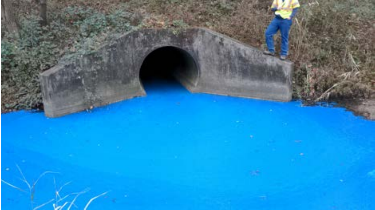
12/2/2021 Inspection – Overview of outfall J03O006.
