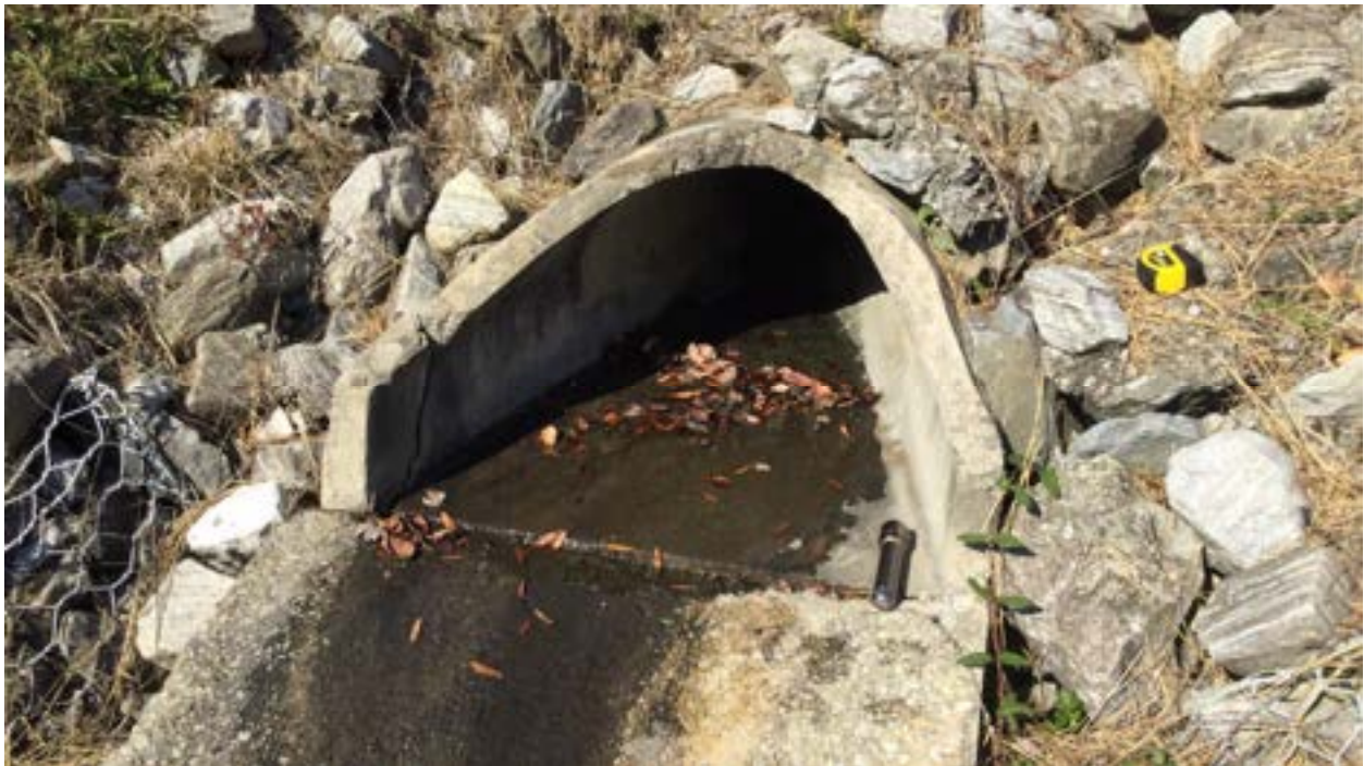
11/10/2021 Inspection – Overview of outfall G06O006.
