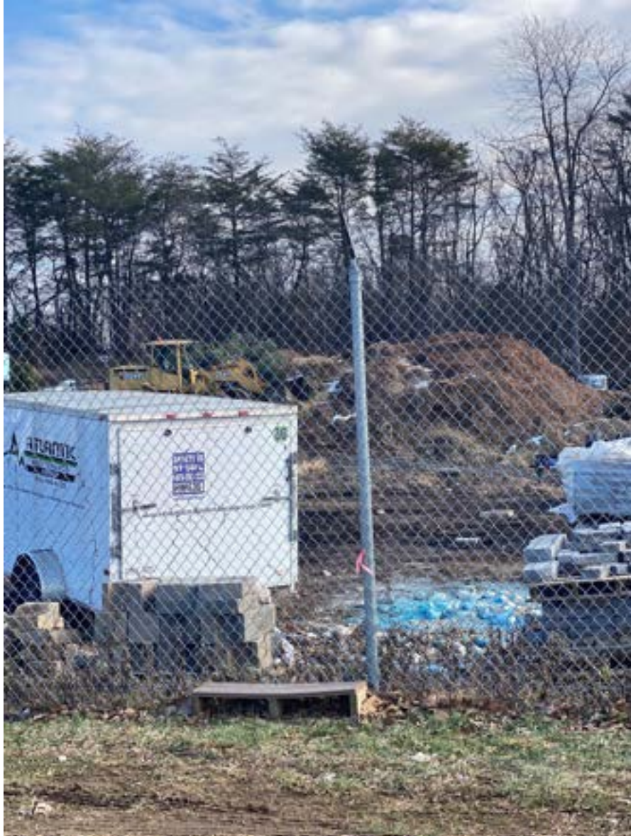
01/14/2022 Inspection – Location of blue deposit.
