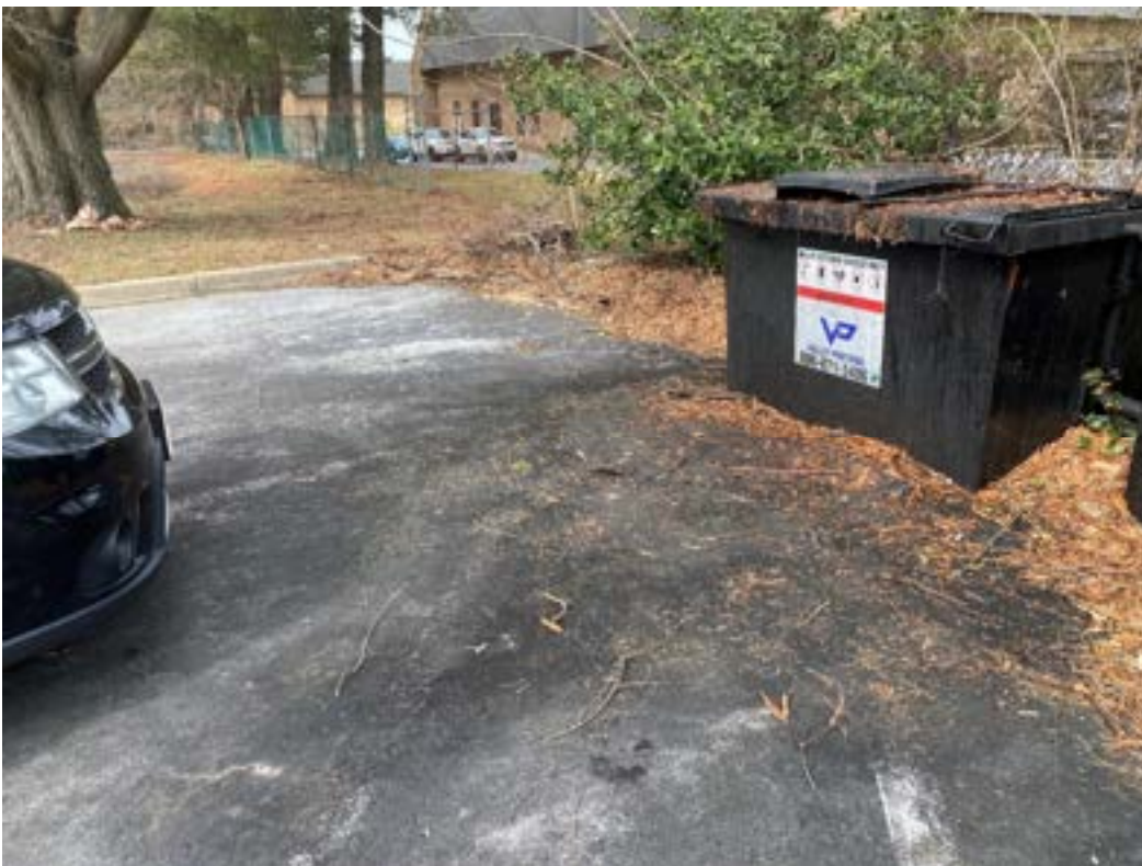
3/1/2022 Inspection – Location of stains in the vicinity of the kitchen grease barrel.
