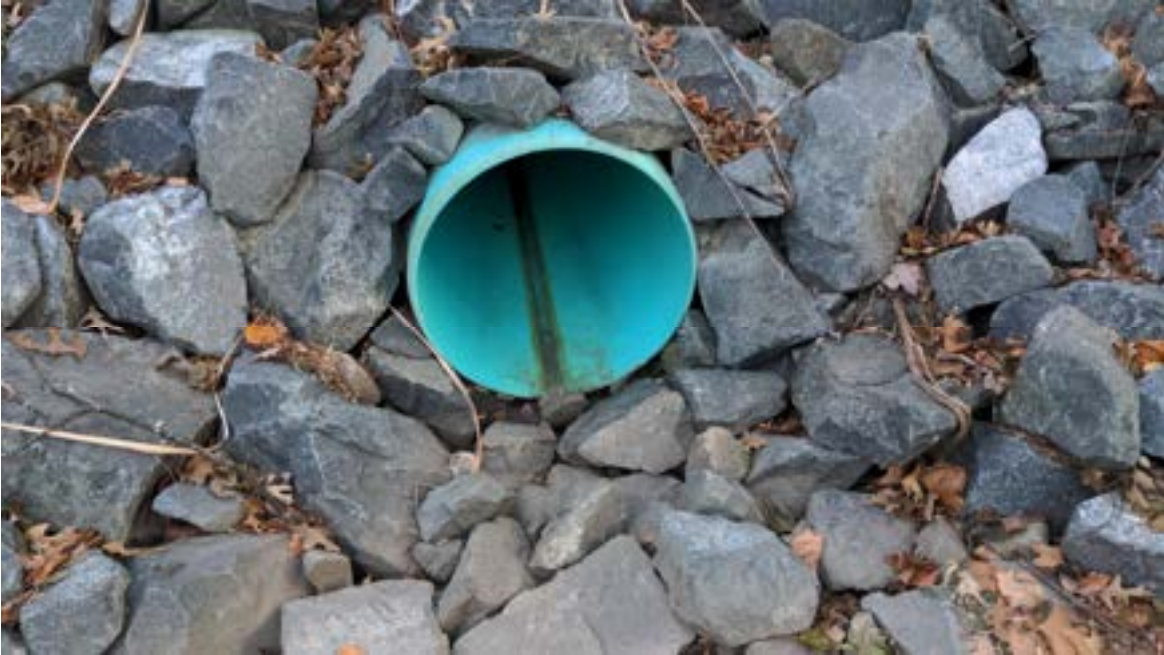
Inspection 12/16/2021 – Overview of outfall J040024.
