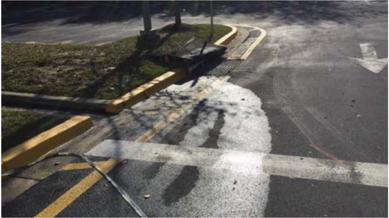
11/10/2021 Inspection – Leaking fire hydrant into storm drain.
