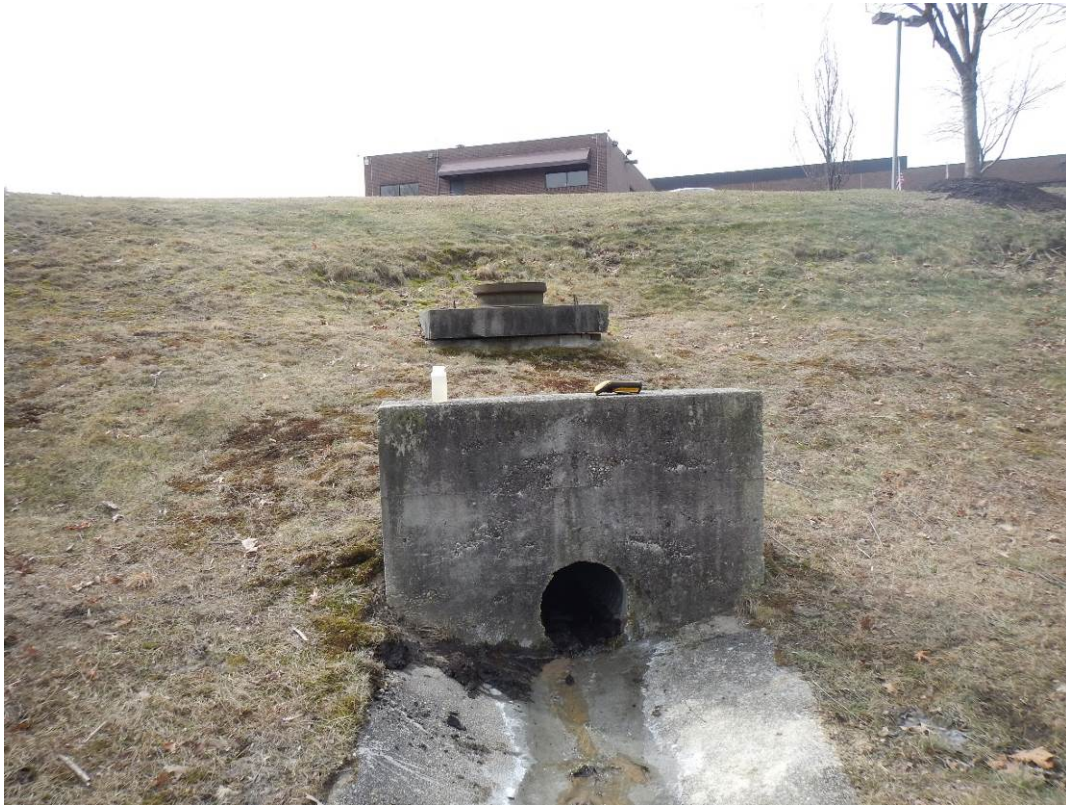
Figure 1. Outfall L07A1O004 at 1000 Stewart Ave.
