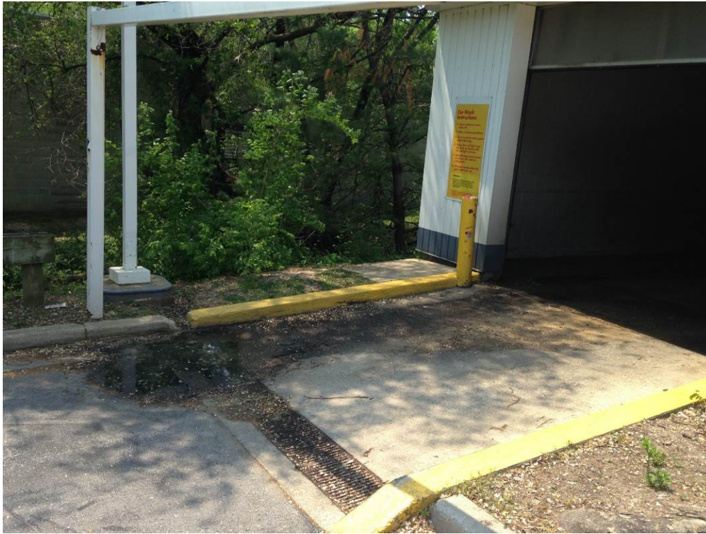
Figure 6. Trench drain at entry to Shell car wash
