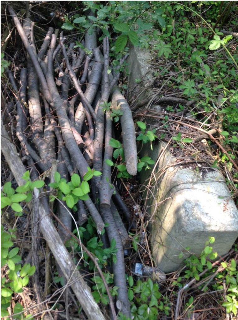
Figure 5. Outfall F09G5O001 with branches placed in front of orifice.
