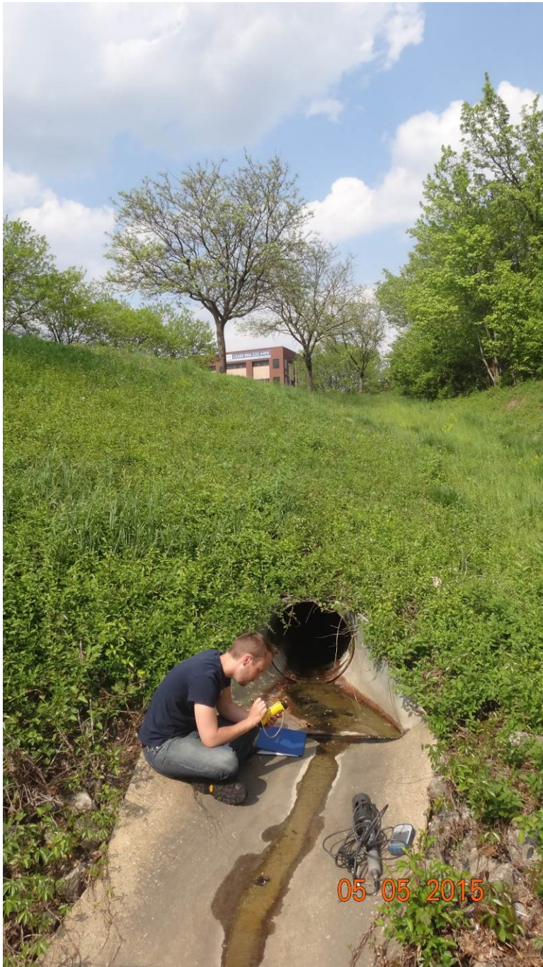
Figure 2. Outfall I04F3O014 discharging to dry pond
