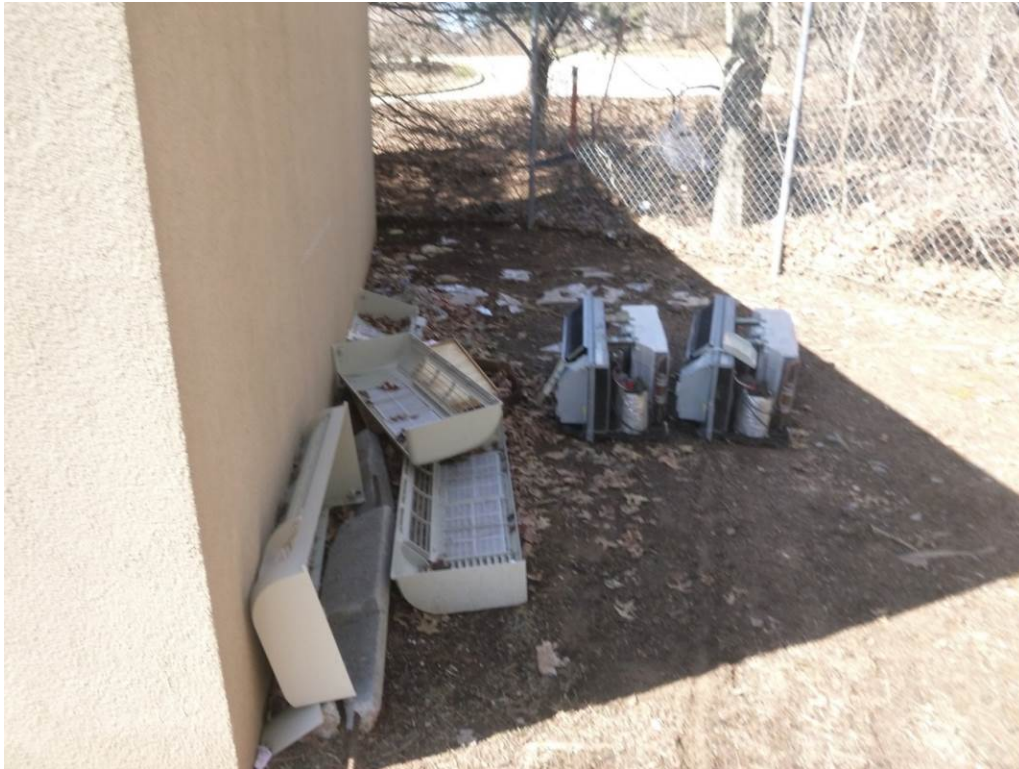
Figure 5. Several ventilation units and associated parts found on the ground near the dumpster
