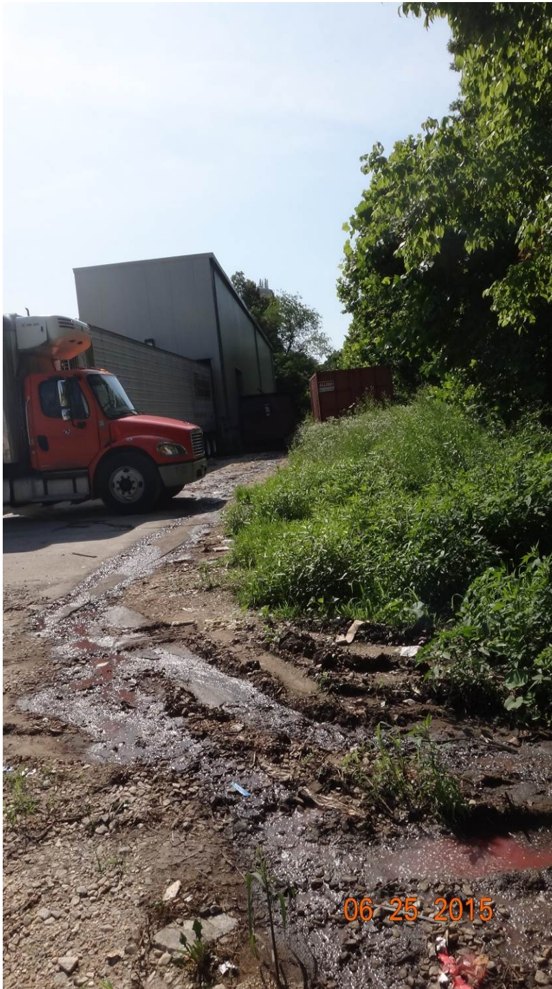
Figure 4. Red liquid leachate leading into the woods from the parking lot, as observed on June 25, 2015
