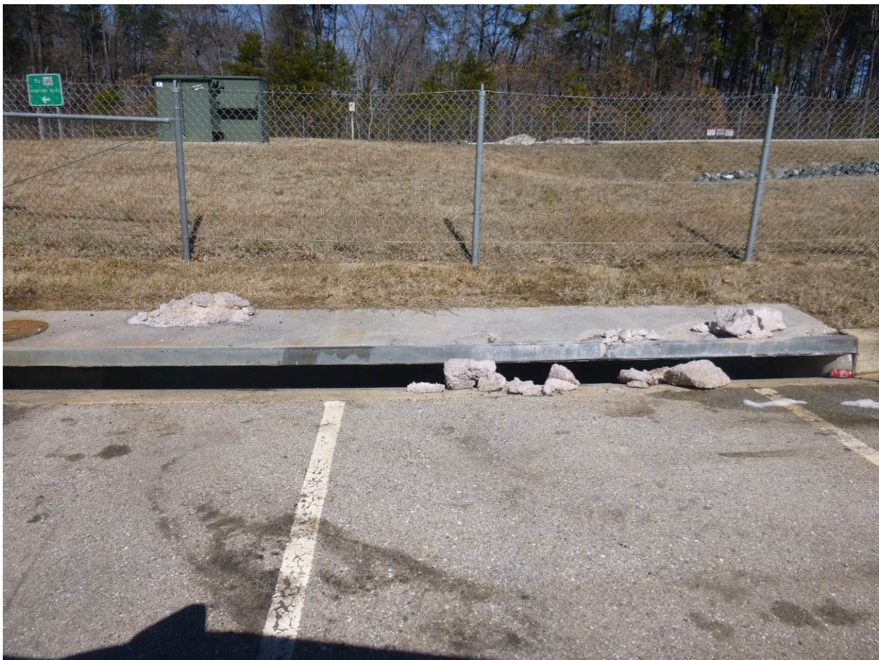
Figure 1. Road salt found at a curb inlet in a parking area associated with BWI Freight
