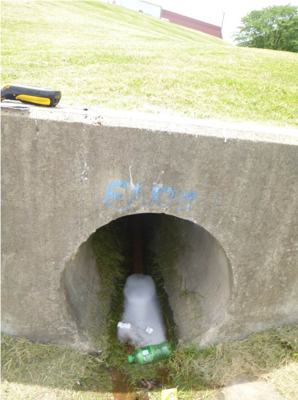
Figure 1. Outfall K02B8O002 with suds, May 28, 2015
