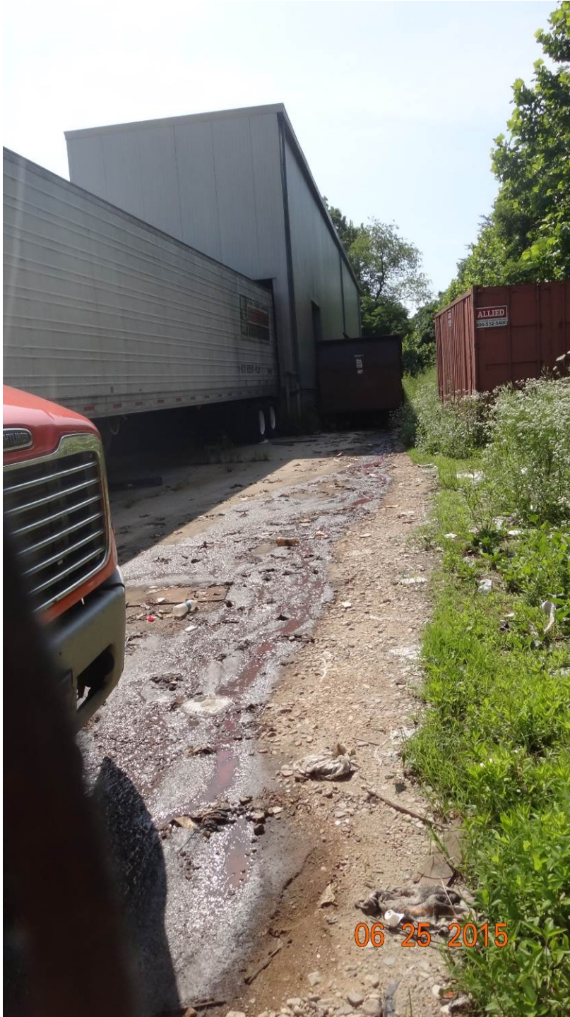
Figure 3. Fresh leachate trail as observed facing the dumpster on June 25, 2015
