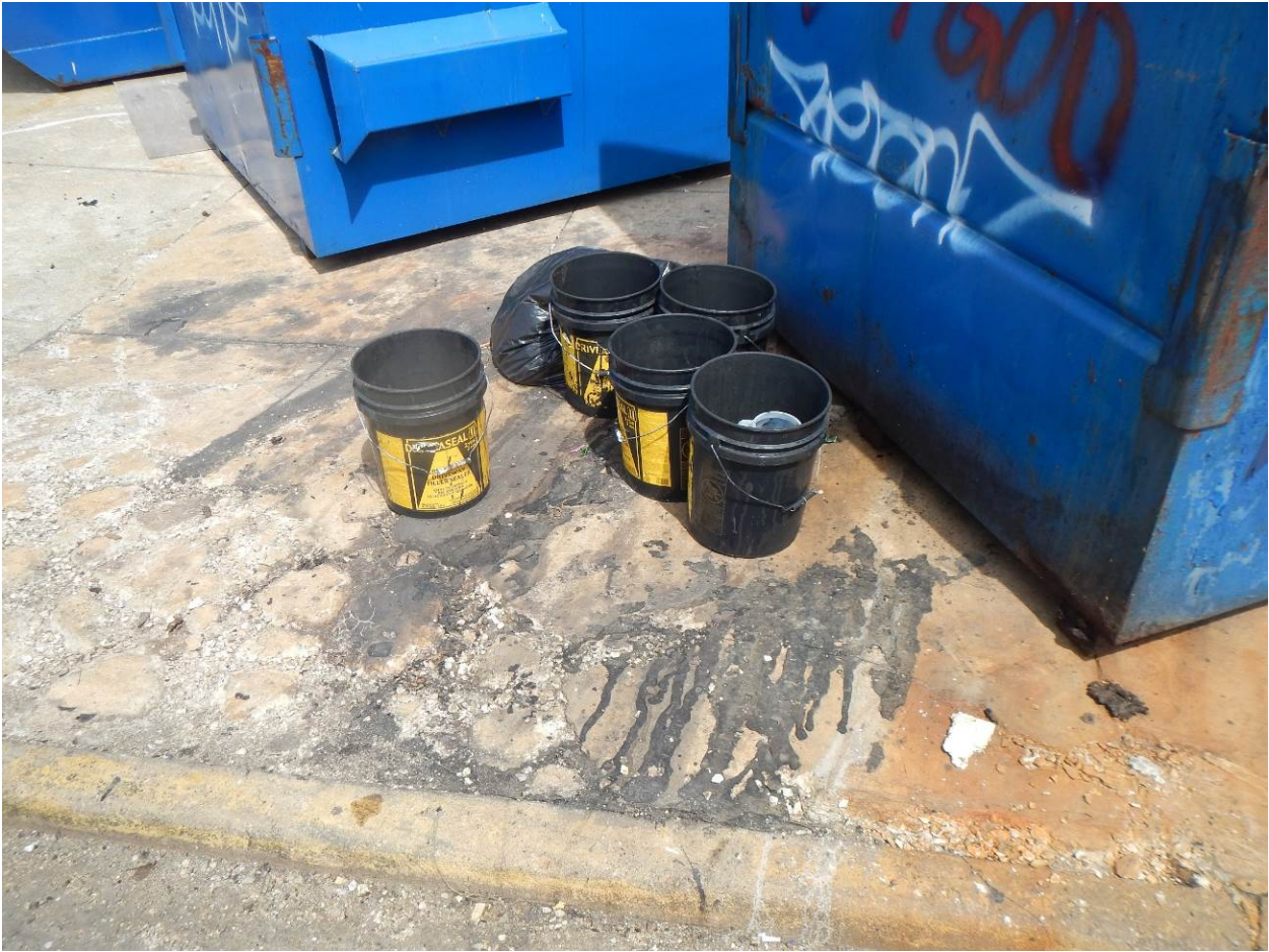
Figure 2. Extensive staining on the sidewalk near the open buckets of sealer
