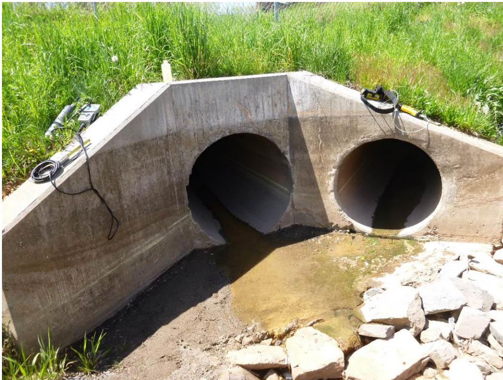
Figure 1. Outfalls F07F8O003 and F07F8O003NEW near Arbor Grove Drive
